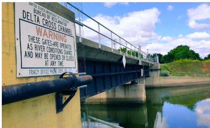
Two radial gates, each 60 x 30 feet and weighing a total of 243 tons, open to allow water to flow down the channel, or close to prevent drawing endangered fish species into the interior Delta.
