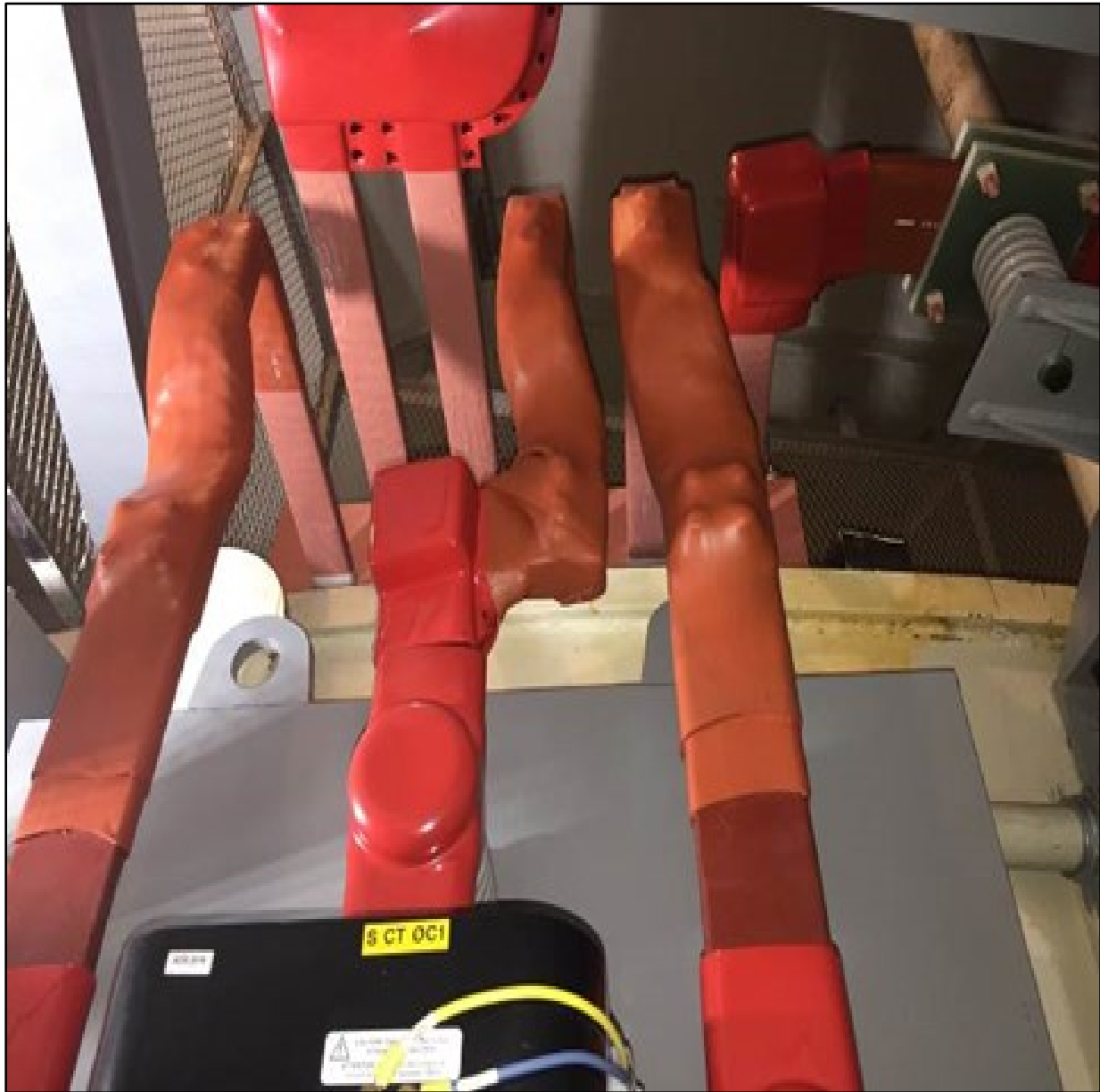
Phase B, single bar on with insulating boots and with shrink tube.
