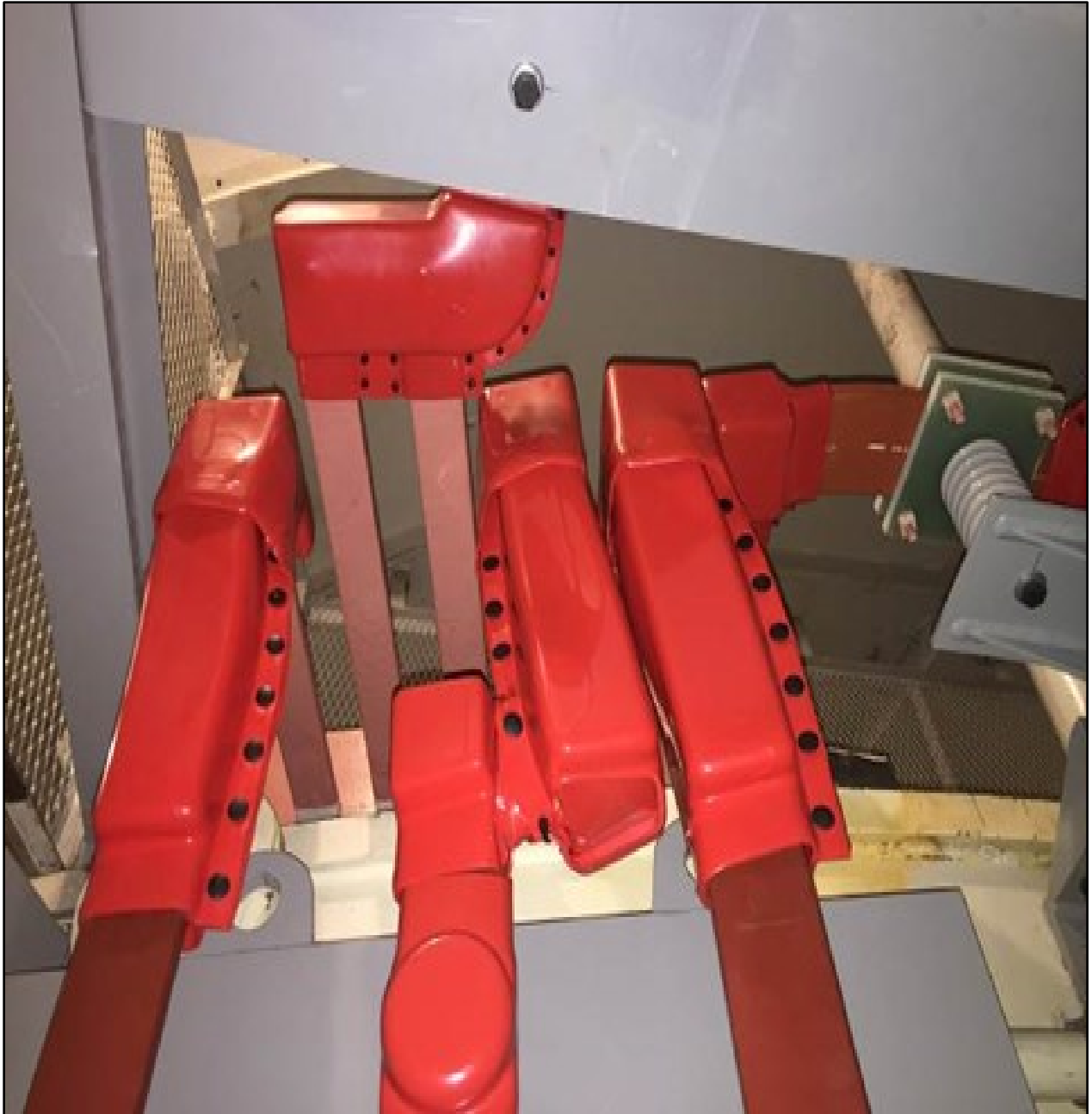
Looking up at Phase C with insulating boots and with shrink tube.
