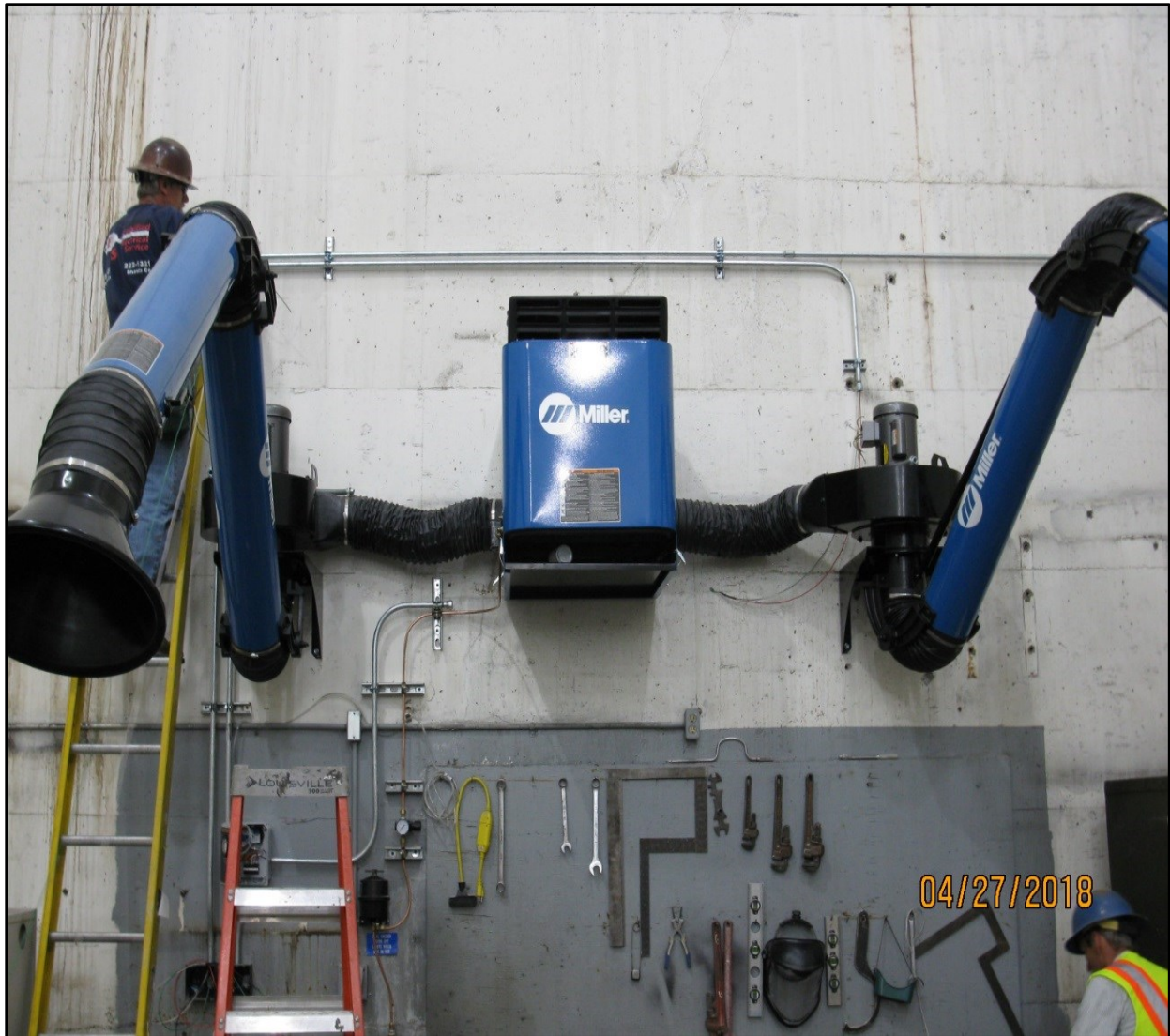
Keswick Powerplant: Installed welding shop ventilation system with two suction hoods and filtration cabinet
