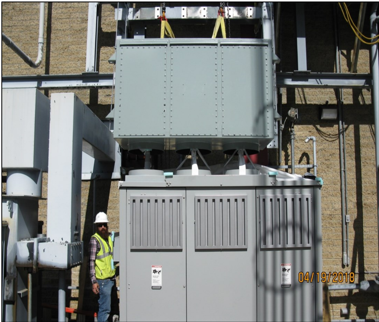
Transformer KRB set in place and the new CT compartment hung ready for connections
