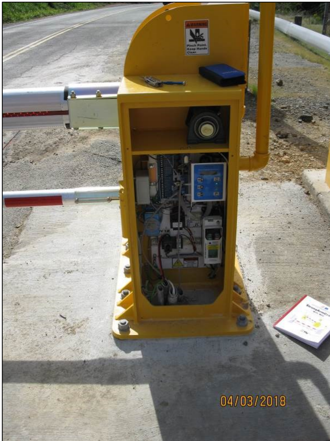
Shasta barrier control panel and junction box wiring inside the distribution box.
