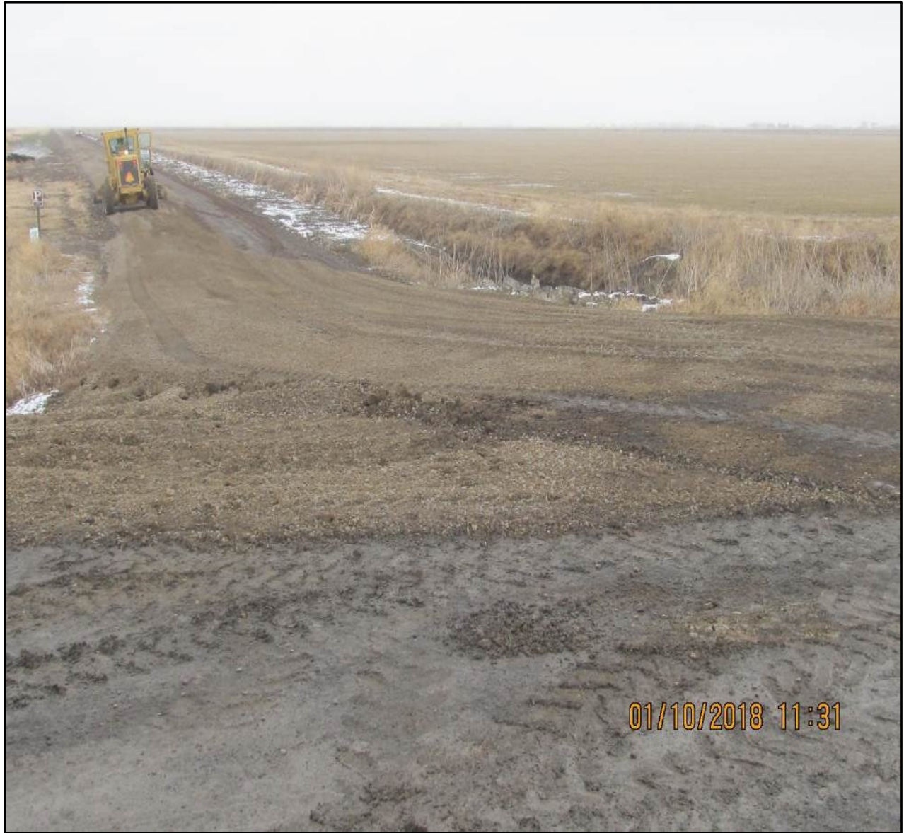
Tulelake Road Improvement Project, Phase 2 - Coleman Environmental Engineering Inc. Grader completing the last 6' wide section of the 20' wide East Road at the return onto "B" Dike Road.
