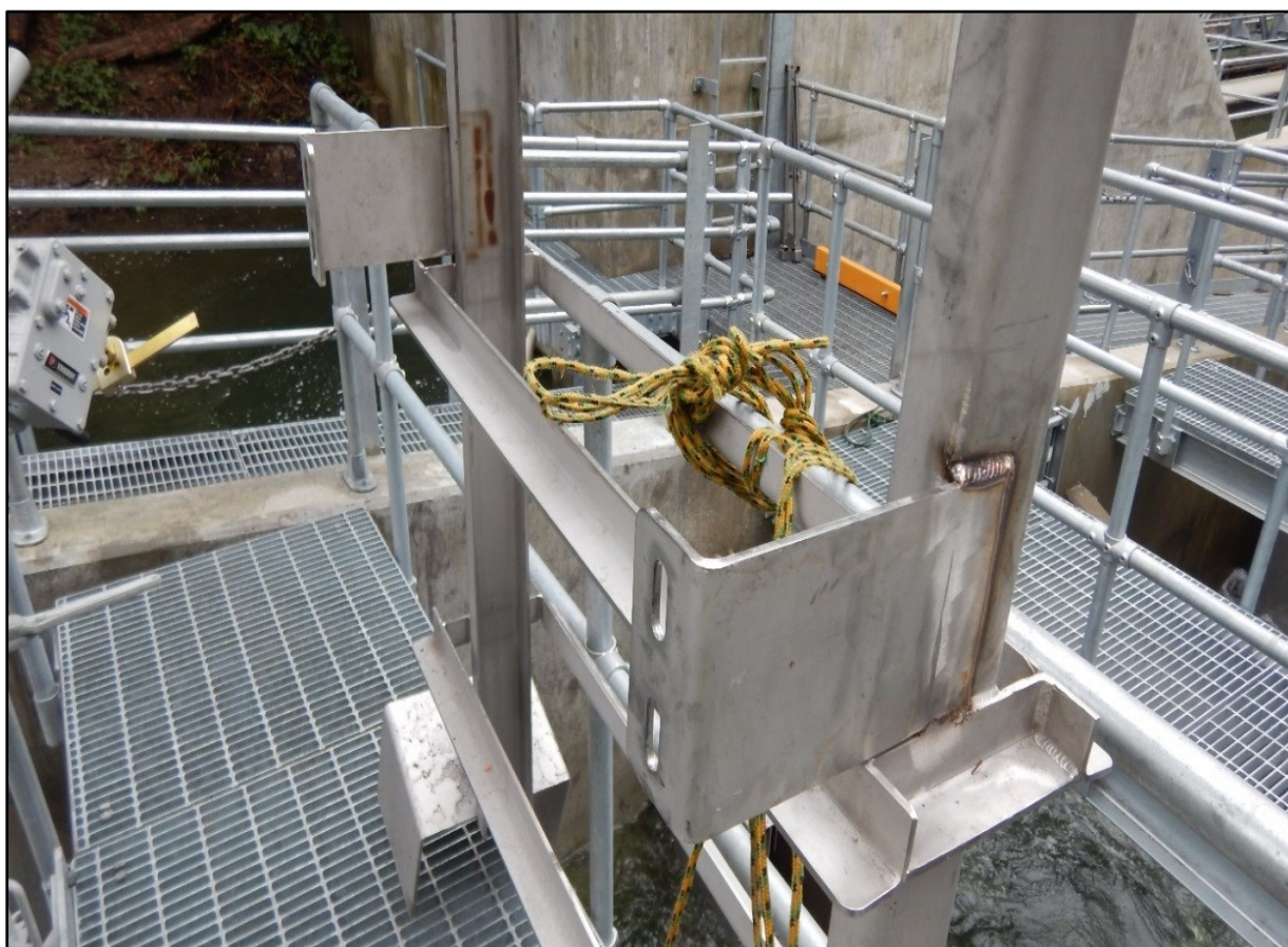
North Fork Screens and Ladders Completion Contract Modifications to the flash board guides at NBCFDD
