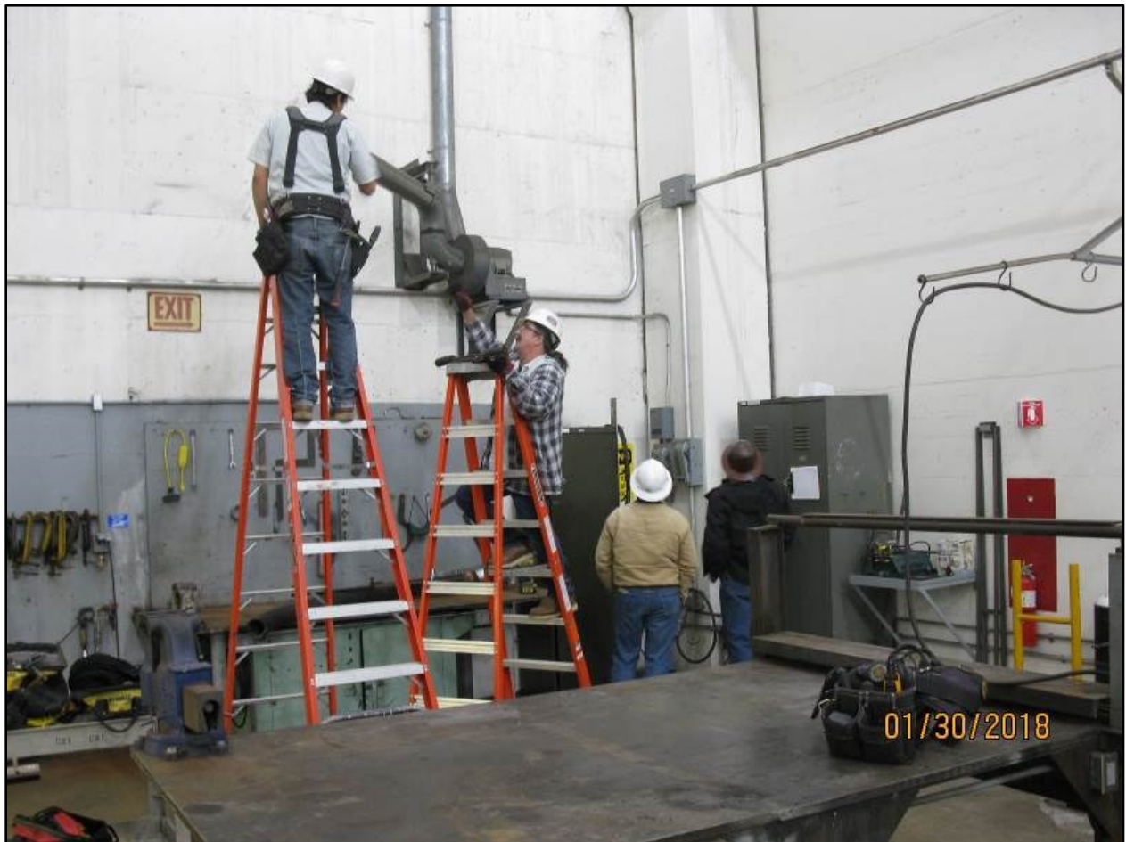
Keswick Powerplant Weldshop Removal of the existing ventilation system
