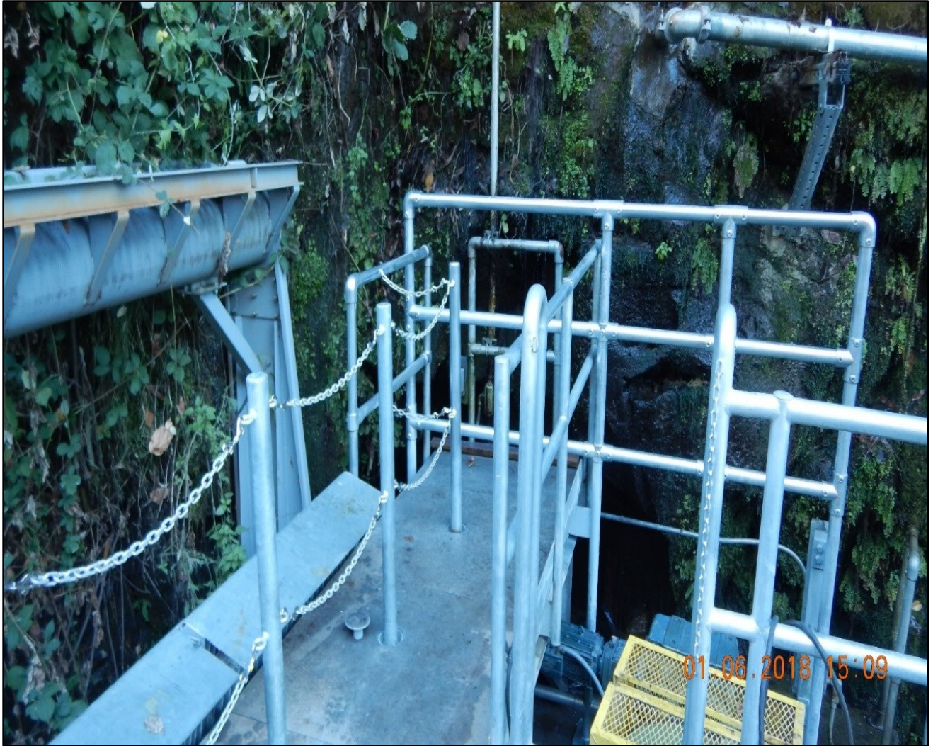
North Fork Screens and Ladders Completion Contract Installation of the ECDD removable guardrail
