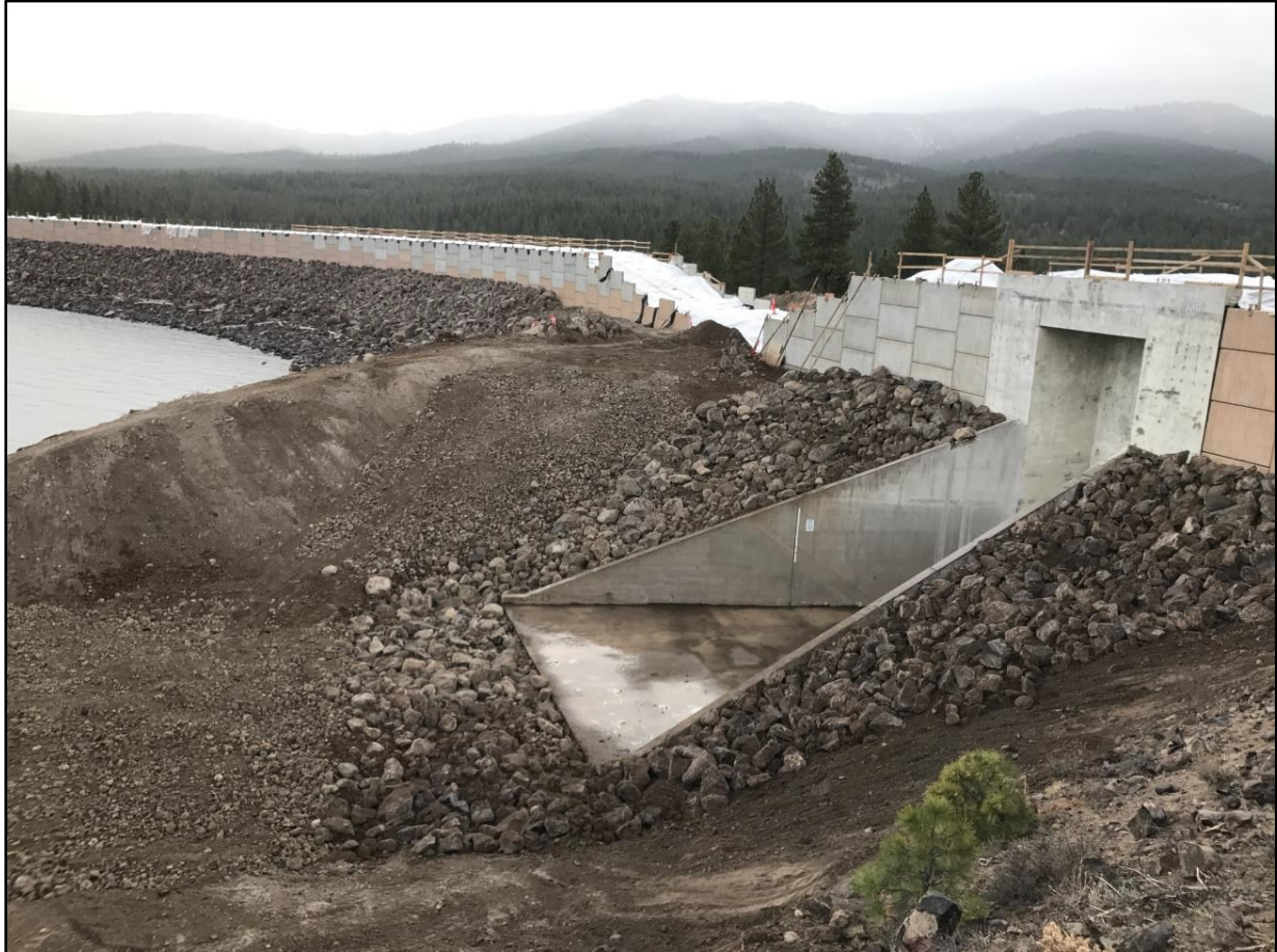
Stampede Dam, Dam Safety Modifications A view of the Stabilized Spillway Inlet Channel and Mechanically Stabilized Earth Paneling.
