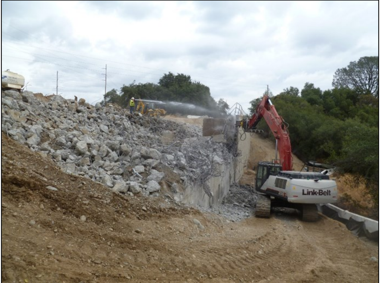
Folsom Aggregate Structure Demolition, Removal & Disposal The Excavator using the Hydraulic Hammer to Demolish the Concrete Aggregate Sorting Structure.
