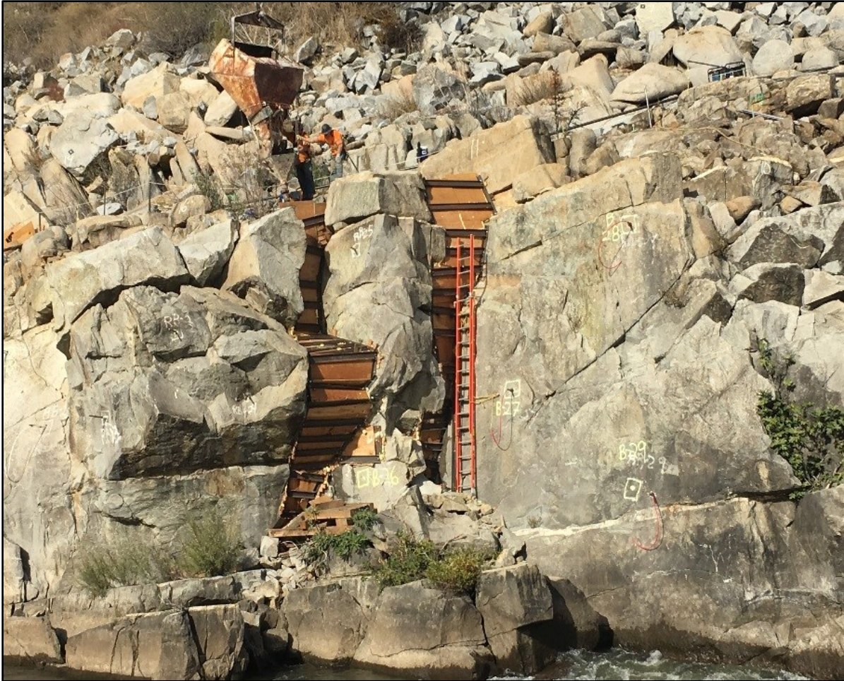
Folsom Dam Auxiliary Spillway American River Phase V – Right Bank Stabilization A View of the Dental Concrete Formwork at the entrants
