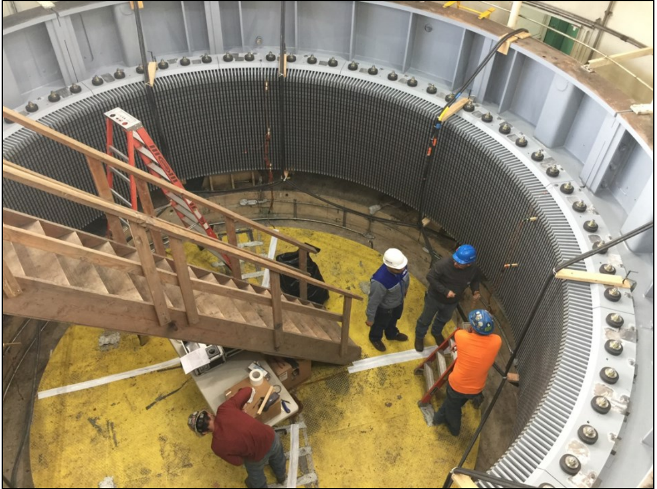
Trinity Powerplant Generator Rewinds A View of the Stator Core being Prepared for Testing.
