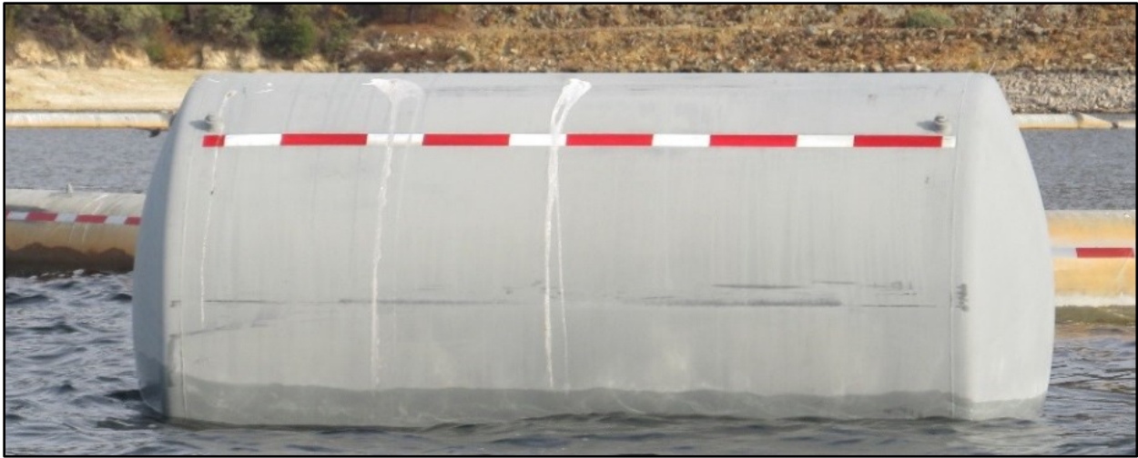
Whiskeytown Lake, Spring Creek Temperature Control Curtain An Image of Some of the New Reflective Tape after Being Installed.
