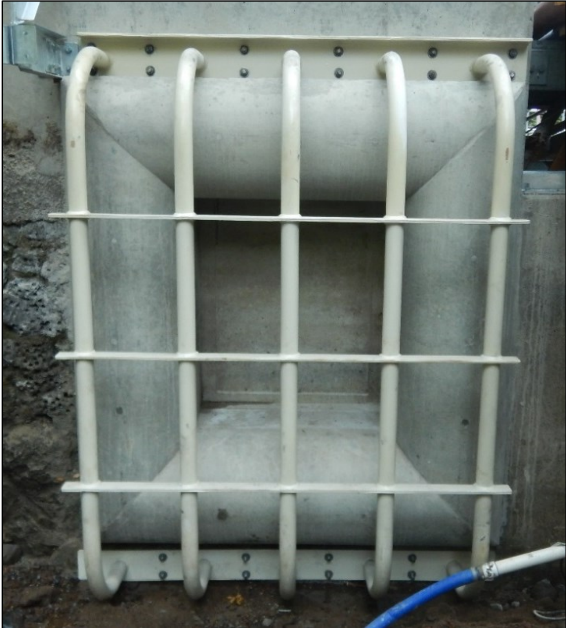
North Fork Screens and Ladder Completion Contract A View of the New Bullnose Trash rack on the North Battle Creek Feeder Diversion Dam.
