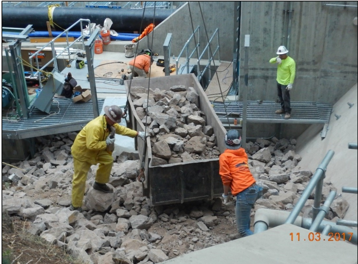
North Fork Screens and Ladder Completion Contract Riprap being Installed on the downstream left abutment.
