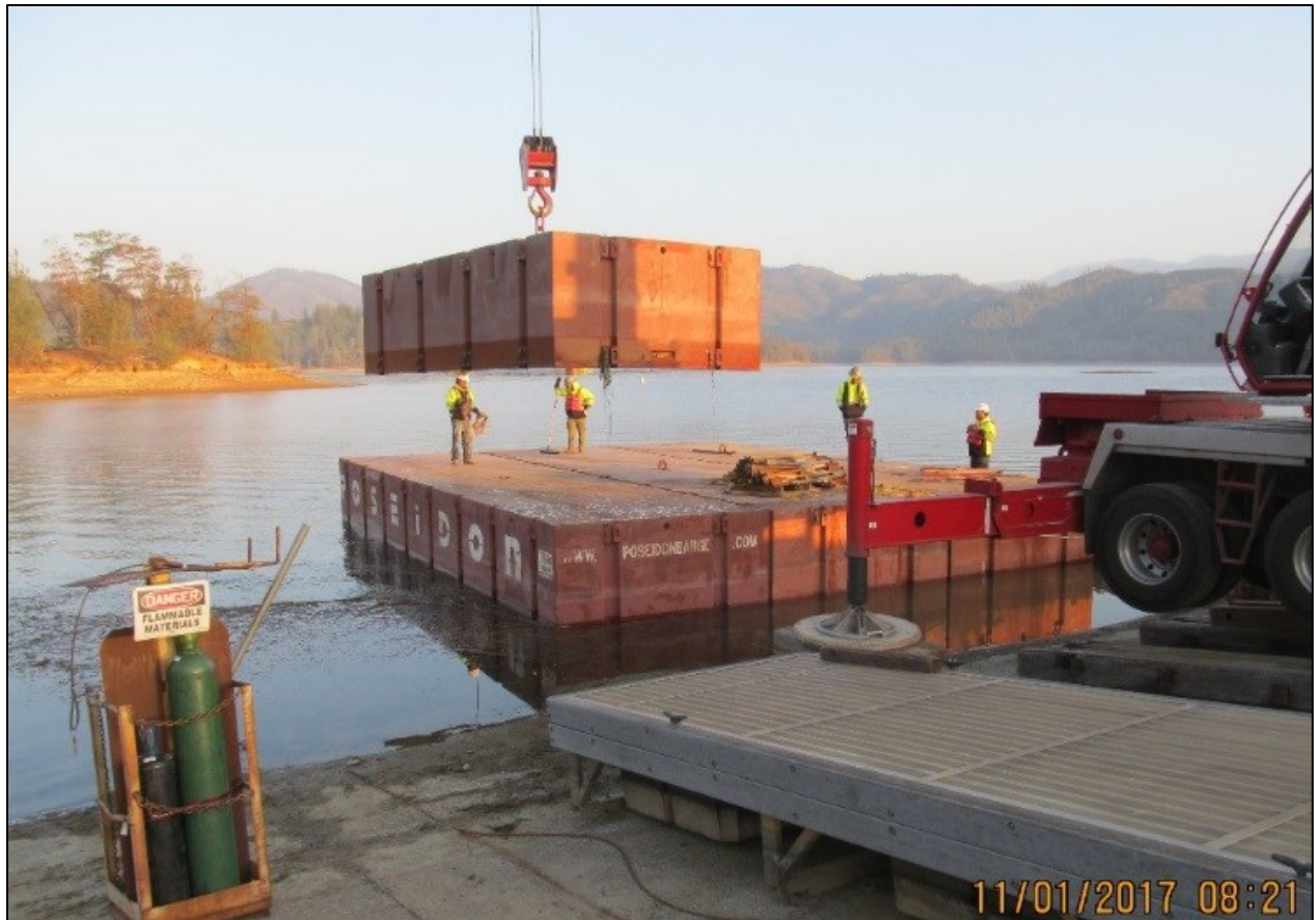
Whiskeytown Lake, Spring Creek Temperature Control Curtain A View of the Contractor Disassembling the Barge.
