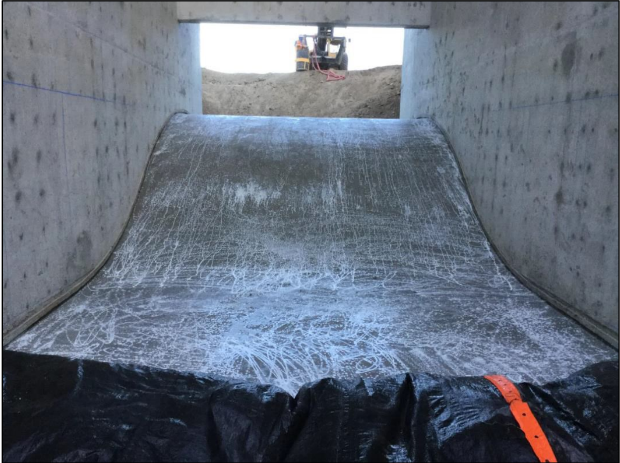
Stampede Dam, Dam Safety Modifications A view of the Ogee Crest
