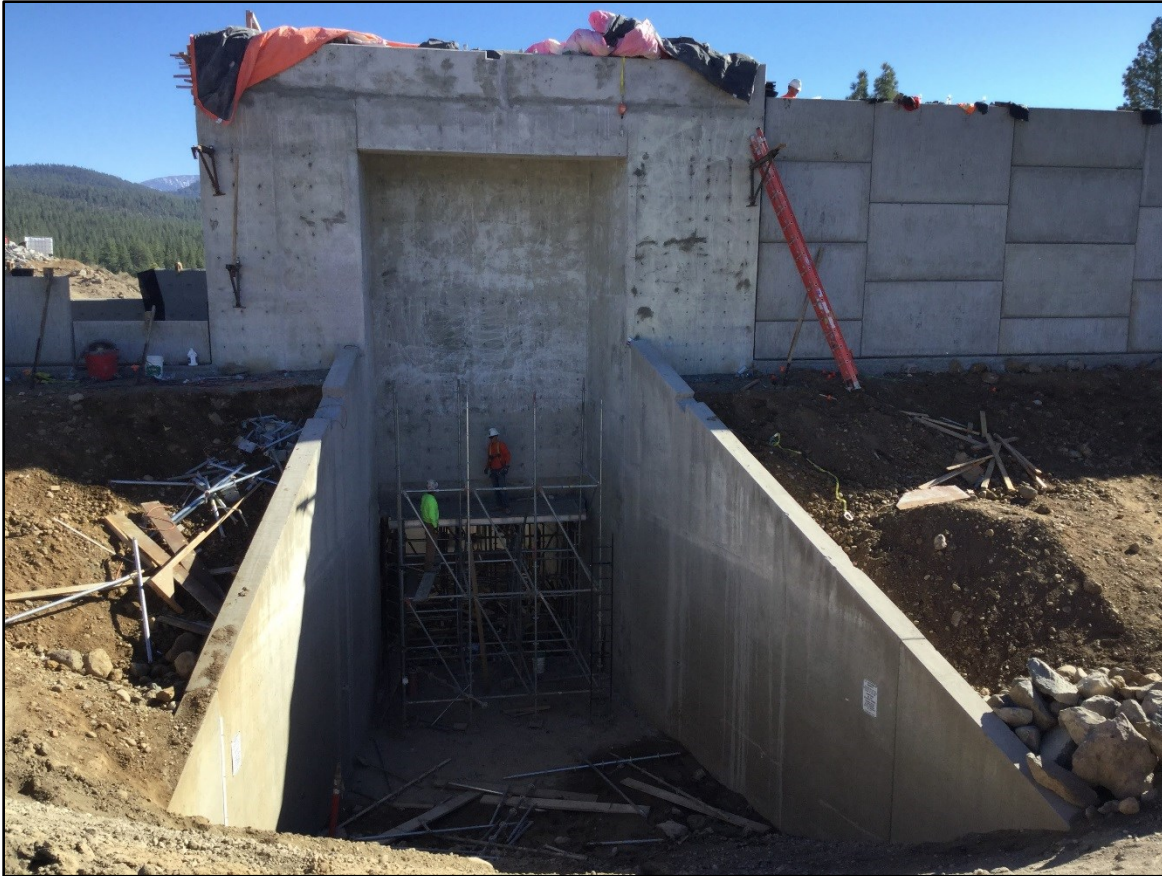
Stampede Dam, Dam Safety Modifications The new spillway bridge deck and headwall.
