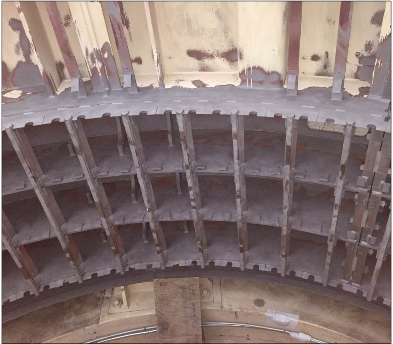
Trinity Powerplant Generator Rewinds A view of the stator frame after being abrasive blasted.
