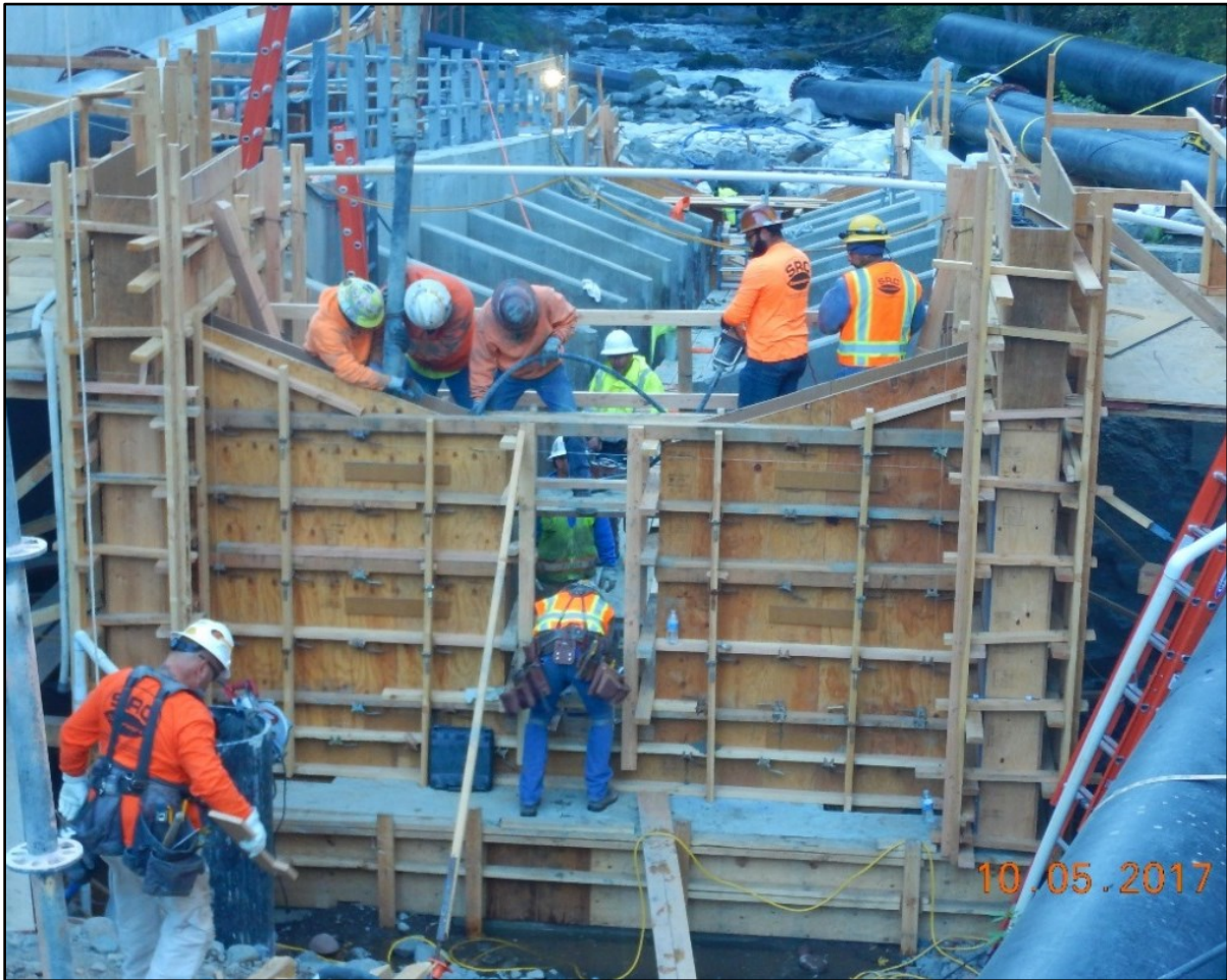
North Fork Screens and Ladder Completion Contract Concrete placement of the Fish Ladder Baffle A Walls.
