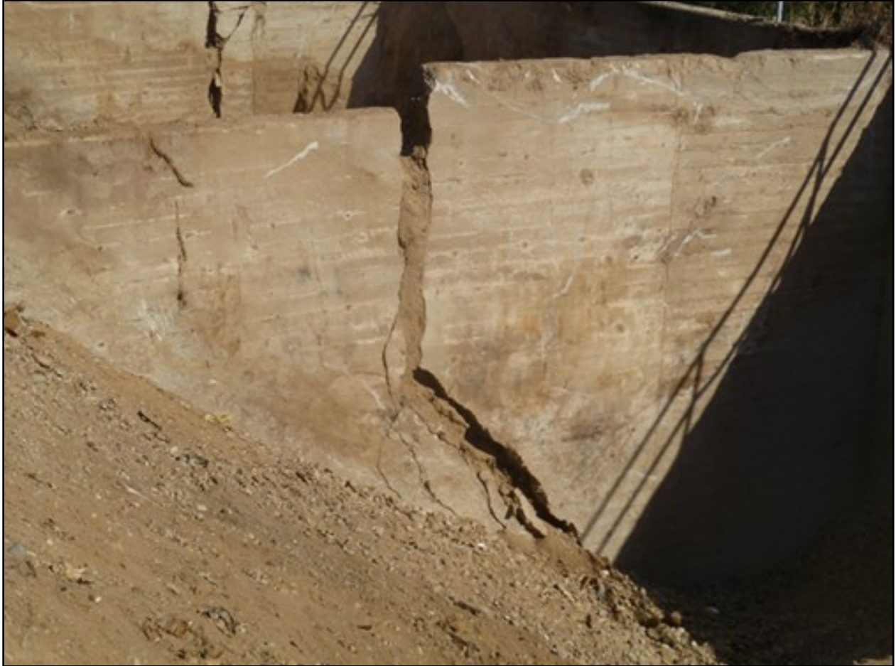
Folsom Aggregate Structure Demolition, Removal & Disposal A view of a significant failure along the interior wall of one of the aggregate structure sorting bins.
