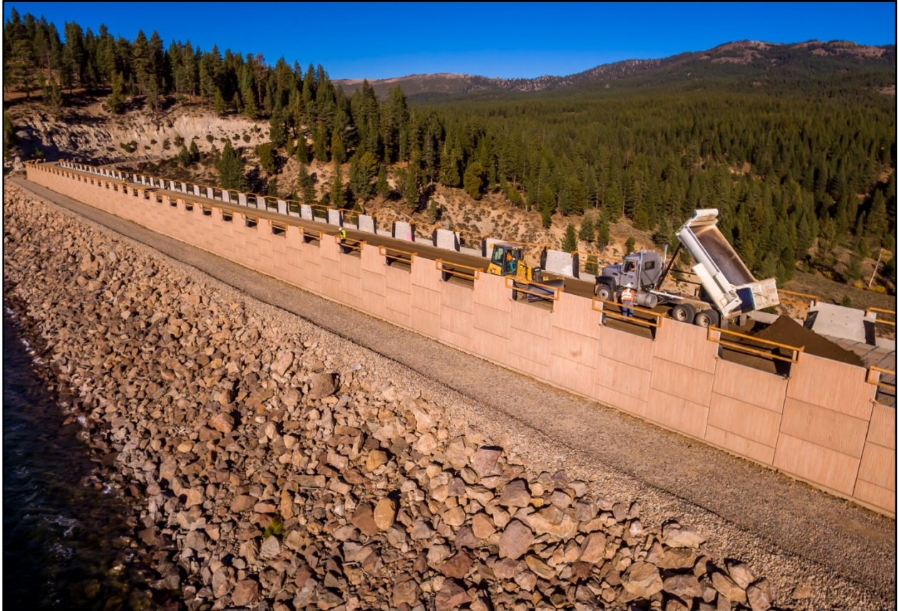
Stampede Dam, Dam Safety Modifications A view of the Mechanically Stabilized Earth wall being completed.
