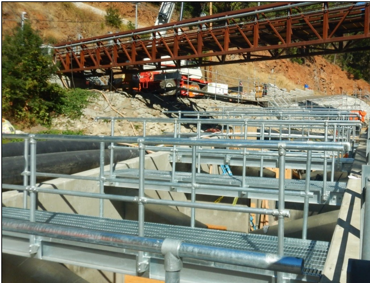
North Fork Screens and Ladder Completion Contract The new catwalks over the baffle bays.
