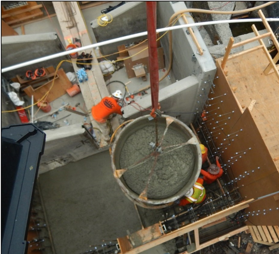
North Fork Screens and Ladder Completion Contract A view of the upstream slab being poured.
