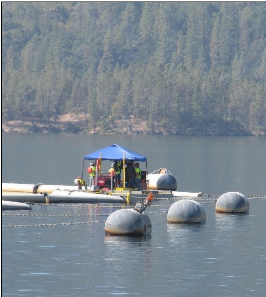
Whiskeytown Lake, Spring Creek Temperature Control Curtain The Contractor installing the foam injection nipples on the float tanks.
