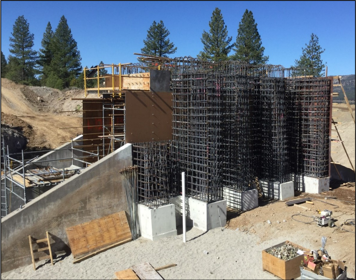
Stampede Dam, Dam Safety Modifications A view of the second wall lift at the spillway.
