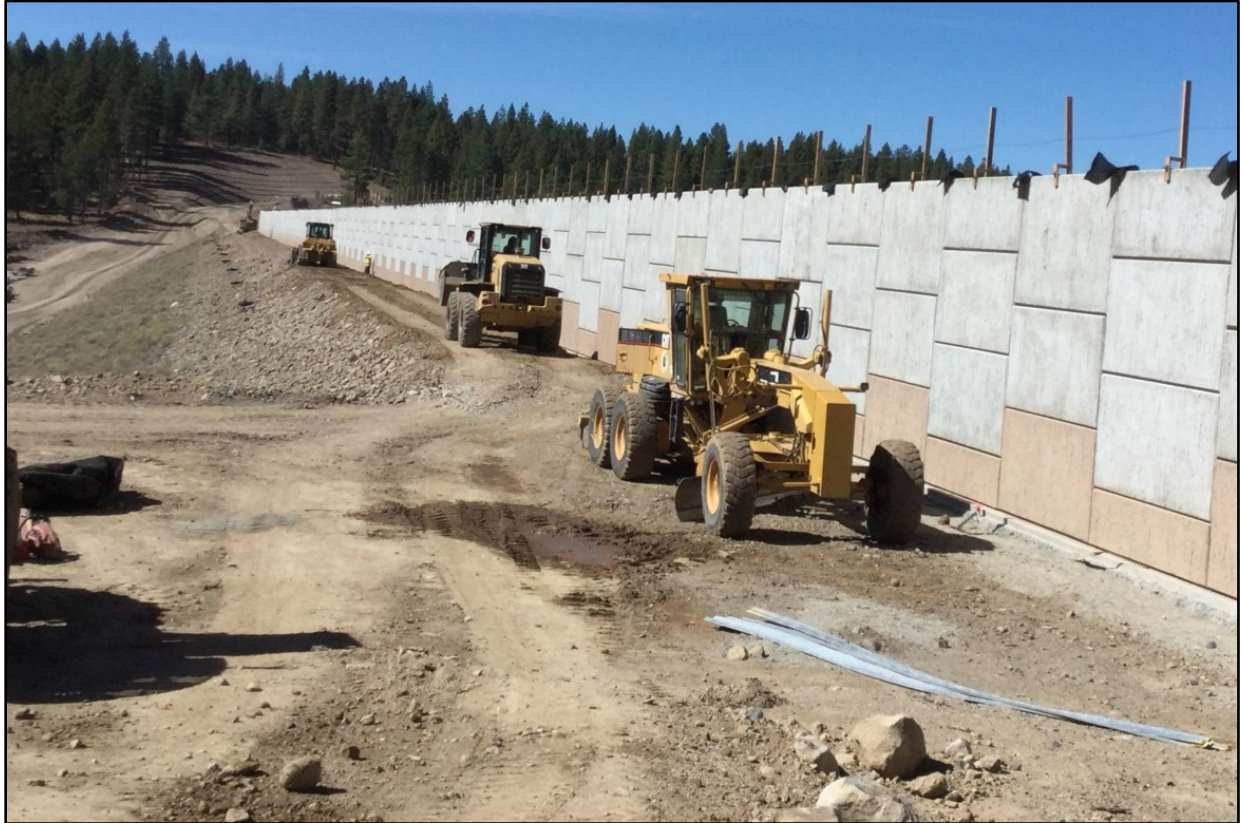
Stampede Dam, Dam Safety Modifications The O&M road being constructed.
