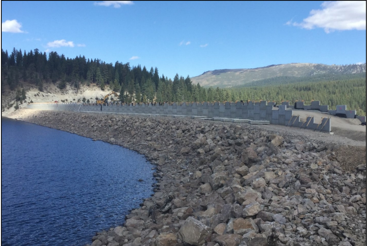
Stampede Dam, Dam Safety Modifications A view of the Fourth Course of MSE wall on the dam.
