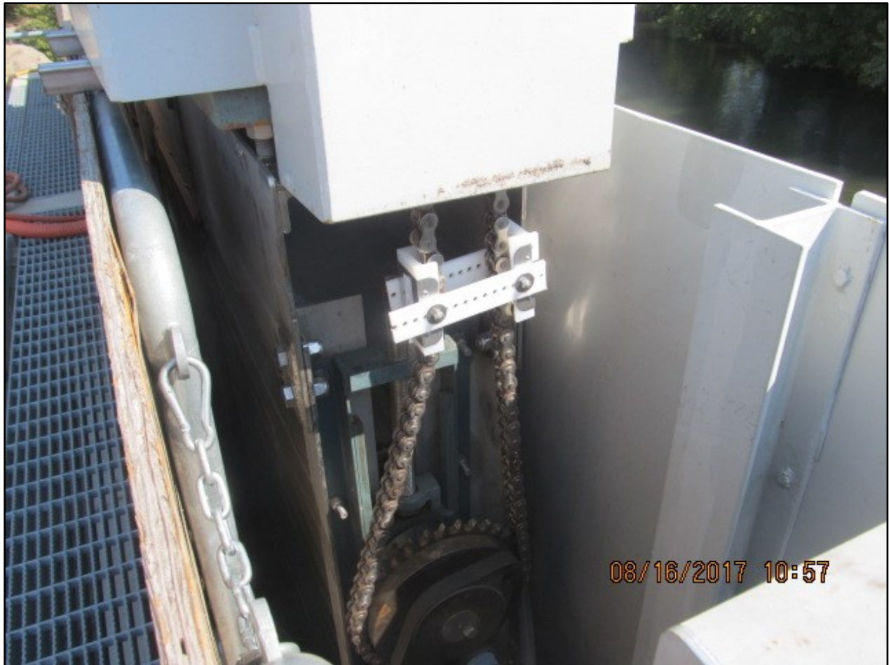
Intake 3 Screen Extension, Coleman National Fish Hatchery An image of the installed chain tensioner.
