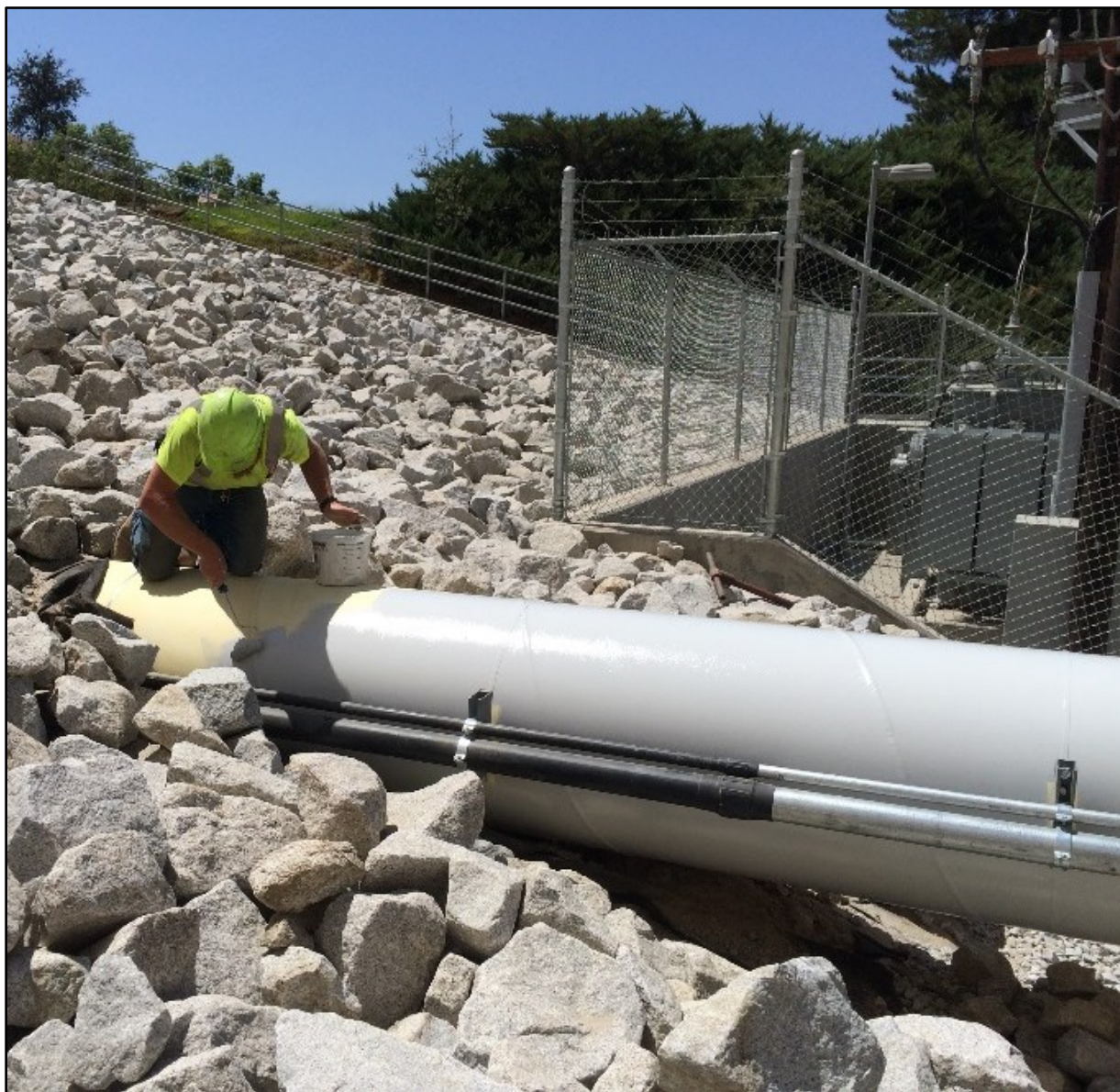
San Joaquin Hatchery Water Supply Pipeline A view of the pipe being coated by the contractor.
