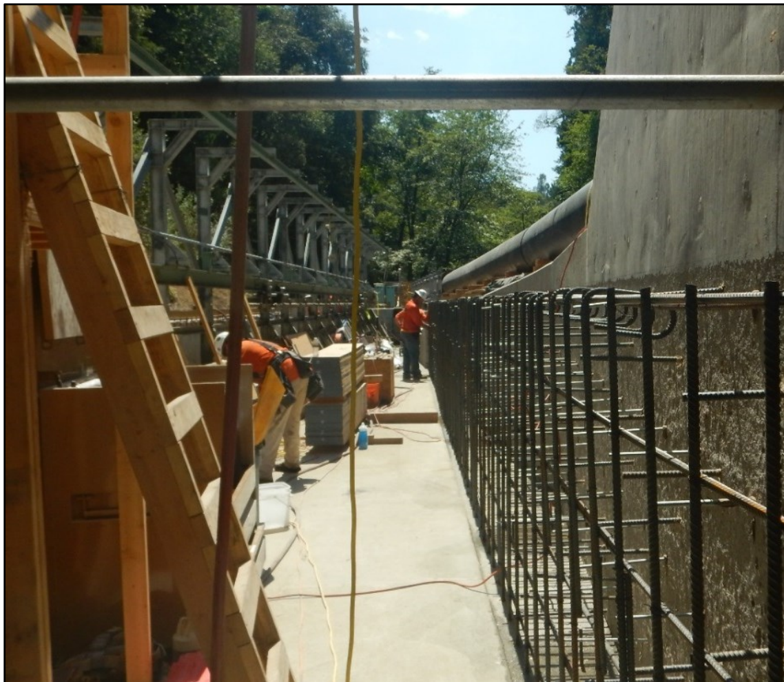
North Fork Screens and Ladder Completion Contract A view of the completed rebar for the wall extension
