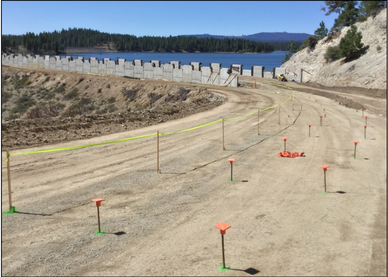
Stampede Dam, Dam Safety Modifications A view of the survey stakes marking the area for the step up leveling pad.
