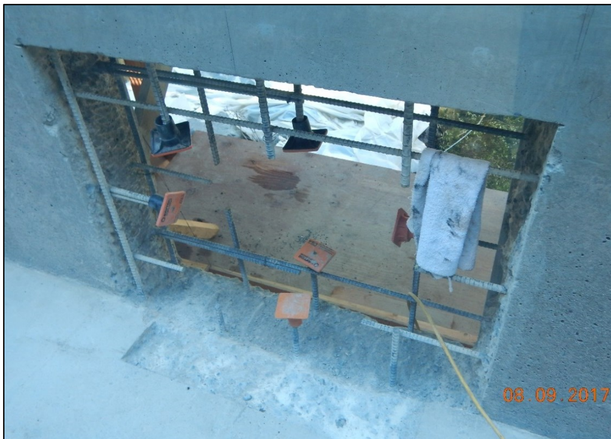
North Fork Screens and Ladder Completion Contract A view of the new slide gate opening that was chipped out this period.
