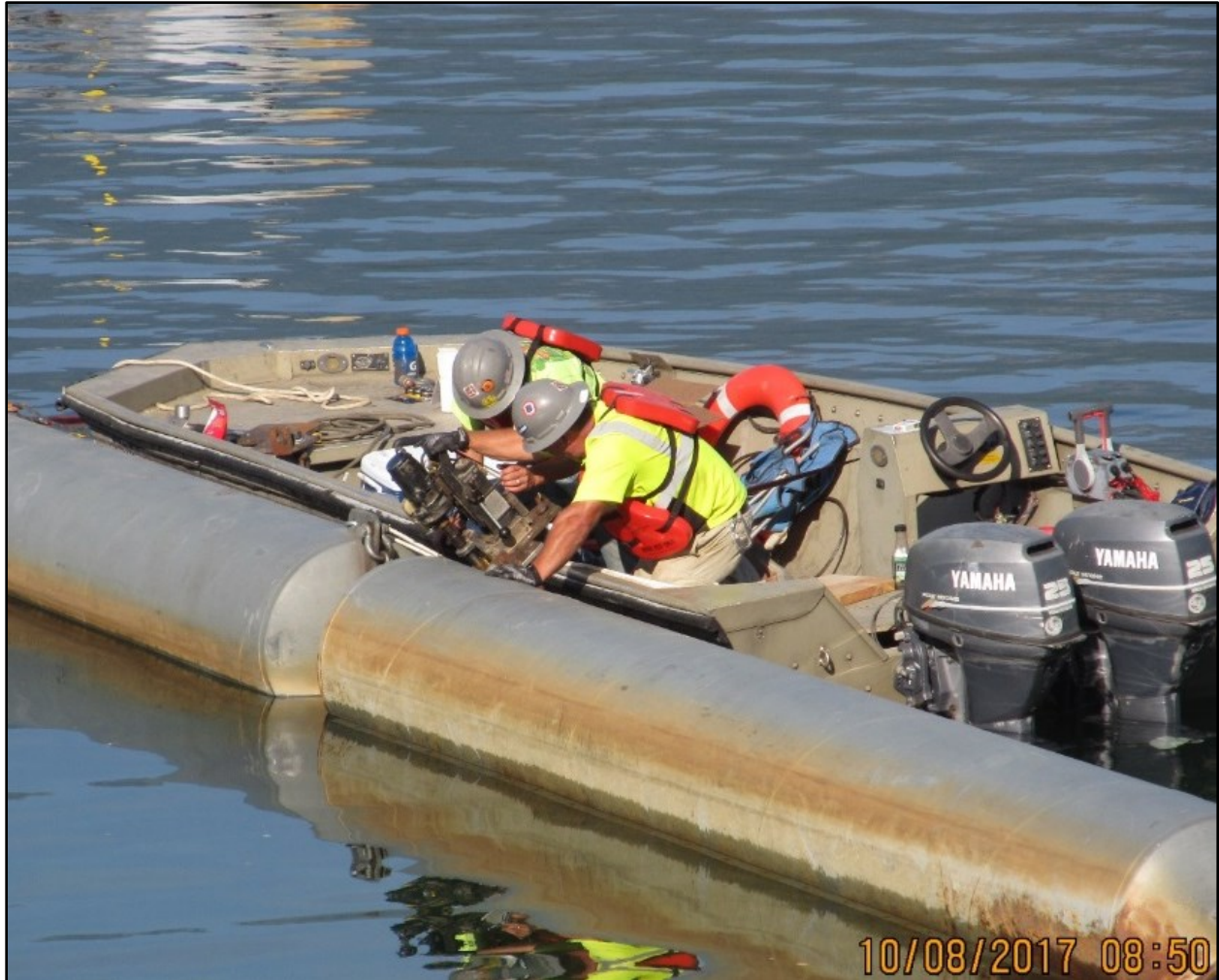
Whiskeytown Lake, Spring Creek Temperature Control Curtain A view of the contractors working on the float tank connections.
