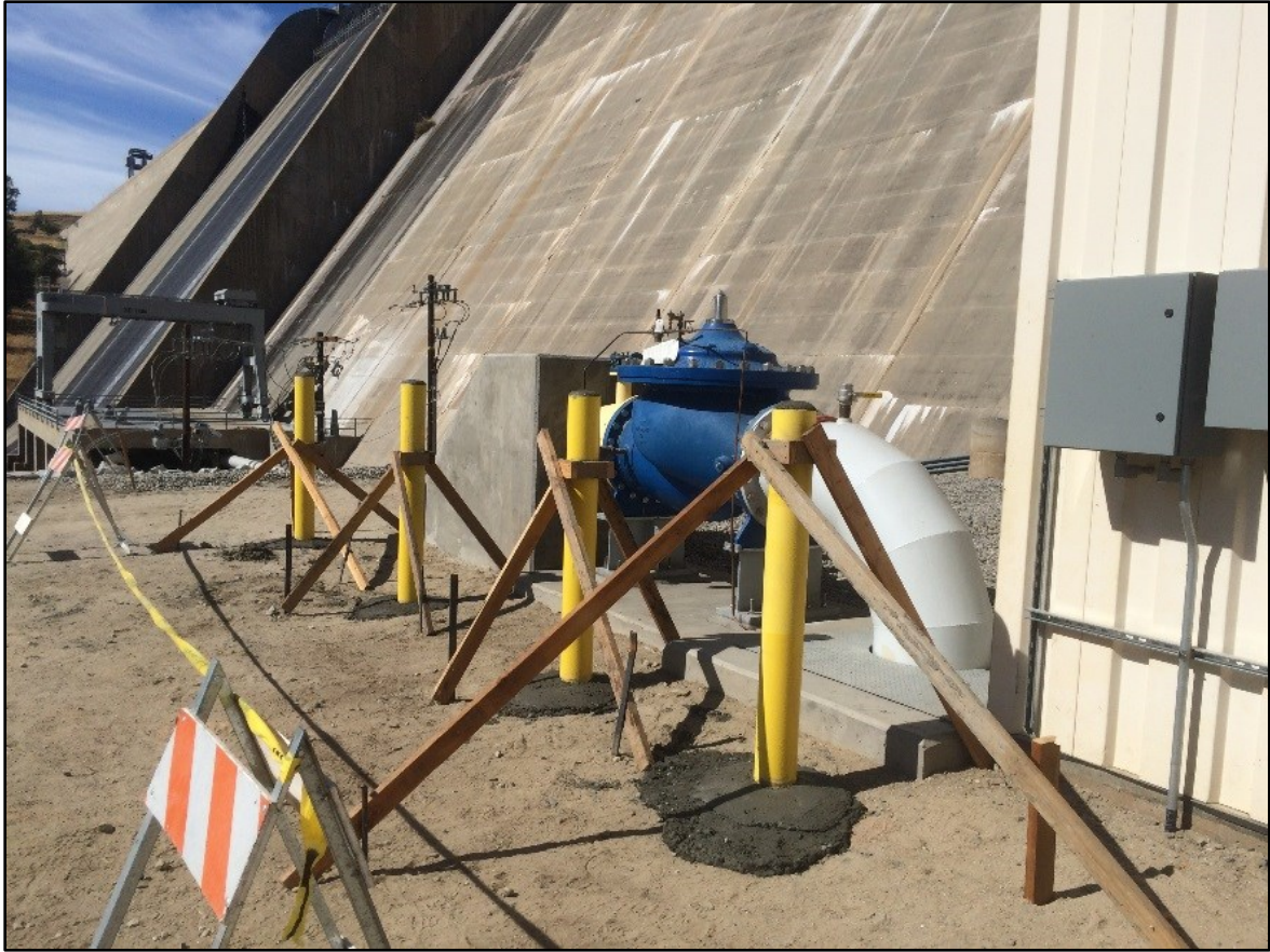
San Joaquin Hatchery Water Supply Pipeline An Image of the guard posts being set in concrete.
