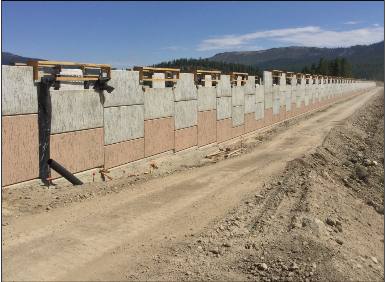
Stampede Dam, Dam Safety Modifications A view of fifth course of panels on the dike.
