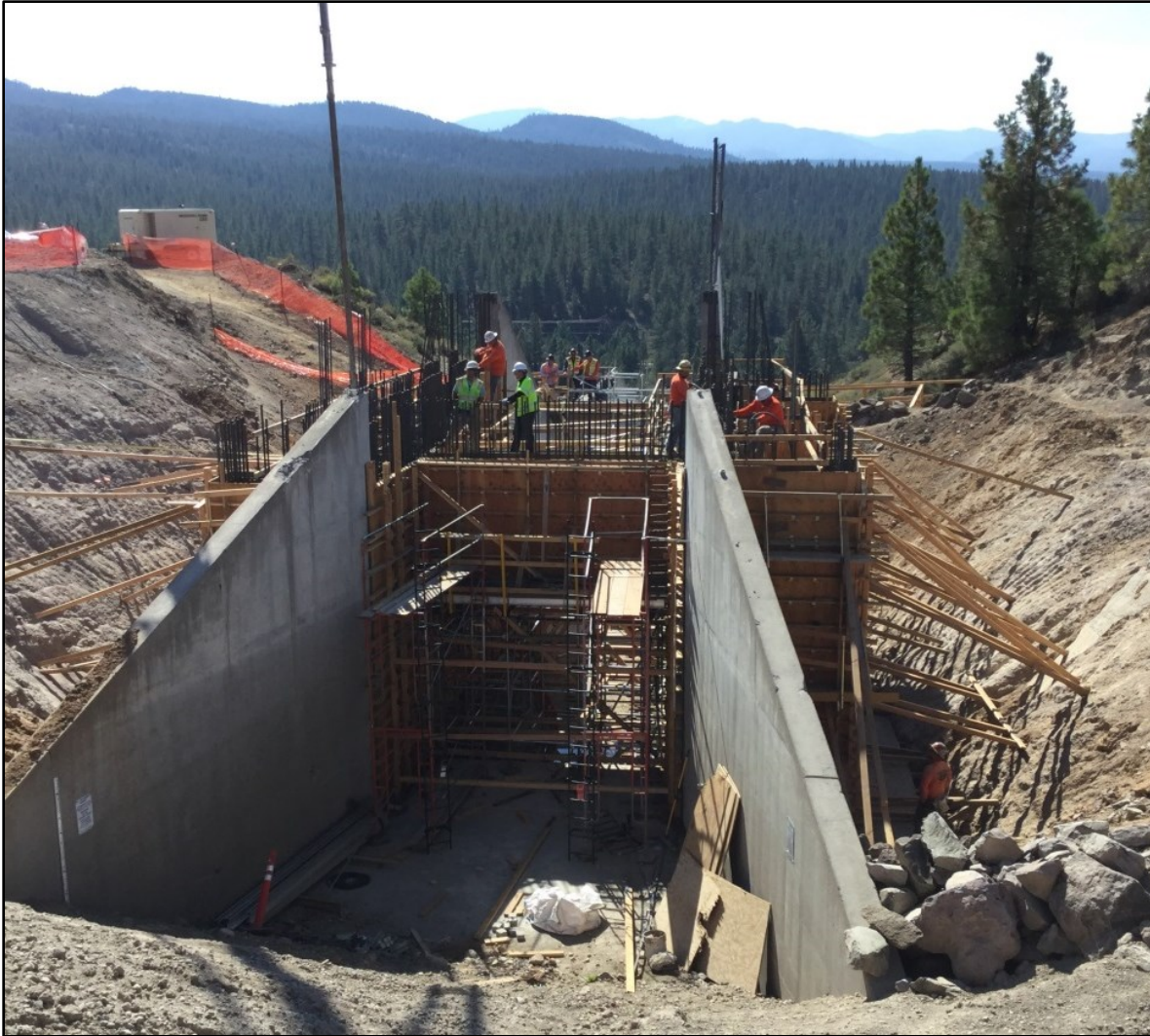
Stampede Dam, Dam Safety Modifications A view of the concrete placement for the first wall lift on the spillway.
