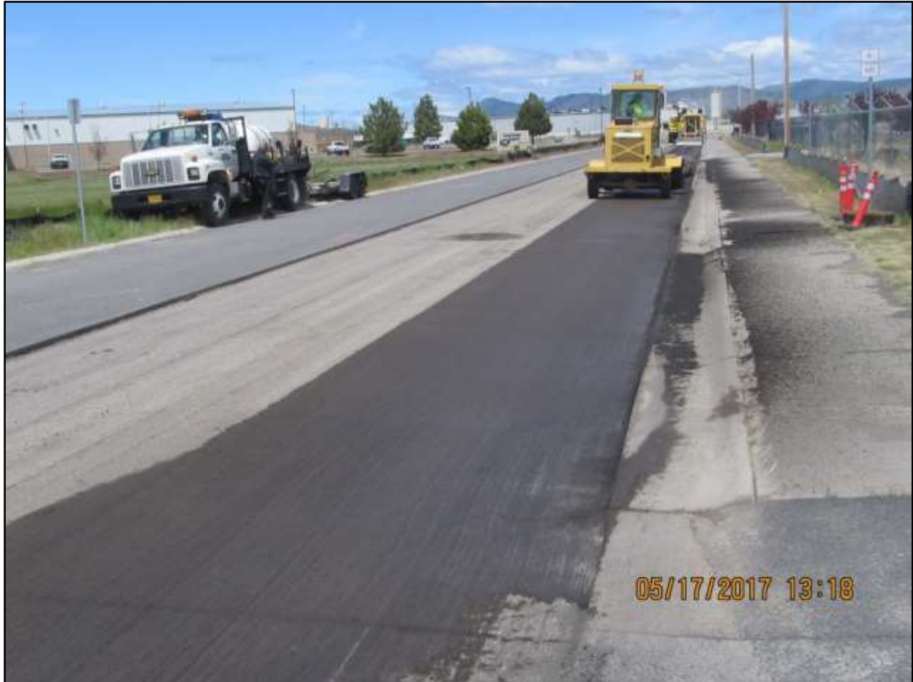
Klamath Basin Area Office Sewer Lift Station The subcontractor sweeping the Swan Court area after 2" of asphaltic cement was ground off.
