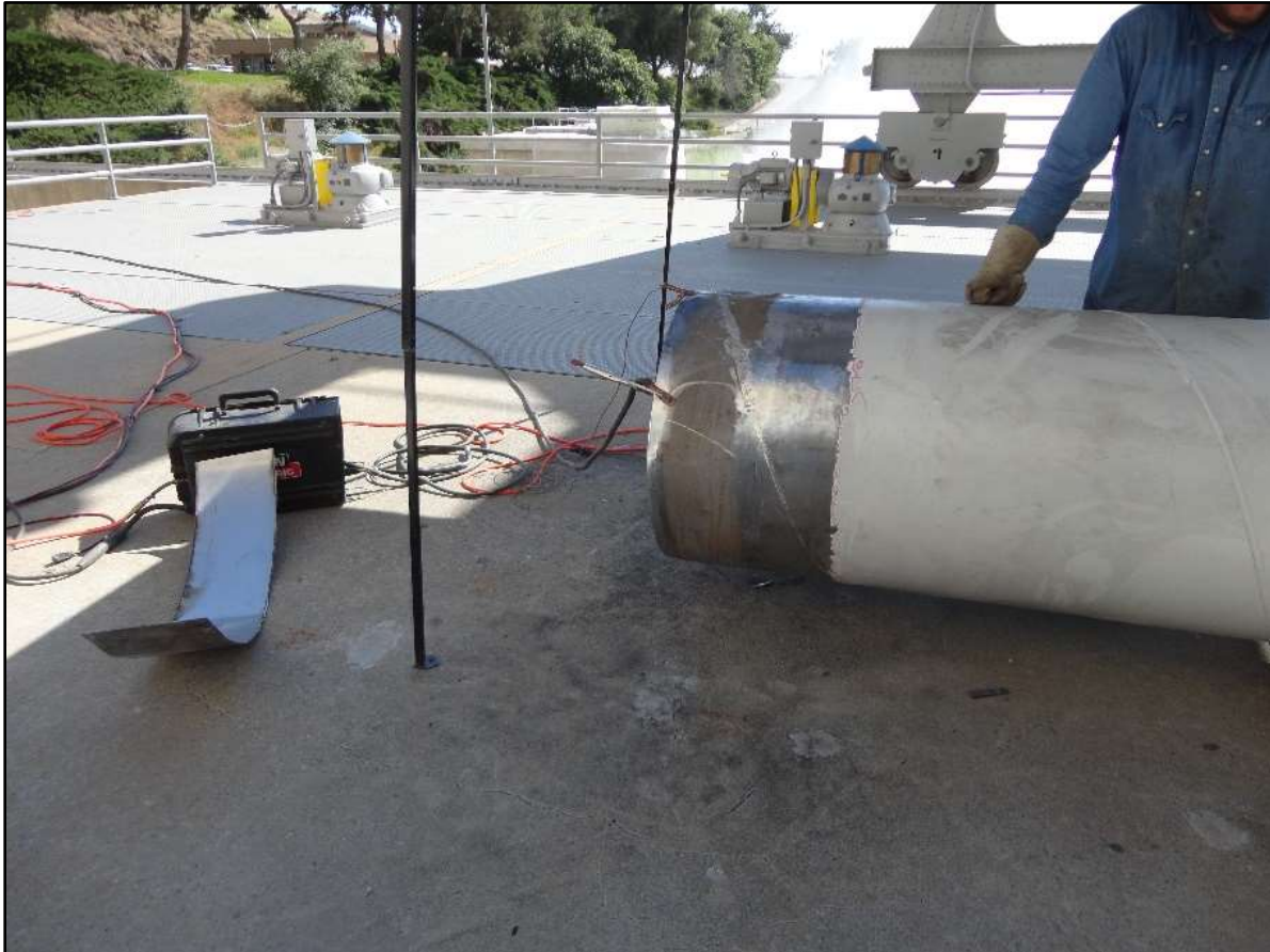
San Joaquin Hatchery Water Supply Pipeline Chapman Welding, preparing for the installation of the Baker Coupling.
