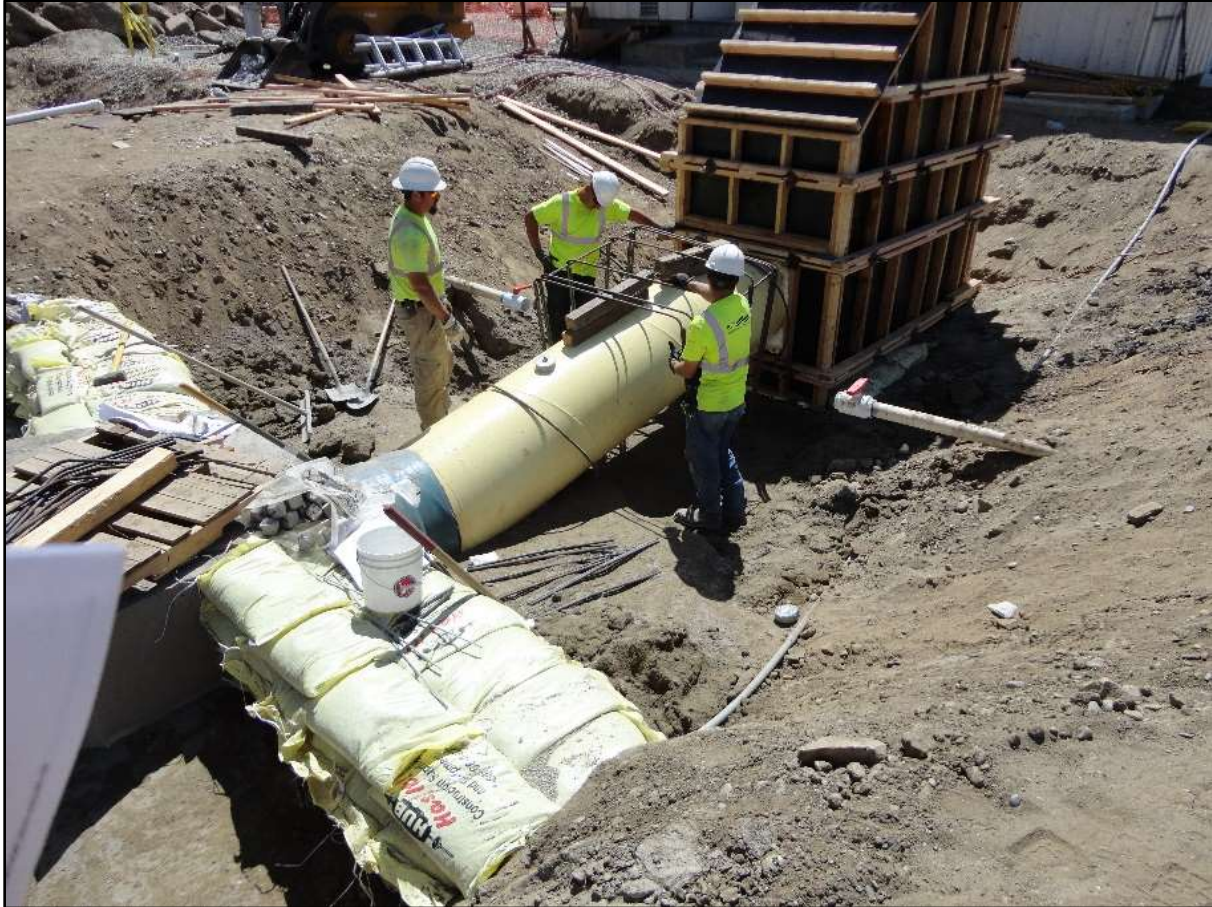
San Joaquin Hatchery Water Supply Pipeline Placing Rebar for Thrust Block Number 5
