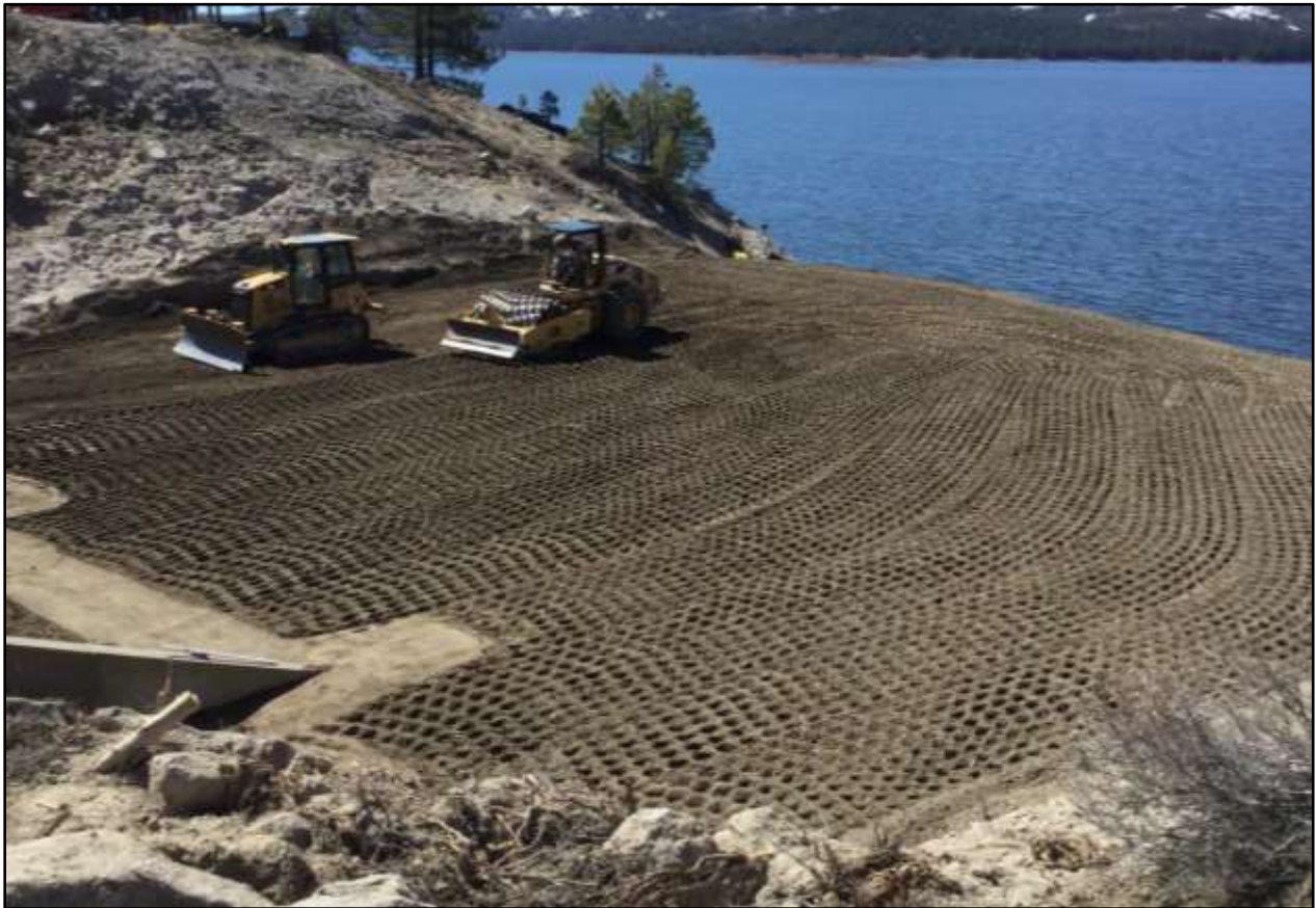
Stampede Dam, Dam Safety Modifications An image of the earthfill cofferdam under construction
