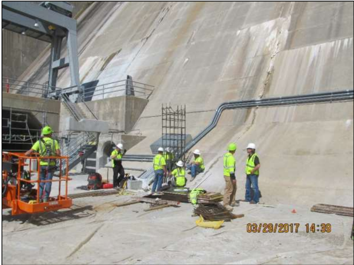
San Joaquin Hatchery Water Supply Pipeline The Contractor installing reinforcement for Column No. 1.
