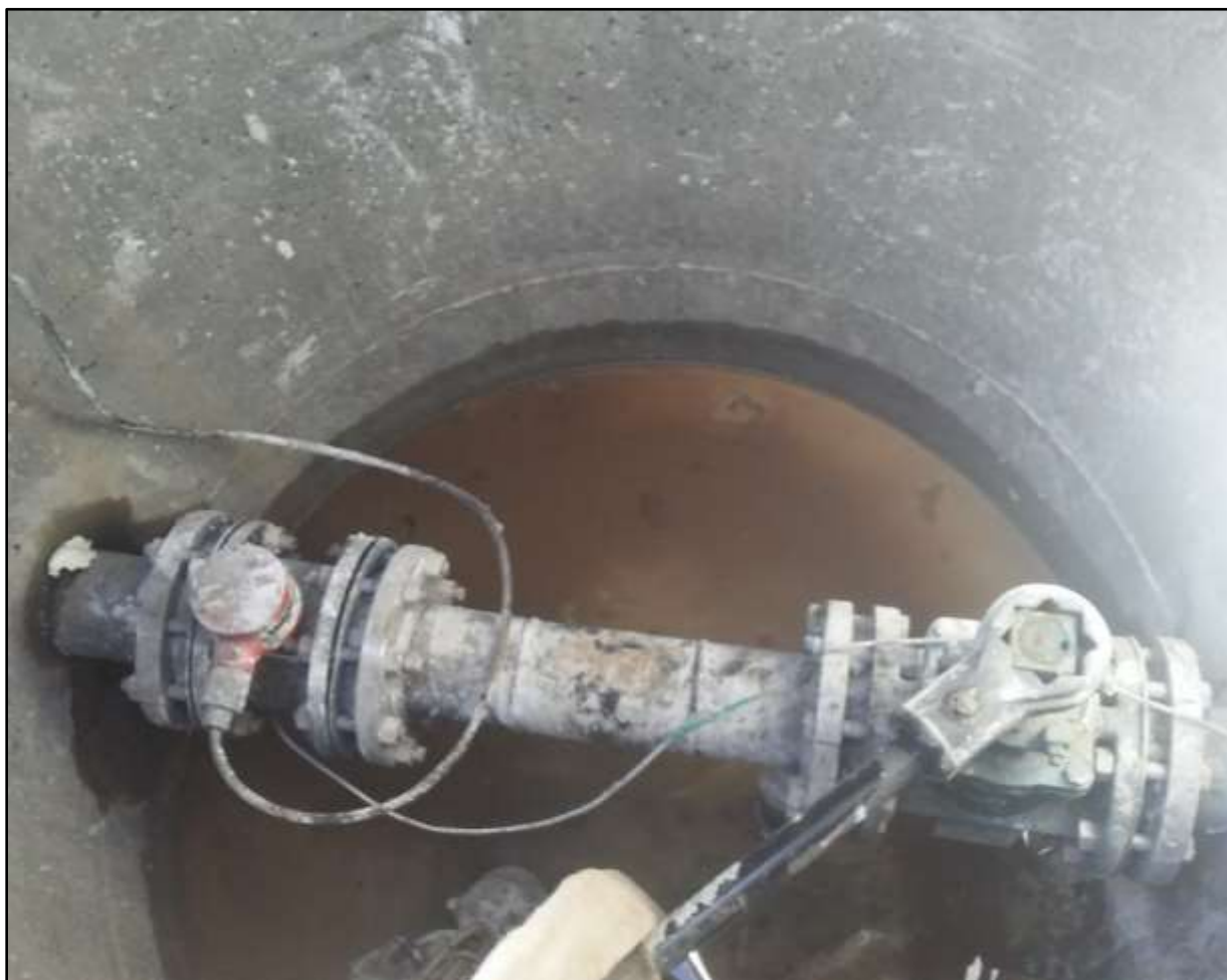
Klamath Basin Area Office Sewer Lift Station A view of the vault where water was found to be seeping two weeks after the warranty repairs were made.
