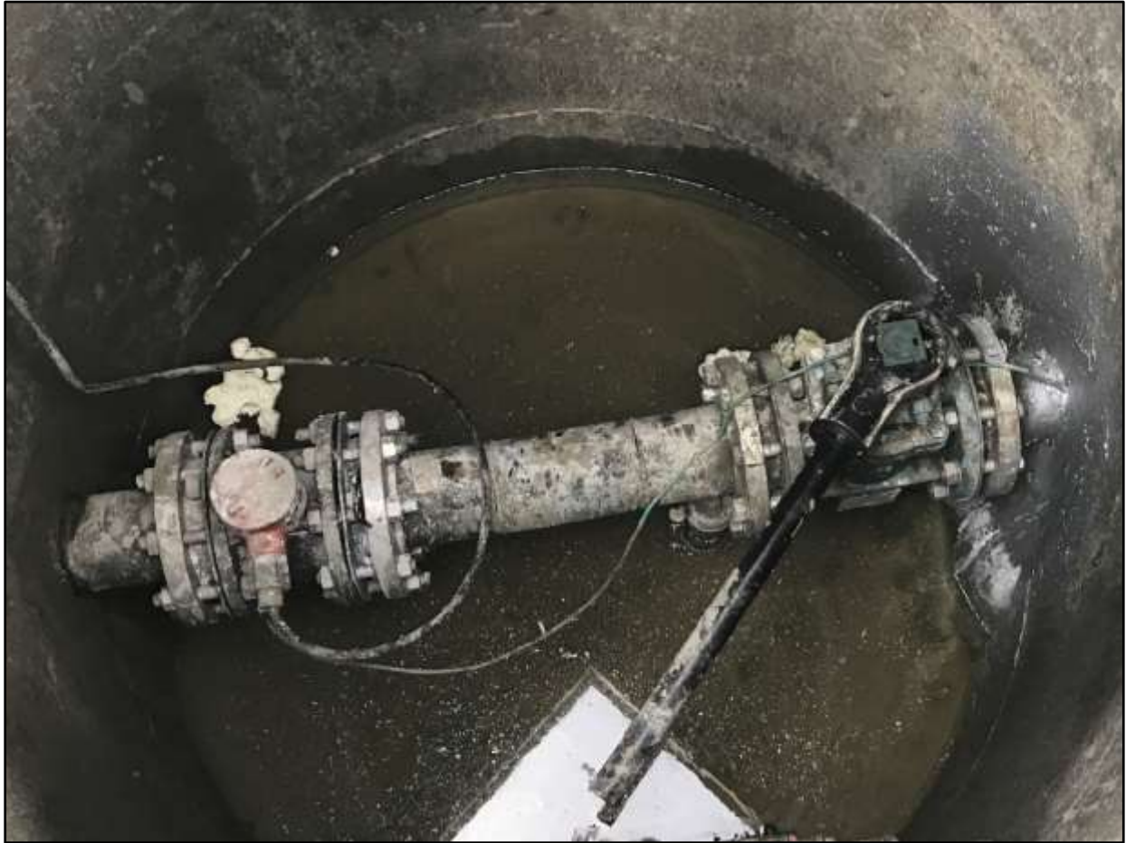
Klamath Basin Area Office Sewer Lift Station A view of the vault where water was found to be seeping.
