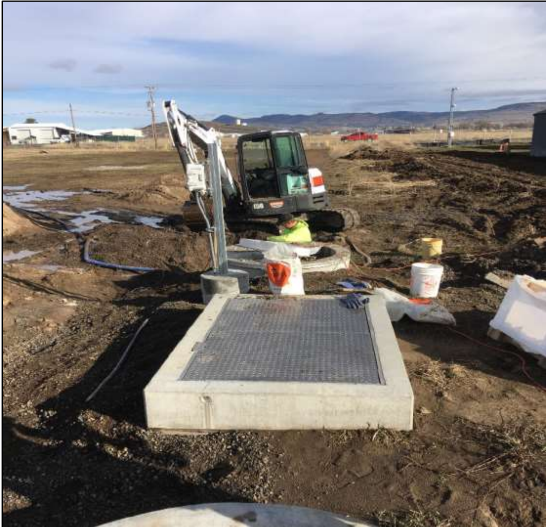
Klamath Basin Area Office Sewer Lift Station The Subcontractor making warranty repairs on the vault.
