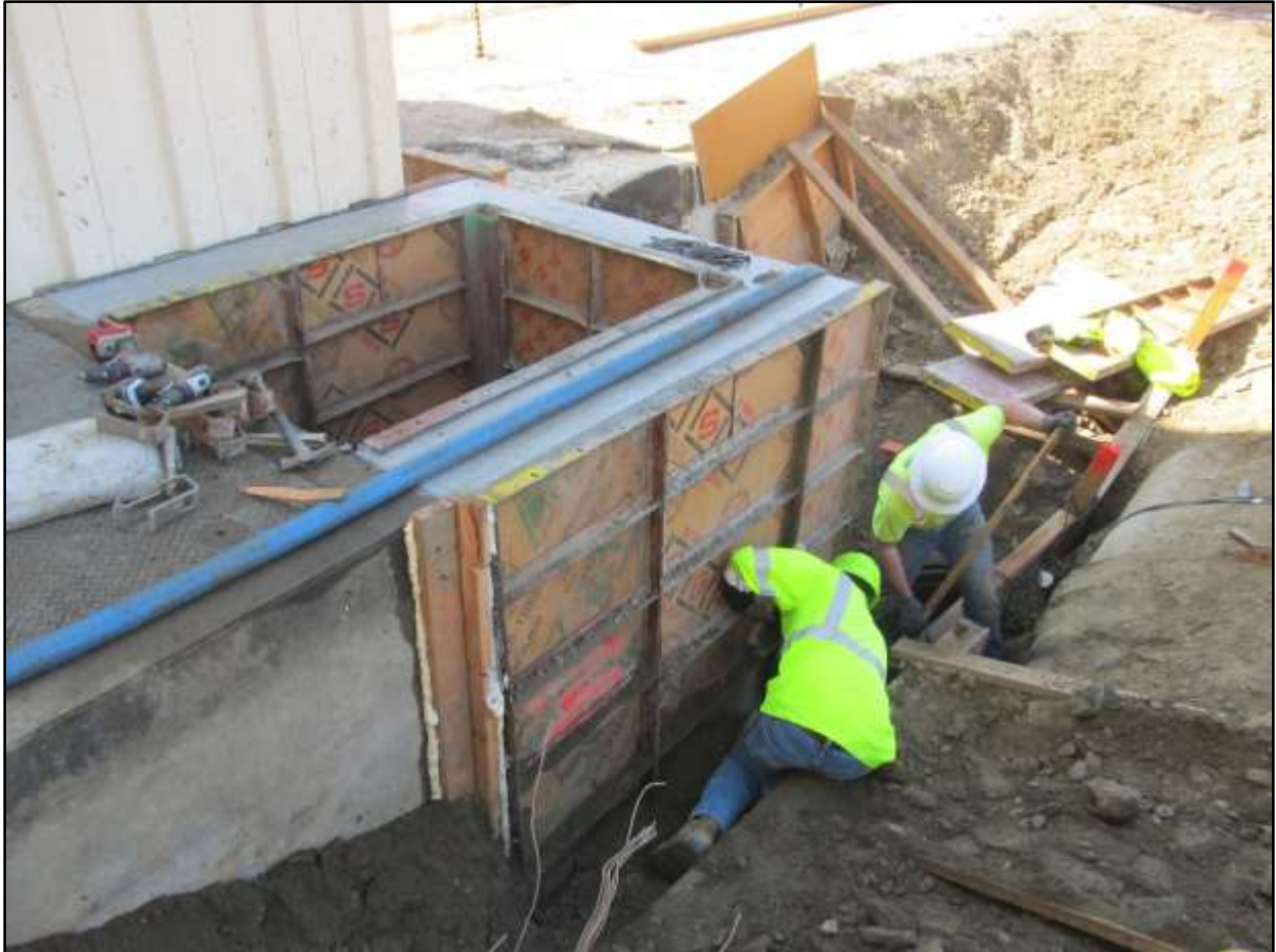
San Joaquin Hatchery Water Supply Pipeline Contractor removing the form work for the new discharge vault.
