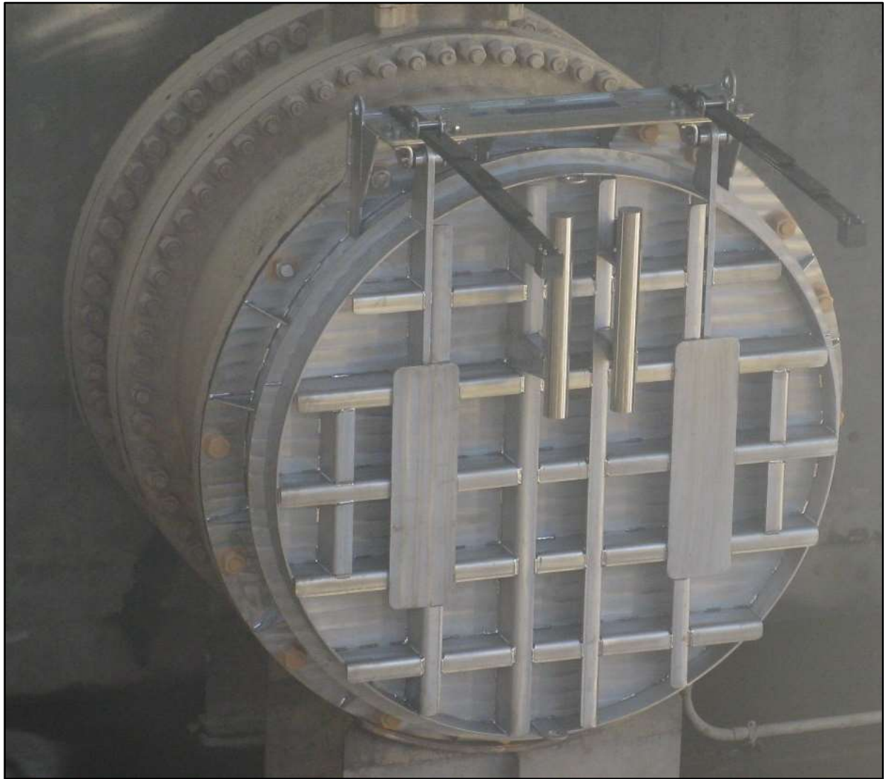
Red Bluff Flap Gate Retrofit A view from downstream of a newly Installed stainless steel flap gate.
