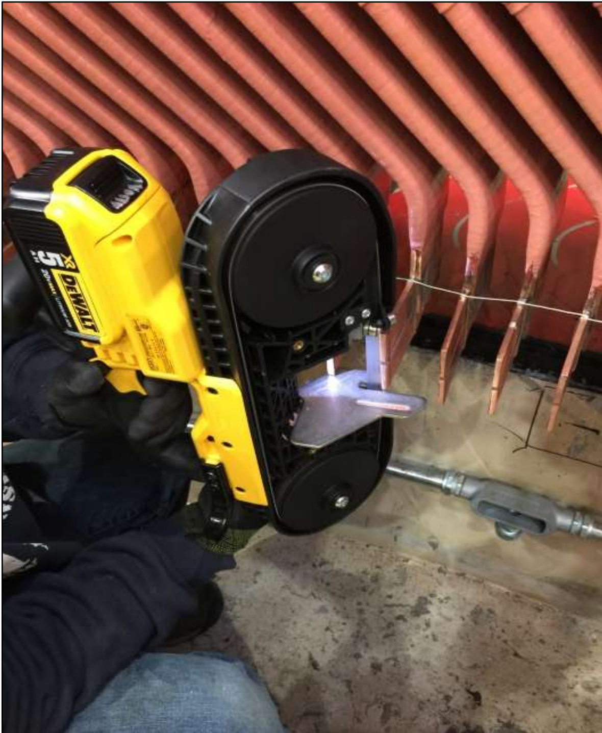
Trinity Powerplant Generator Rewinds The Contractor trimming the bar clips so that overlapping does not occur.
