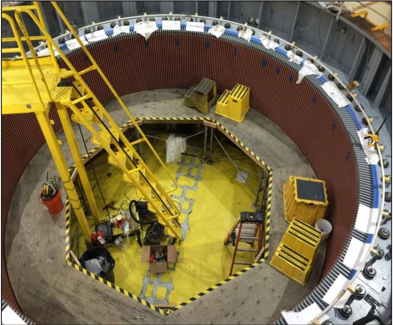
Trinity Powerplant Generator Rewinds A view of the Stator Bore.
