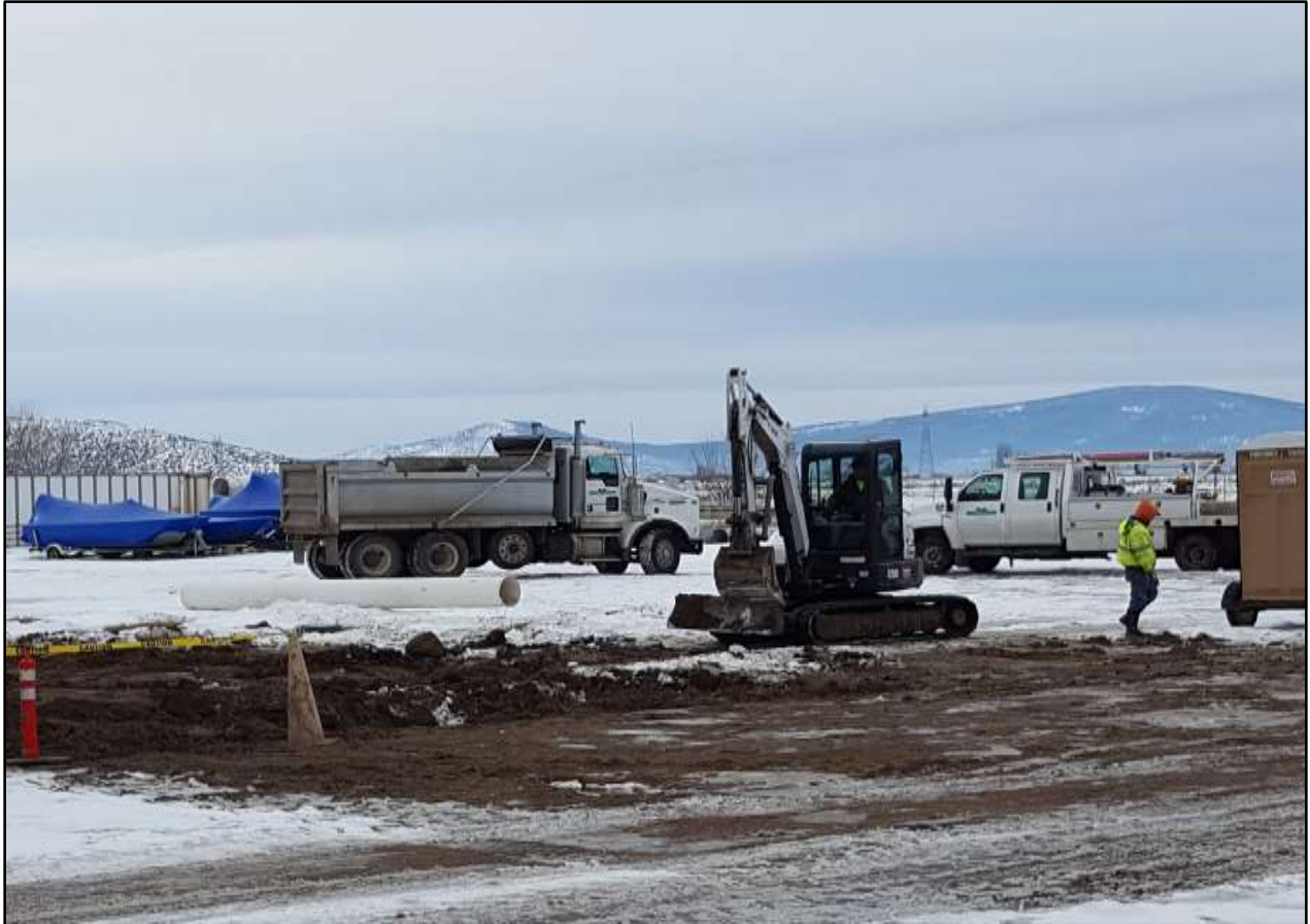
Klamath Basin Area Office Sewer Lift Station The subcontractor leveling the ground after the removal of the old leach fields.
