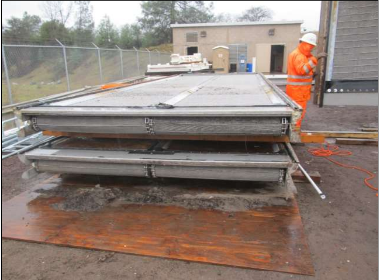
Intake 3 Screen Extension, Coleman National Fish Hatchery A view of the stacked fish screens after they had been removed
