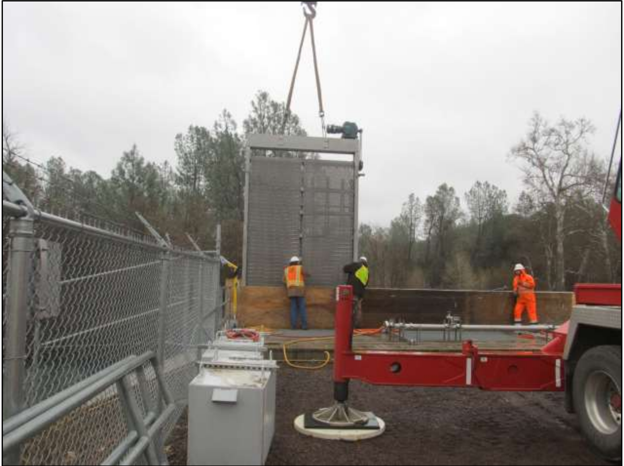
Intake 3 Screen Extension, Coleman National Fish Hatchery A view of the contractors removing Screen 1
