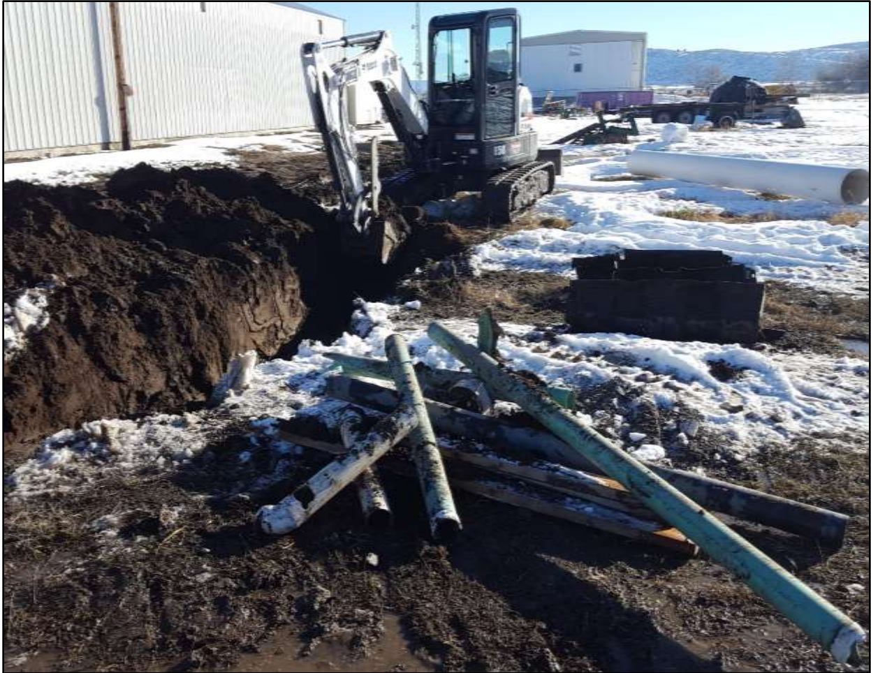
Klamath Basin Area Office Sewer Lift Station The subcontractor removing the old leach field piping.
