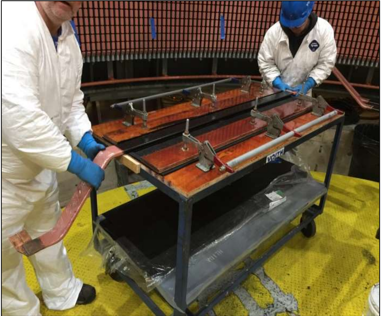
Trinity Powerplant Generator Rewinds The Contractor insulating the bottom bar with conductive paper.
