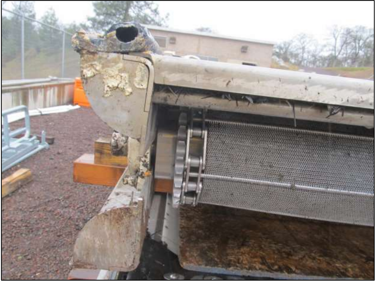
Intake 3 Screen Extension, Coleman National Fish Hatchery A view of the belting chain on screen 3 off of the sprocket
