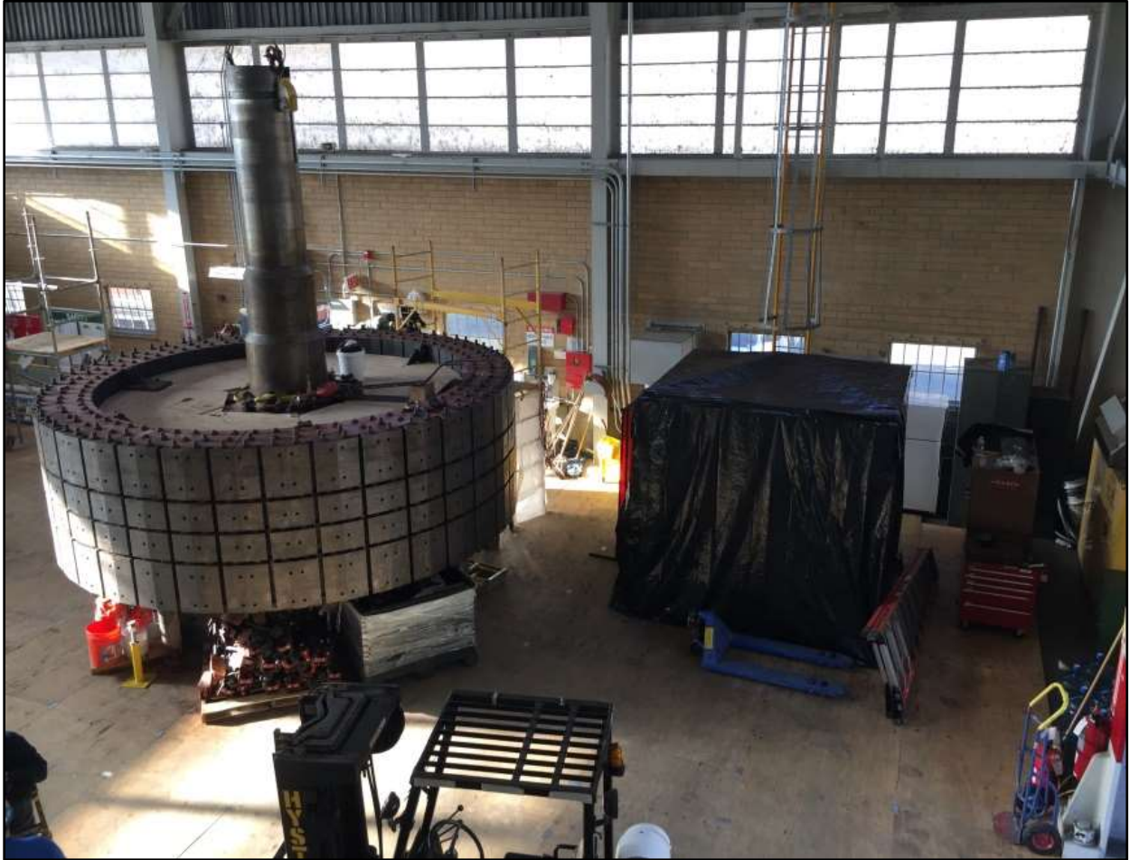
Trinity Powerplant Generator Rewinds A view of the rotor rim steel without the poles
