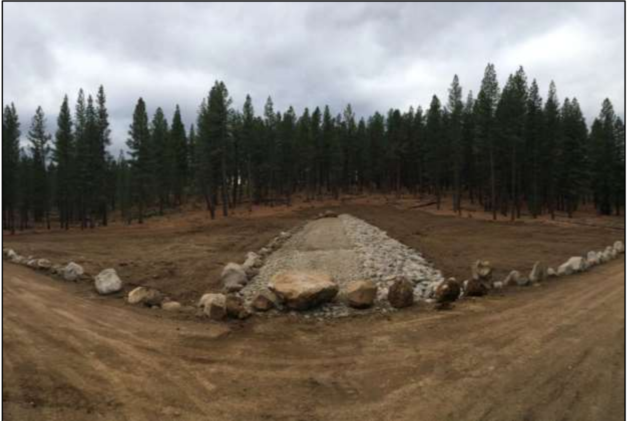
Stampede Dam – Dam Safety Modifications A view of the West Saddle Dike After Completion.
