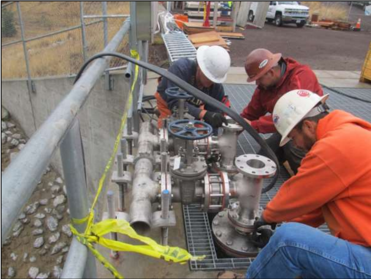
Intake 3, Screen Extension, Coleman National Fish Hatchery Contractor Services Group employees installing the spray water system.
