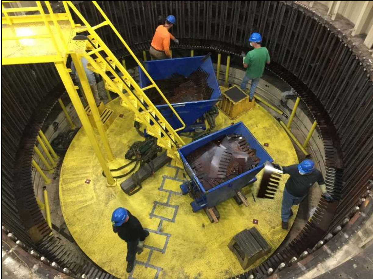
Trinity Powerplant Generator Rewinds The Contractor in the process of removing the stator core
