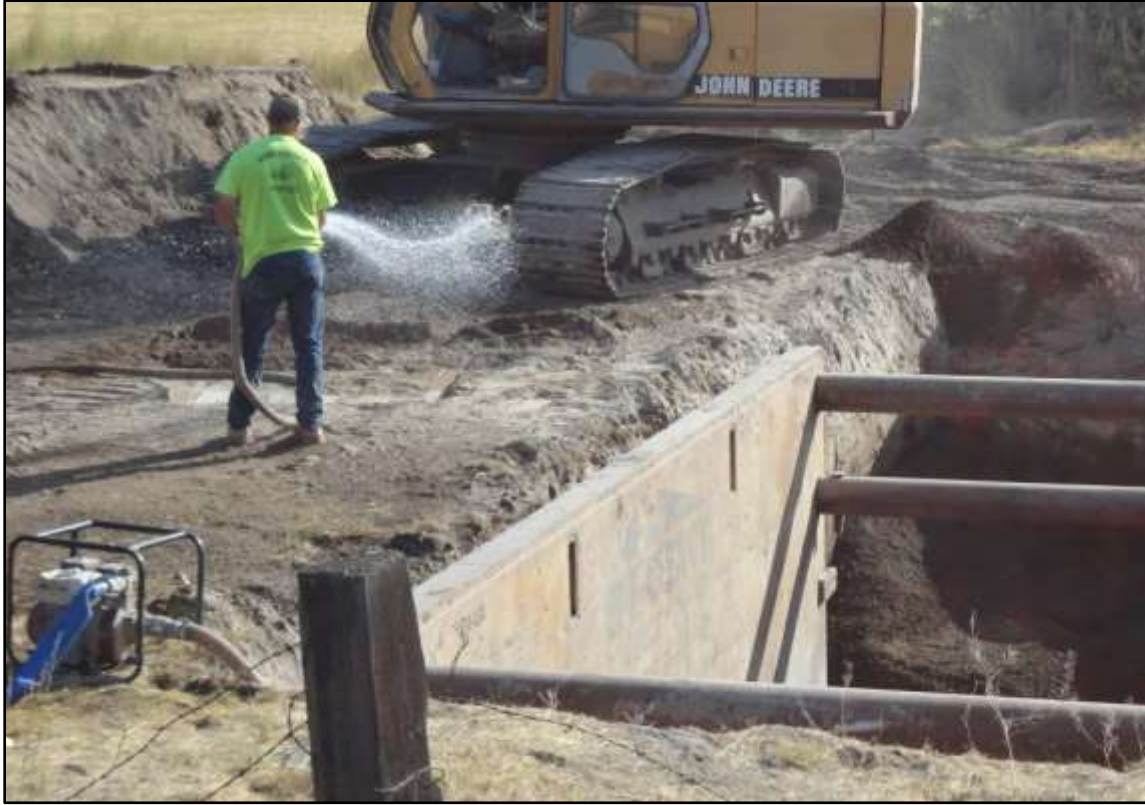
Klamath Basin Area Office Sewer Lift Station Subcontractor Bob's Excavating used \frac{3}{4} -inch aggregate to backfill the bore pit, following removal of the trench shoring. Density testing on the backfill indicated specified results were achieved.
