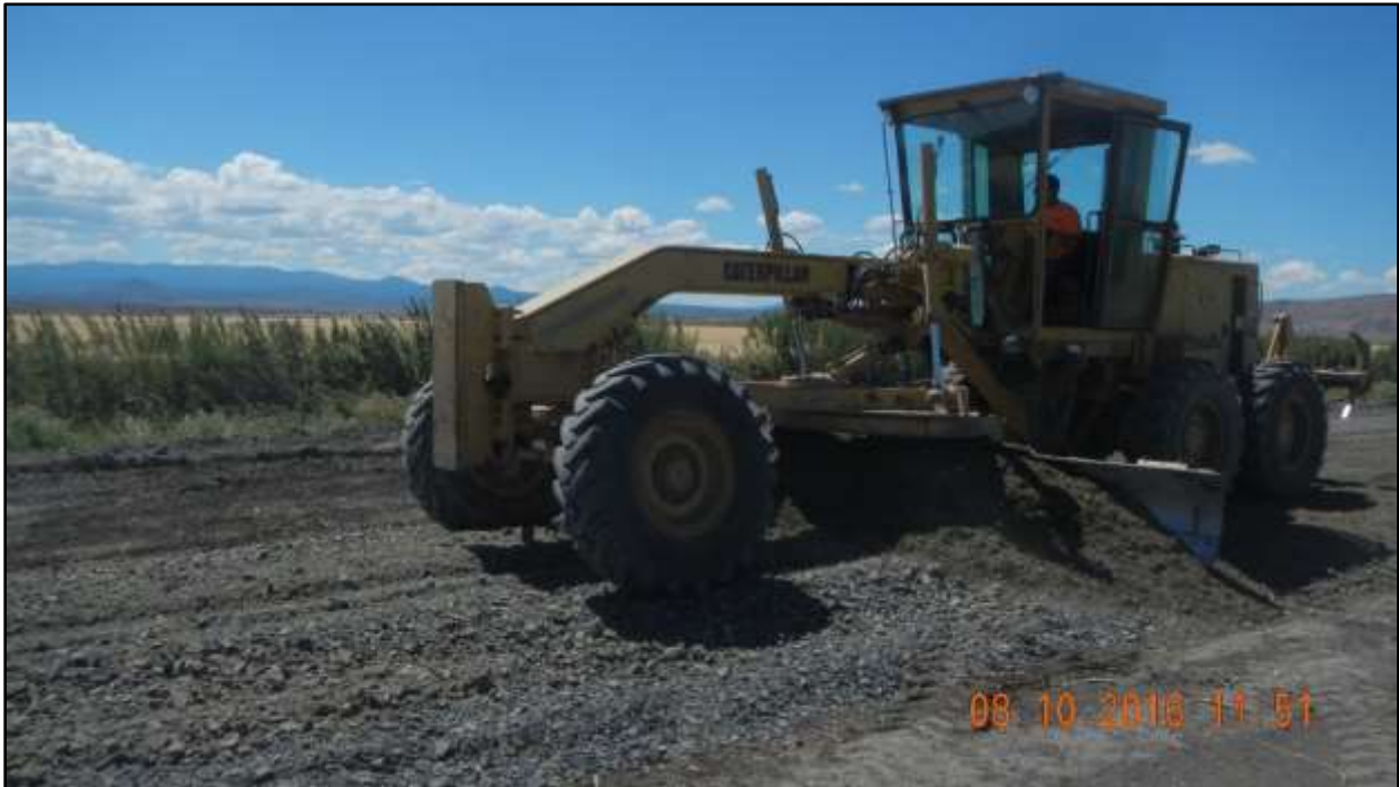
Tule Lake Road Improvements Project The Contractor Spreading the \frac{3}{4} -inch minus material on Pump W Road.
