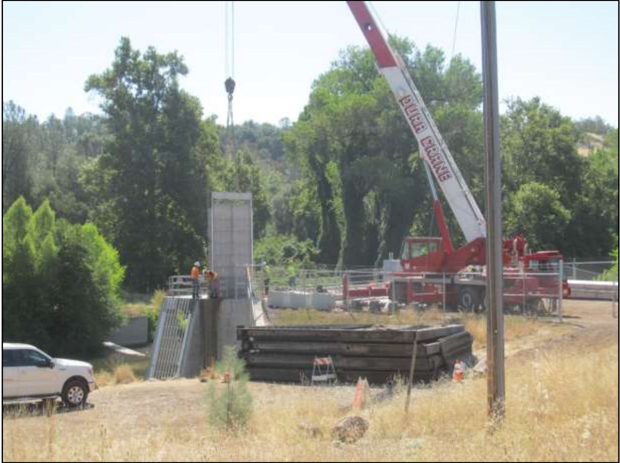
Intake 3 Screen Extension Coleman National Fish Hatchery Subcontractor Dura Crane assisting Contractor Services Group with the installation of the fish screens.
