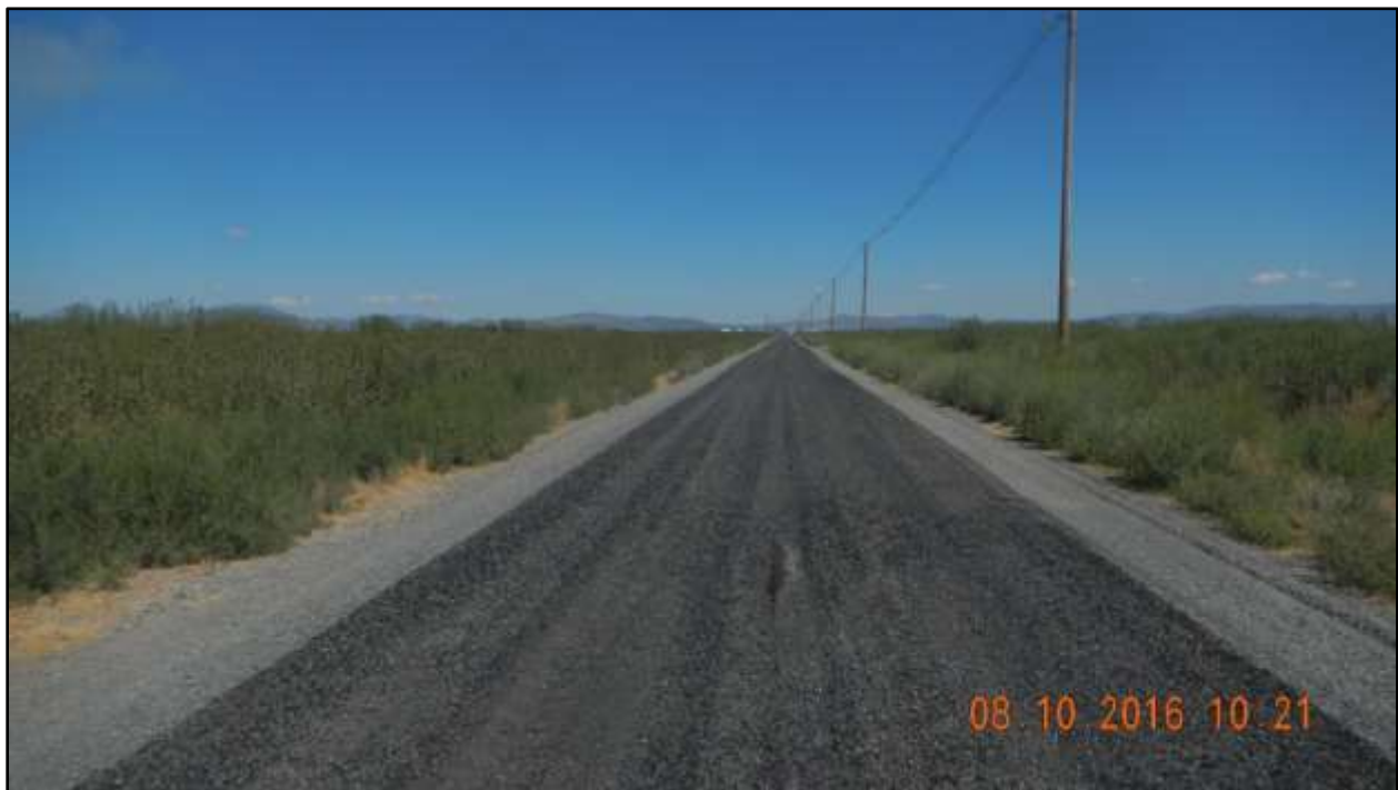
Tule Lake Road Improvement Project A Picture Showing the Dust Palliative on Pole Line Road North of Hunt Shack Road
