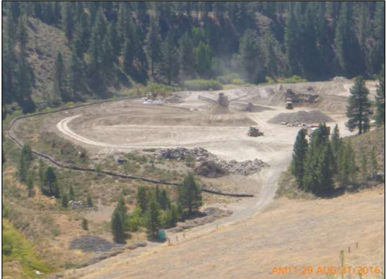
Stampede Dam – Dam Safety Modifications A View of The Operational Borrowing Area after the vegetation and trees had been removed.
