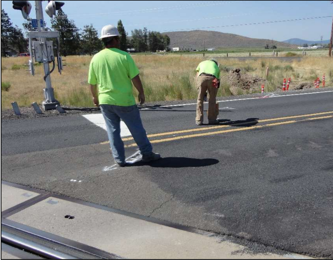
Klamath Basin Area Office Sewer Lift Station The contractor marking the drill head location with paint after using a magnetometer to find its location.
