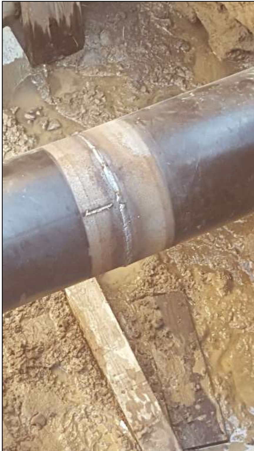
Klamath Basin Area Office Sewer Lift Station A photo showing the welds performed on the boring casing pipe.
