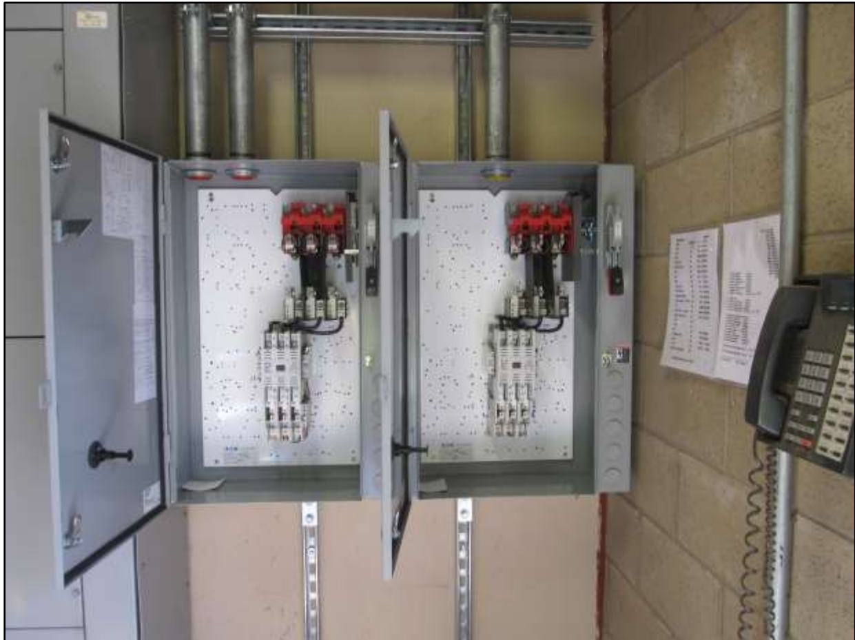
Intake 3, Screen Extension Coleman National Fish Hatchery The two new electrical boxes installed for the new sump pump motors.
