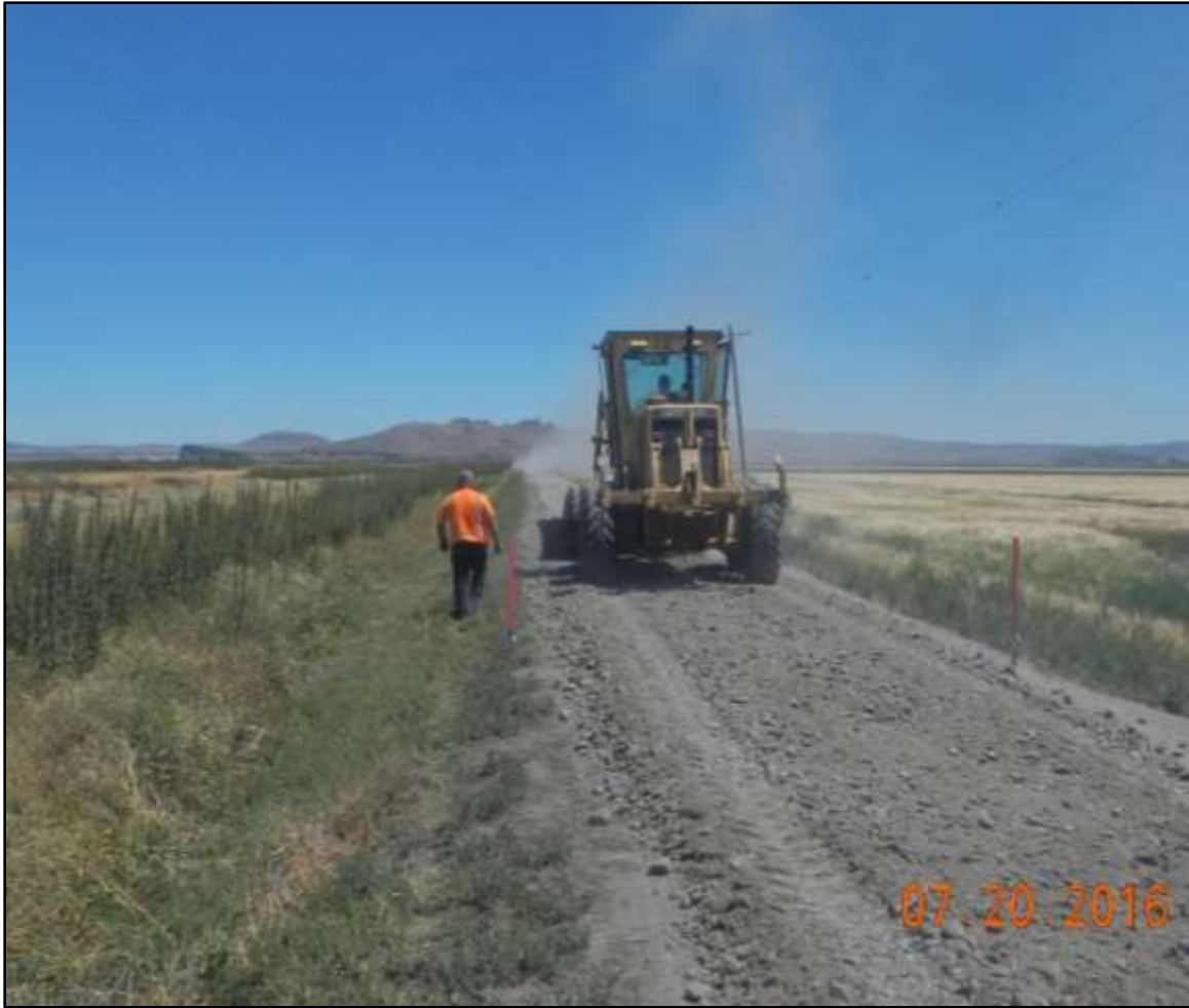
Tule Lake Road Improvements Project Material being spread and compacted in two lifts along Pump 10 Road
