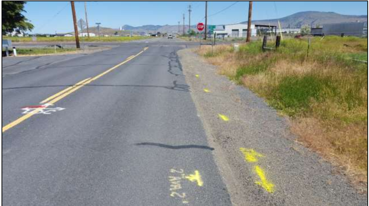
Klamath Basin Area Office Sewer Lift Station A view of the marks showing where underground utilities are located near the site.
