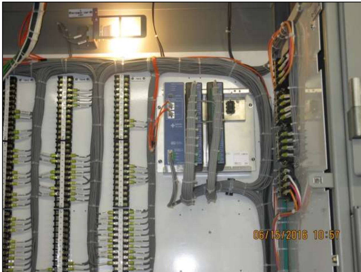
Tracy 13.8kV Switchgear/Breaker Replacement SEL In/Out (I/O) equipment and power coupler in building UZ6A F17 upper breaker cubical
