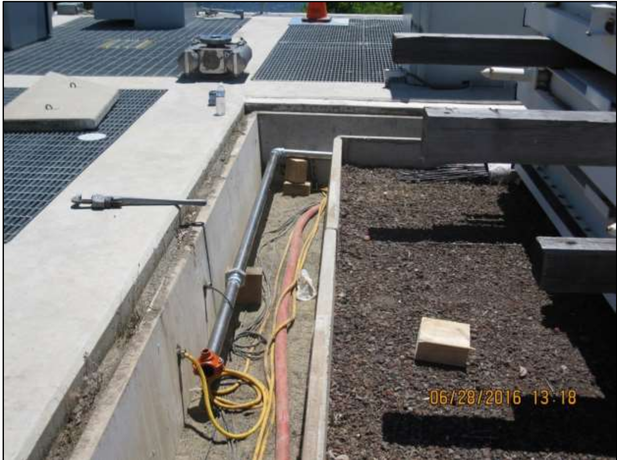
Intake 3, Screen Extension Coleman National Fish Hatchery Installing the stainless steel air burst piping in the cable trench.
