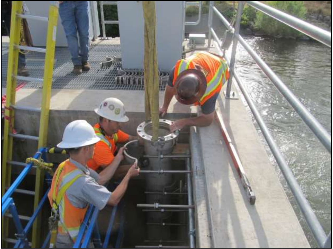
Coleman National Fish Hatchery - Intake 3 Screen Extension Contractor Service Group crew members installing the brackets for the new submersible vertical pump casings
