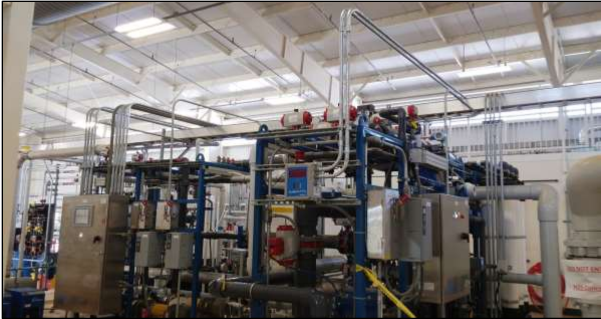
San Luis Demonstration Treatment Plant Photo of Ultra-Filtration (UF) System with the newly installed hydrogen sulfide (H 2 S) monitored installed
