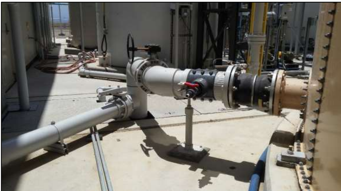
San Luis Demonstration Treatment Plant Photo of newly installed pressure indicating transmitter on the discharge of the ABMet Effluent Tank to monitor the liquid level in the tank
