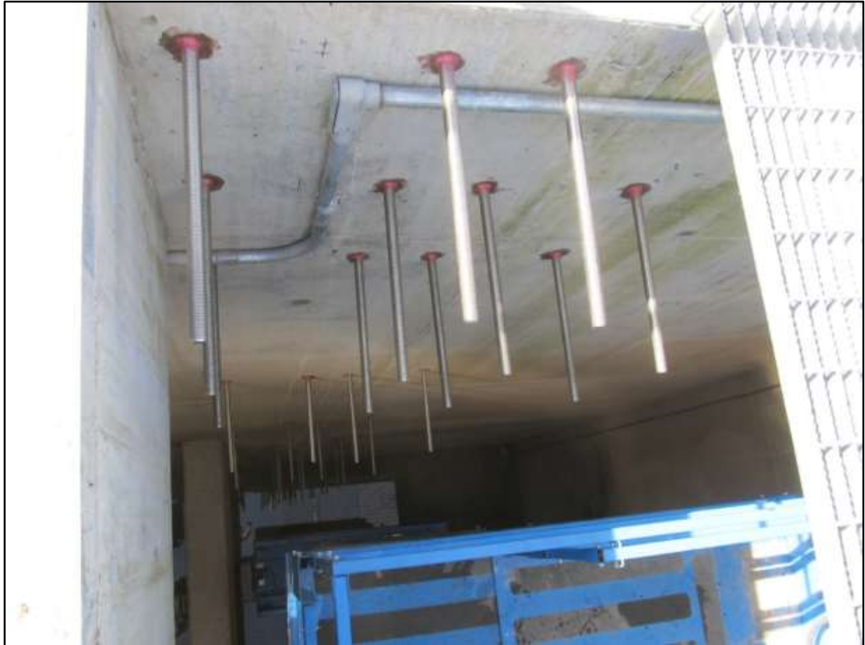
Coleman National Fish Hatchery - Intake 3 Screen Extension A view of the 1" diameter stainless steel rods that were installed
