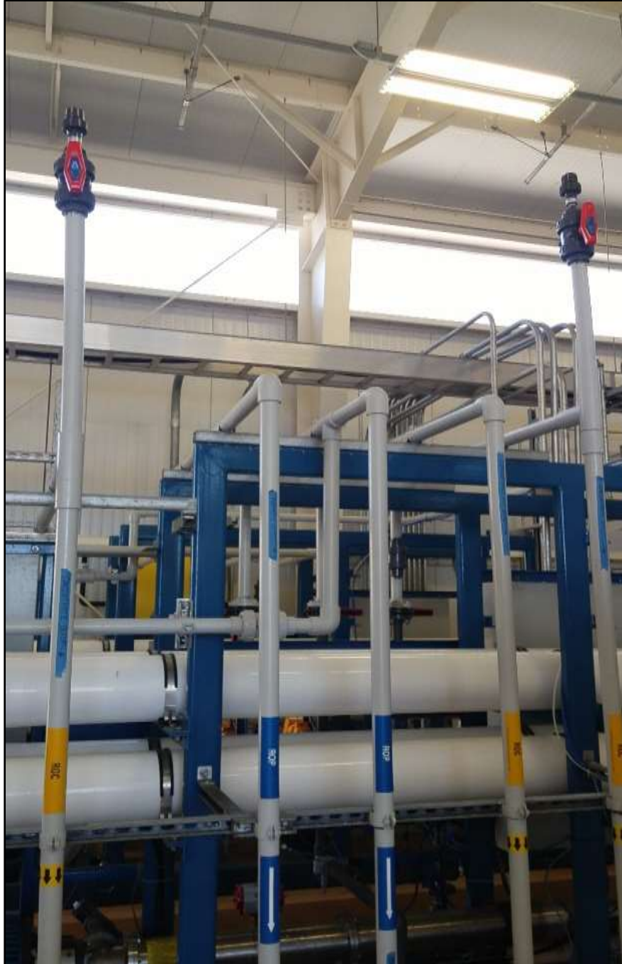
San Luis Demonstration Treatment Plant The newly installed air release valves at the reverse osmosis systems to aid in operations
