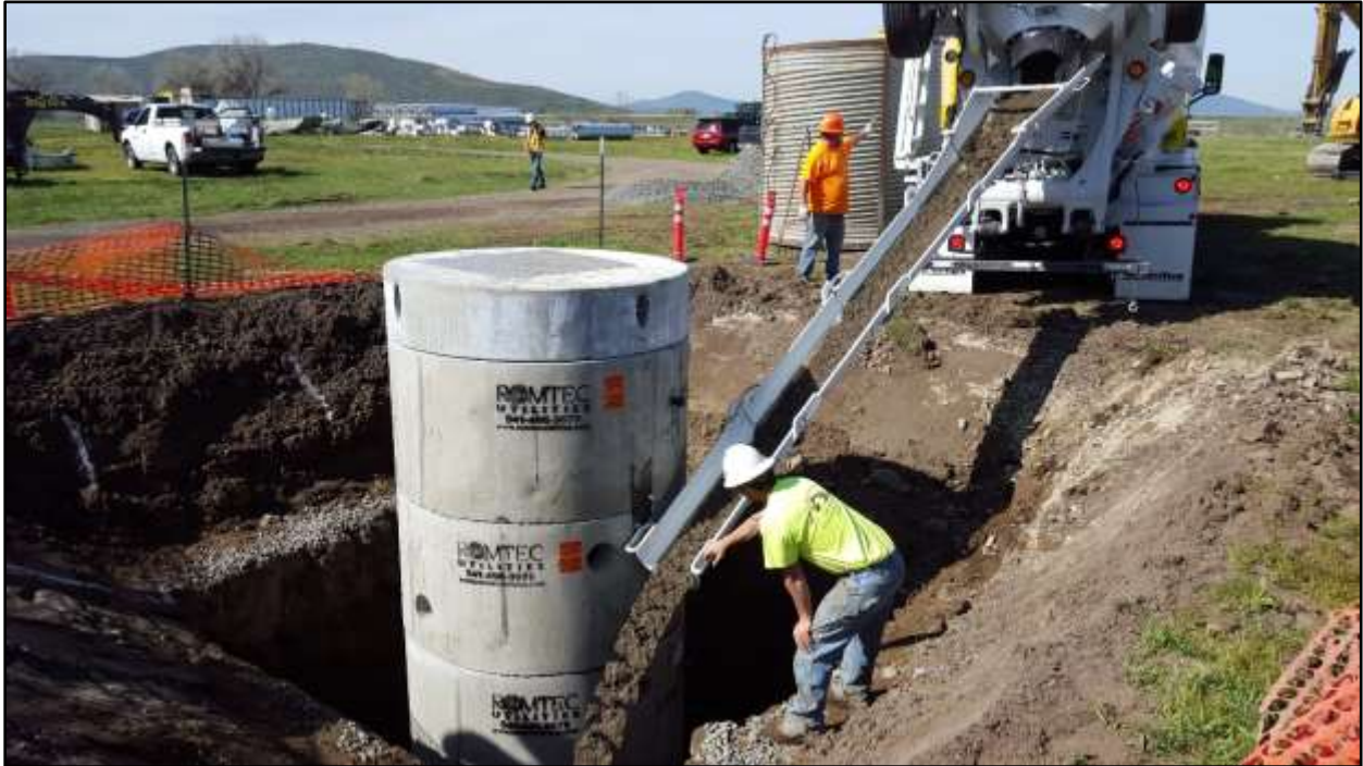
Klamath Basin Area Office Controlled Low Strength Material was used to backfill around the wet well structure to a depth of 5 feet below existing soil grades
