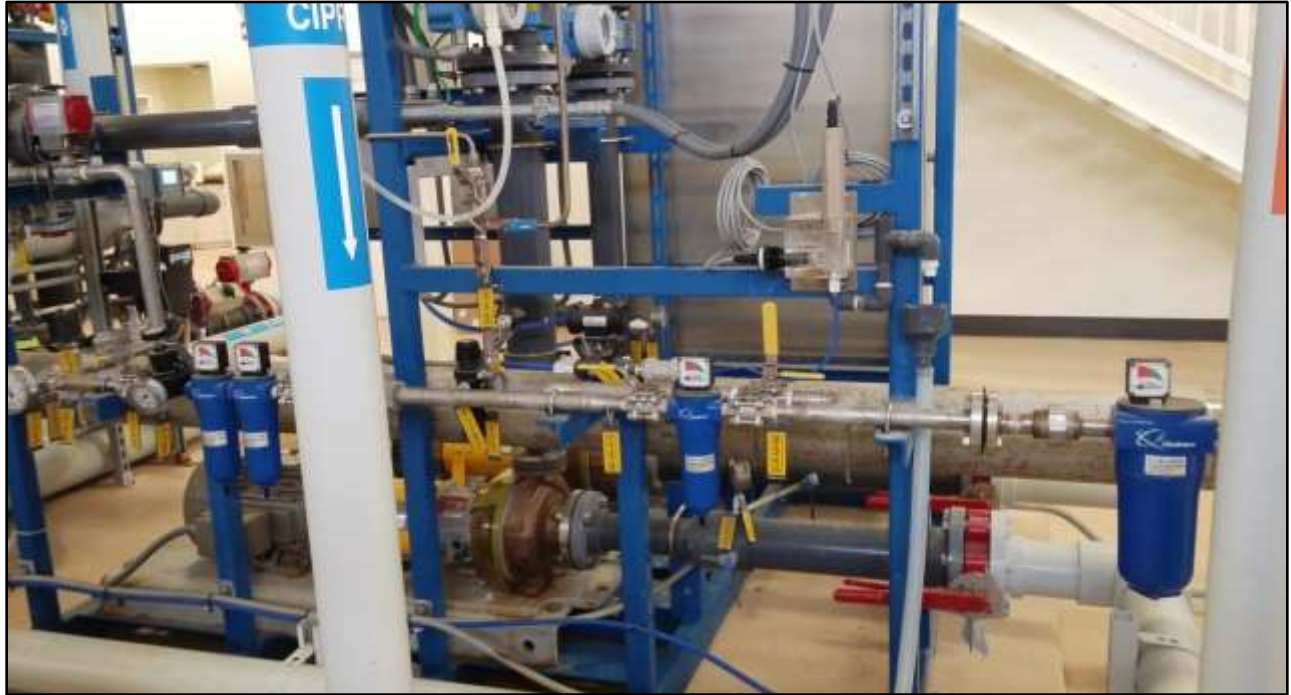
San Luis Demonstration Treatment Plant The inline air filter housings on the Ultra-Filtration System
