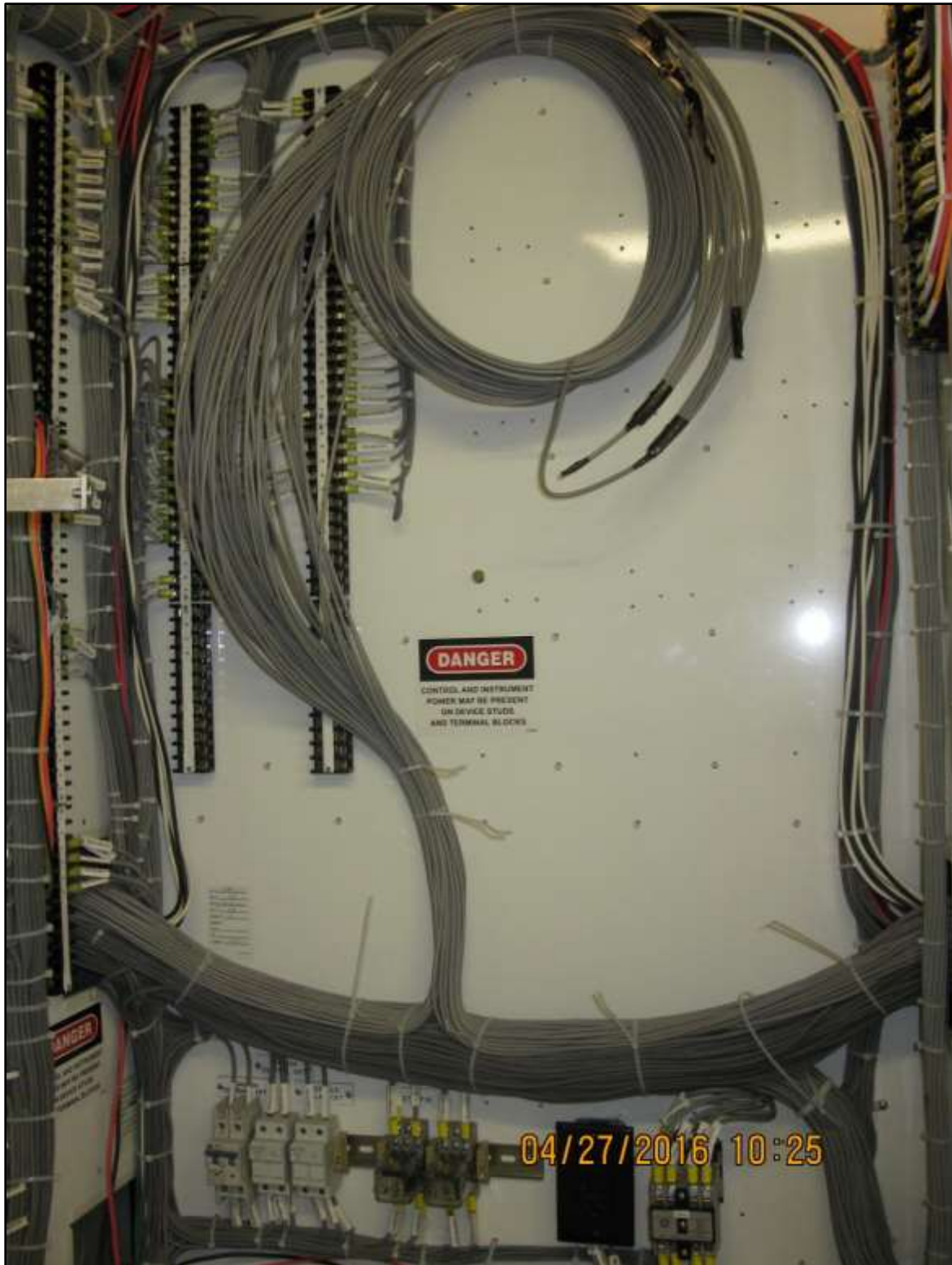
Tracy 13.8kV Switchgear/Break Replacement Upper Section 4 in building UZ11A with new SIS wires run from each upper cubicle to the Location of the new I/O equipment
