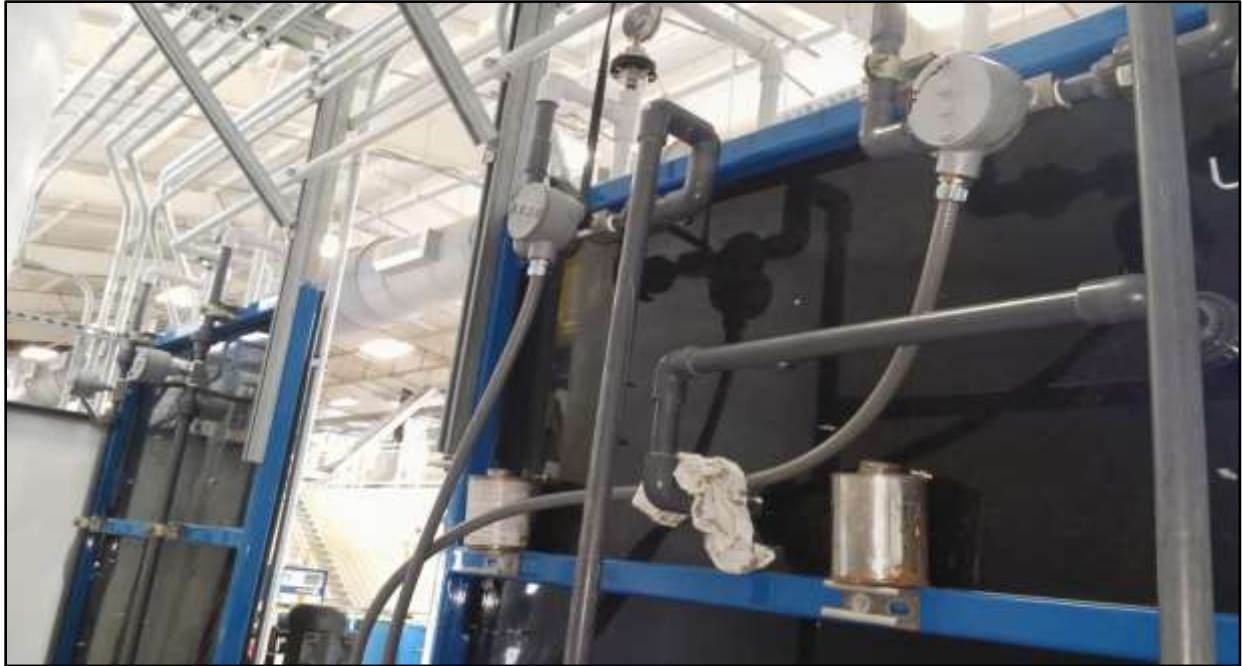
San Luis Demonstration Treatment Plant The modified piping at the nutrient feed pumps
