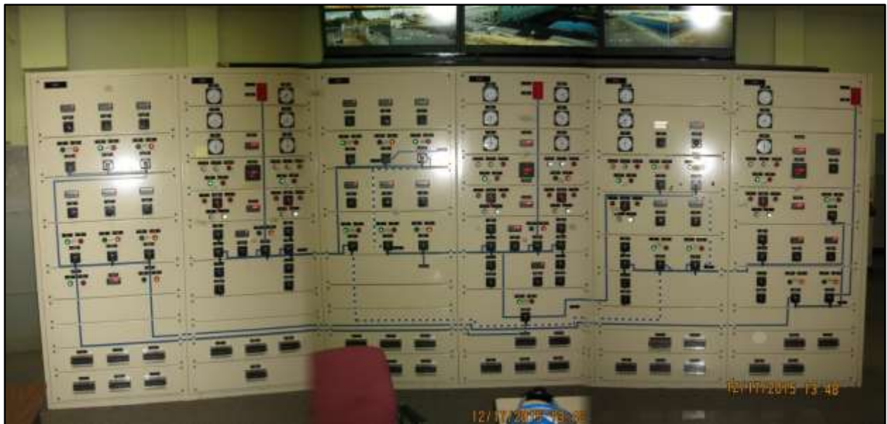
Tracy 13.8 kV Switchgear/Breaker Replacement Control Panels CCA1 through 6F with mimic board installed
