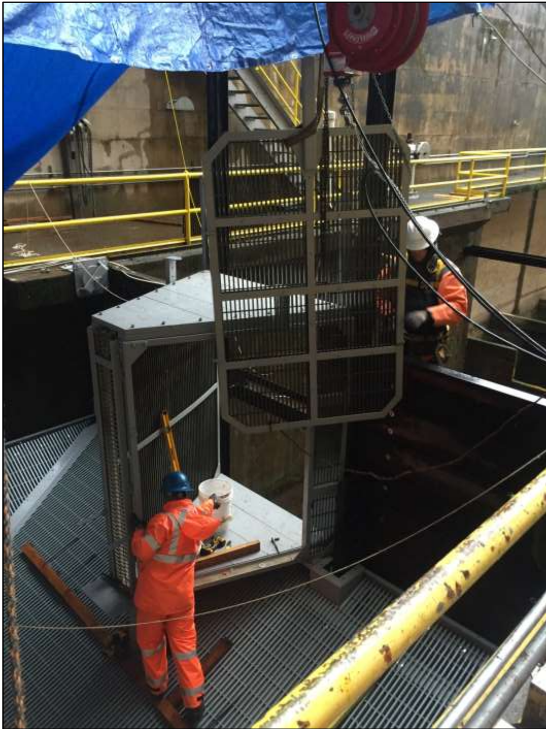
Keswick Fish Trap Brail Replacement Subcontractor Abacus Installing the Escape Door onto the Fish Trap Brail Entrance Structure.
