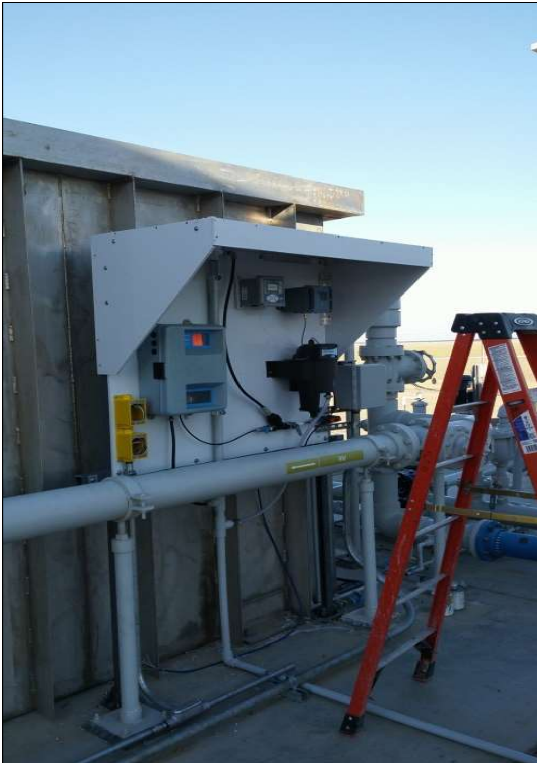
San Luis Demonstration Treatment Plant Installation of new Chlorine, Turbidimeter, and pH/Temperature instruments for Mod 0013 at the pretreatment area
