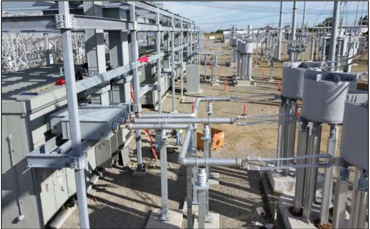
Tracy 13.8 kV Switchgear/Breaker Replacement Overview of work site on the south side of the switchgear buildings, showing current limiting reactors, with building 6A in the foreground
