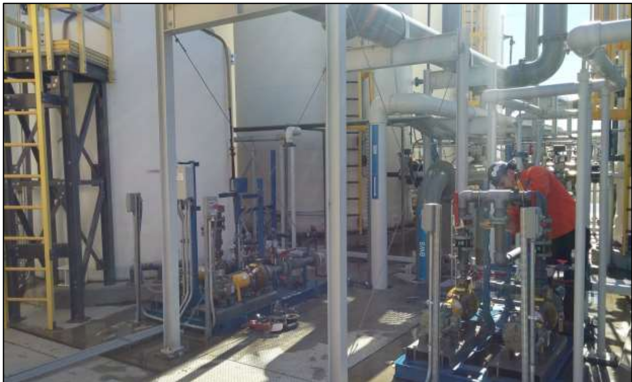
San Luis Demonstration Treatment Plant Removal and replacement of the ABMet First and Second Stage Feed piping
