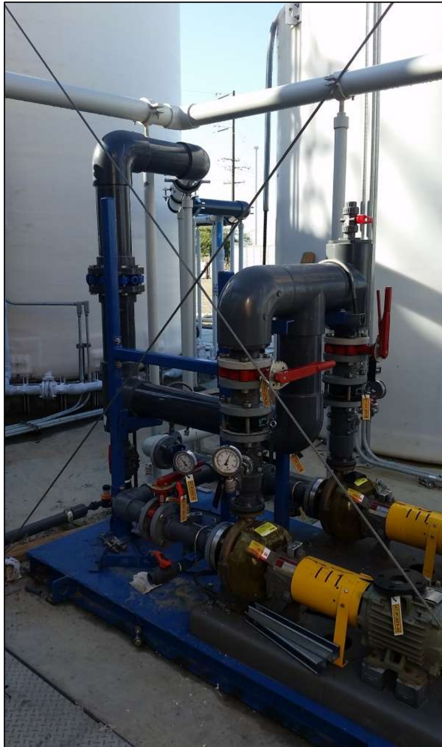
San Luis Demonstration Treatment Plant Completed ABMet Second Stage pump discharge feed piping
