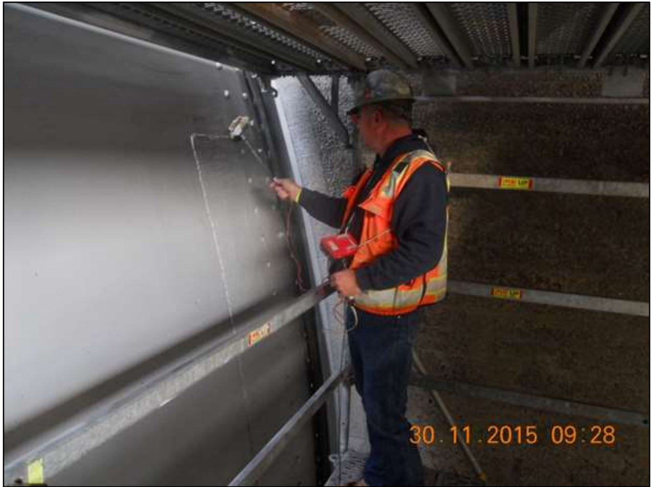
Nimbus Dam Radial Gate Repairs, Phase III FD Thomas foreman performing a discontinuity test on the coatings on the upstream side of Gate 18
