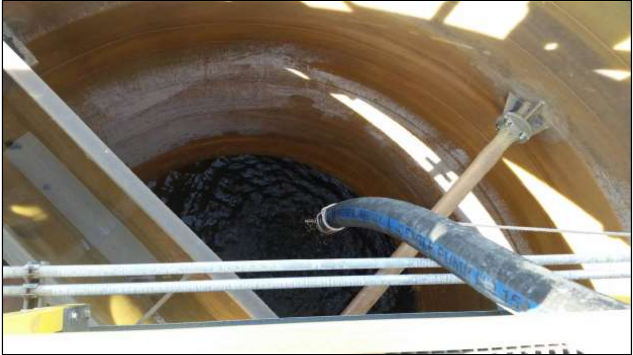
San Luis Demonstration Treatment Plant Installation of the new coconut based granulated activated carbon in the ABMet First Stage bioreactor tanks
