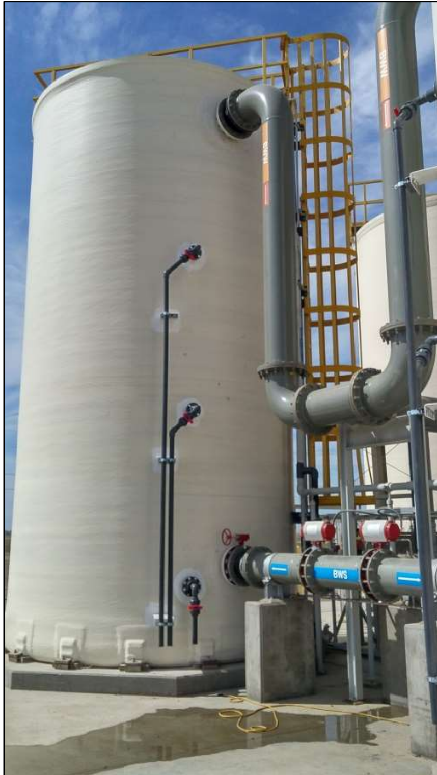
San Luis Demonstration Treatment Plant Sample tap piping installed on ABMet Second Stage bioreactor tank
