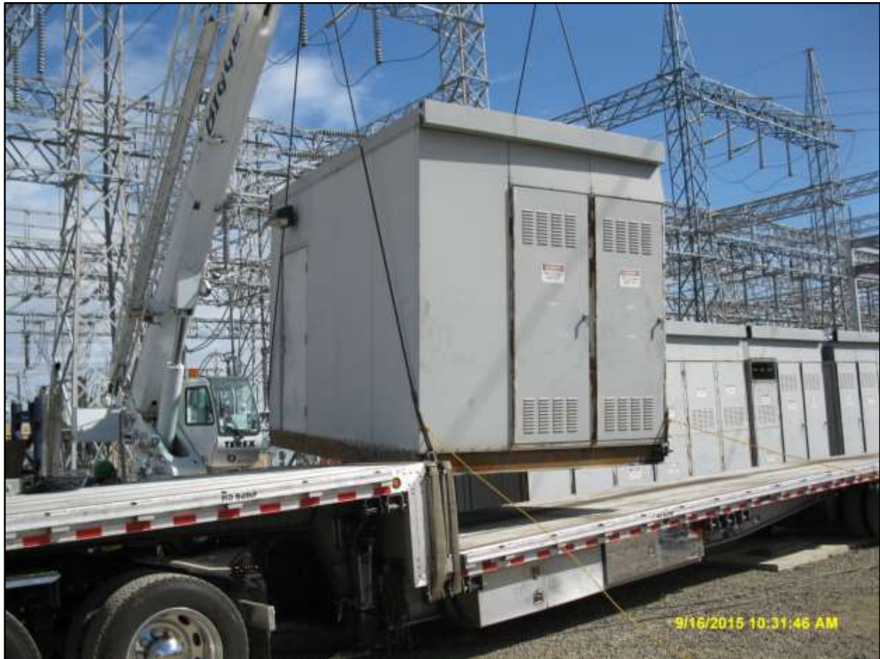
Tracy 13.8kV Switchgear/Breaker Replacement Removal of old switchgear building
