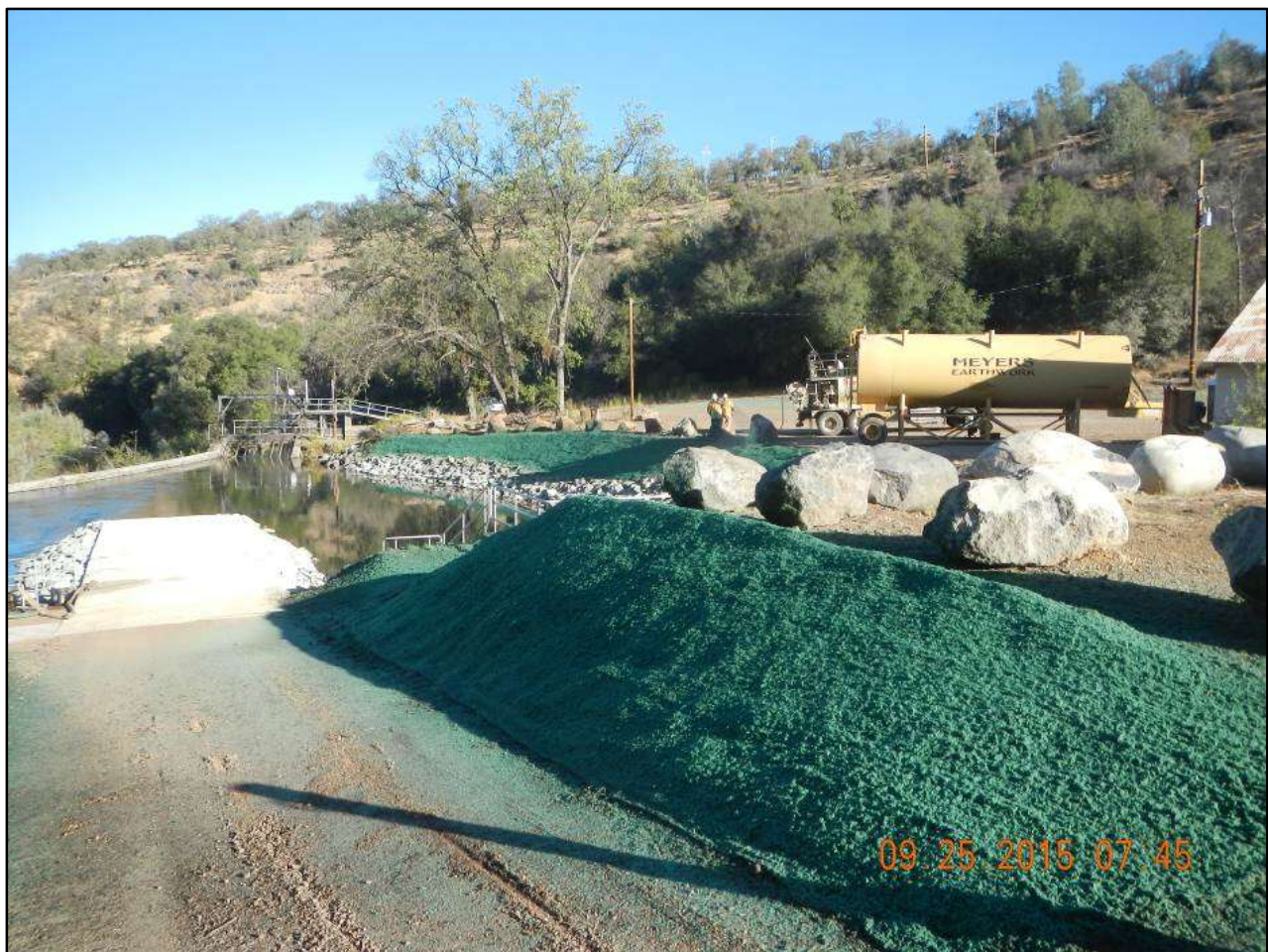
Safety and Facility Access Improvements - Battle Creek Salmon and Steelhead Restoration Seeding near the access ramp into Coleman Canal
