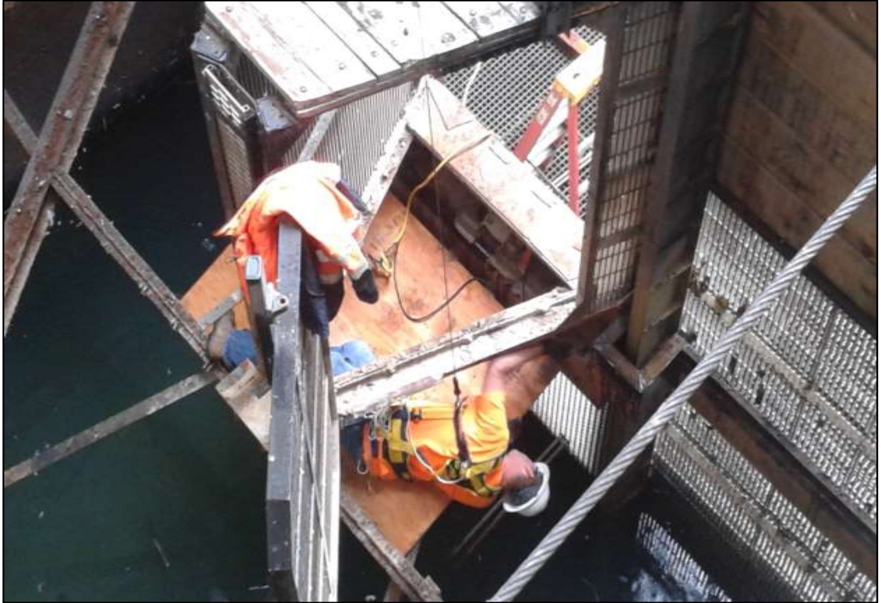
Keswick Fish Trap Brail Replacement Cutting mounts for the telescoping gate below the Brail Inlet
