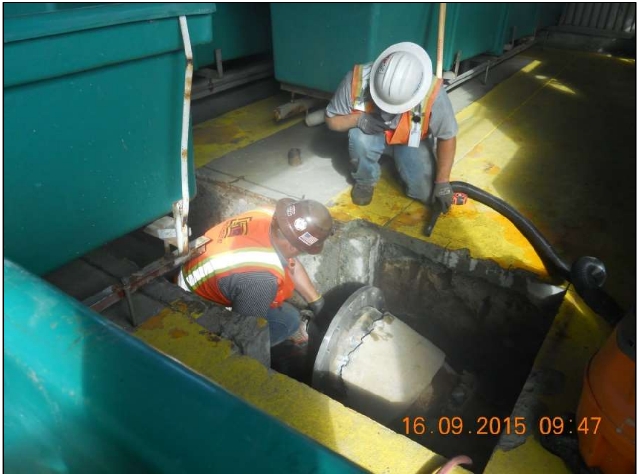
Nimbus 16-inch Pipeline Replacement Workers cut away the returns on the existing concrete troughs to allow installation of new valve operators.
