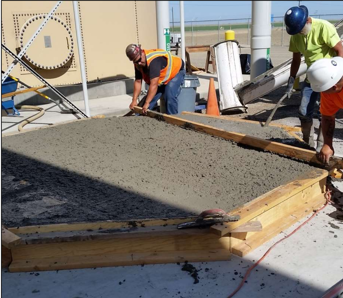
San Luis Demonstration Treatment Plant Concrete placement of the equipment pad for the new ABMet tank
