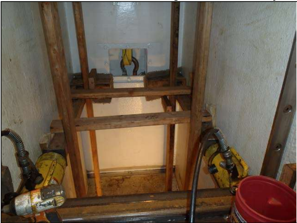
Prosser Creek Dam Refurbish High-Pressure Gate Seats and Regulating Gates Hydraulic jacks were used to apply force to check the gate leaf and frame seat bars clearance
