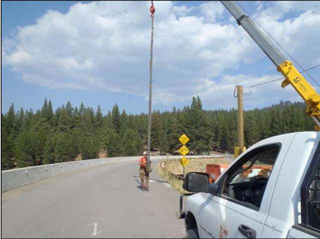
Prosser Creek Dam Refurbish High-Pressure Gate Seats and Regulating Gates The hydraulic oil lines were removed from the gate chamber to modify them.
