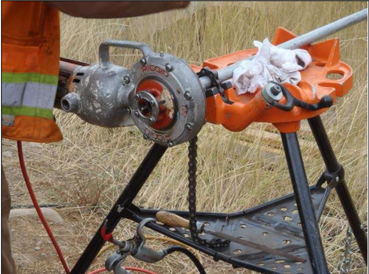
Prosser Creek Dam Refurbish High-Pressure Gate Seats and Regulating Gates Threading pipe for the hydraulic pipe connections to the bypass valve installation
