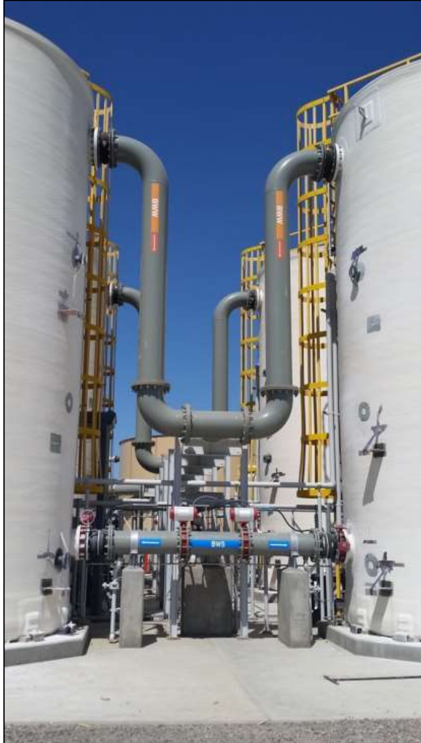
San Luis Demonstration Treatment Plant Sample taps installed on ABMet Second Stage bioreactor tanks
