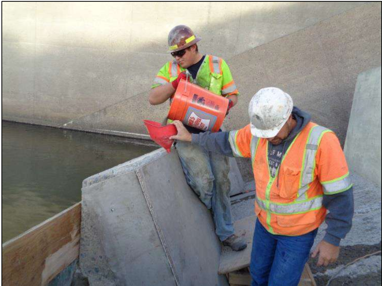
Marble Bluff Dam Spillway Repair Grout being poured to fill the void between the dentate and the stainless steel plate
