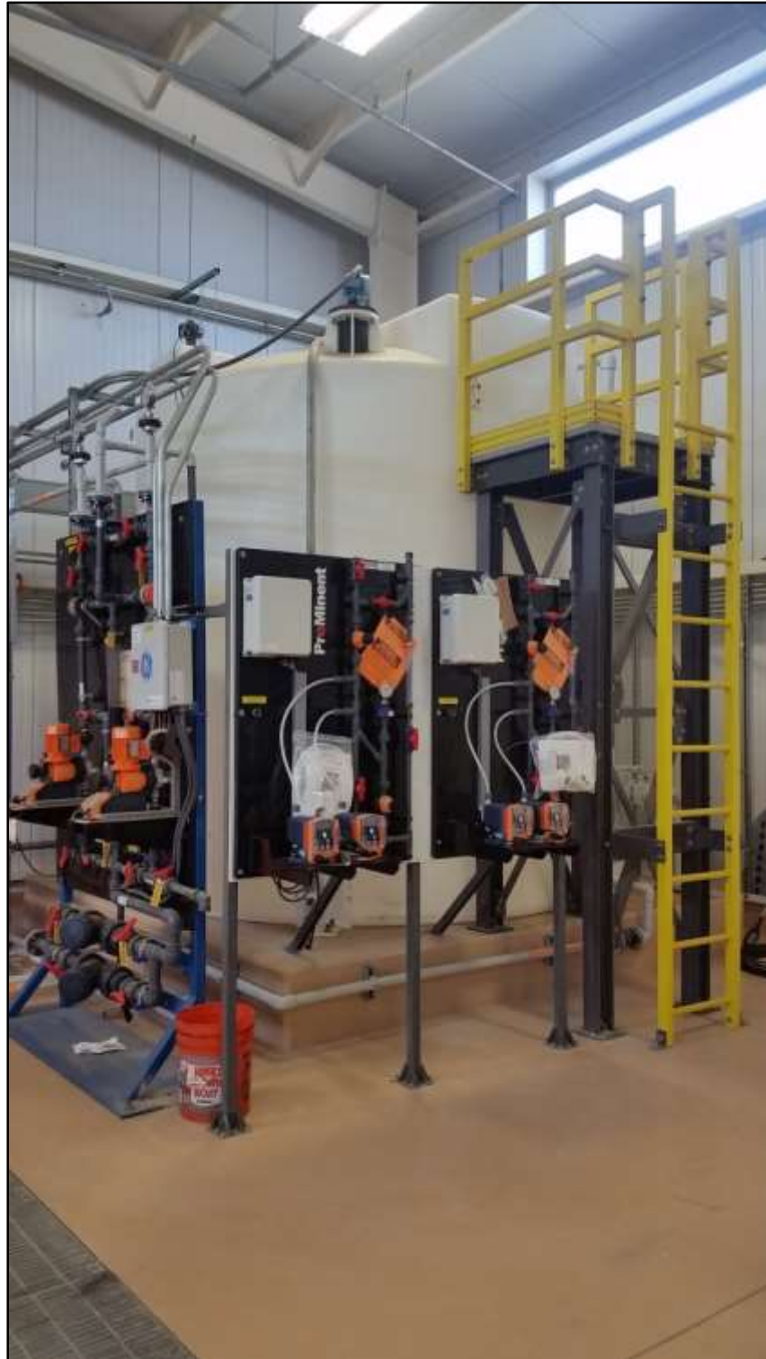
San Luis Demonstration Treatment Plant Installation of two new antiscalant skids to feed the ABMet First and Second Stage bioreactor tanks
