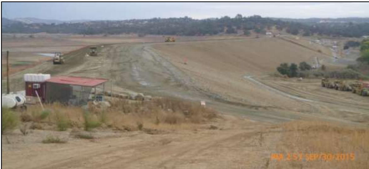
Mormon Island Auxiliary Dam Overlay Overview of the cobble slope placement and gravel surfacing work.
