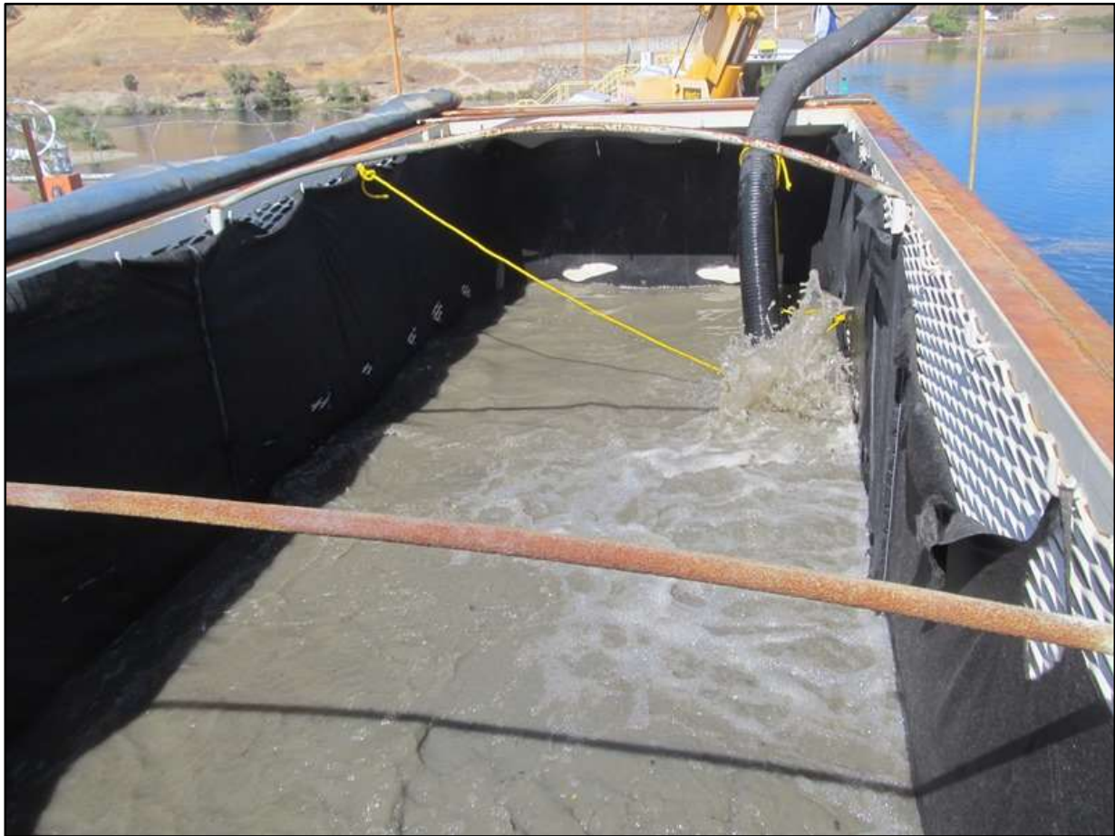
Nimbus Dam Radial Gate Repairs, Phase III Filling dredging material container
