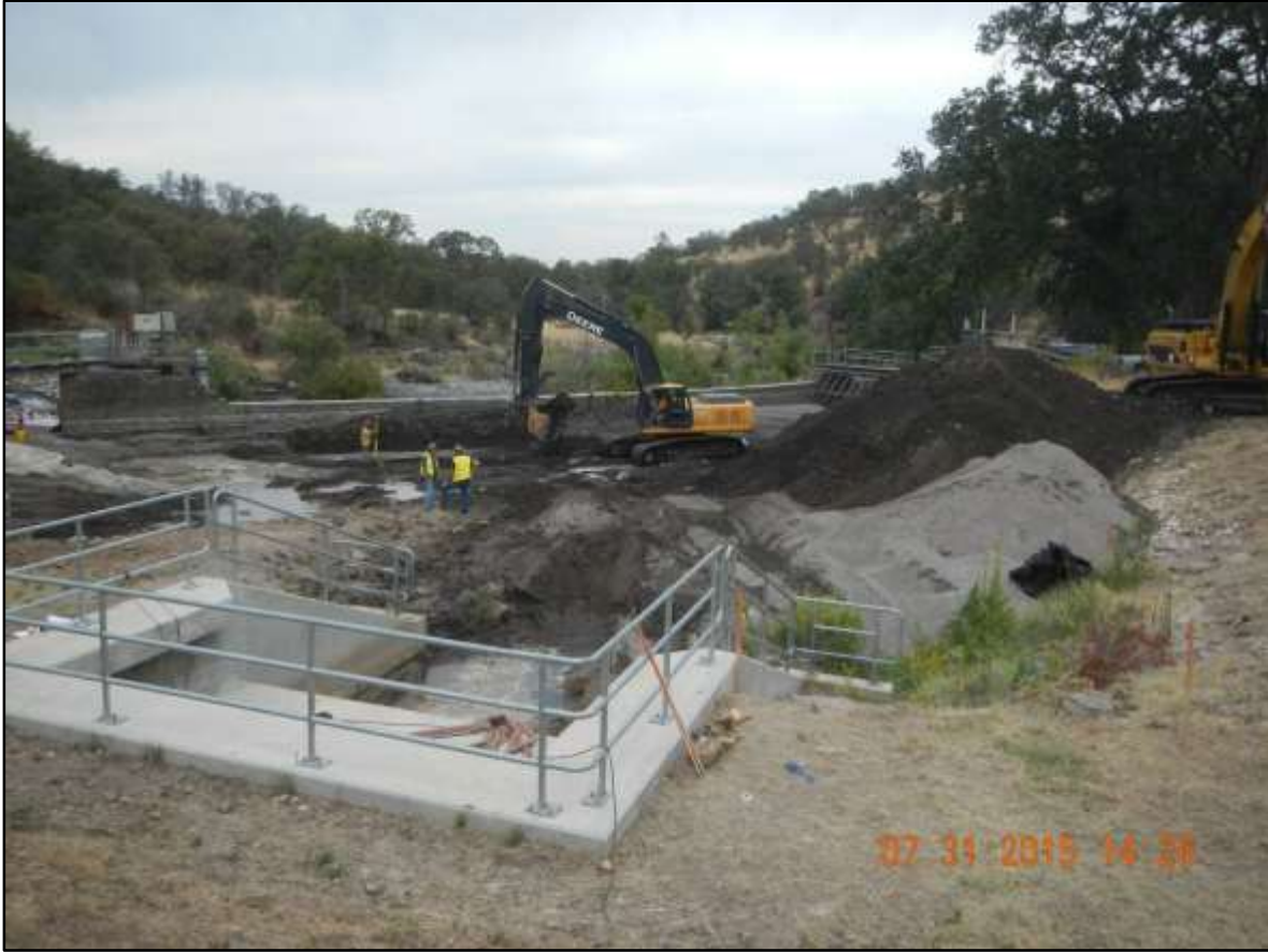
Battle Creek Salmon and Steelhead restoration project – Safety and Facility Access Improvements JD 350 excavator feeding material to the CAT 345 that is loading material for off haul.
