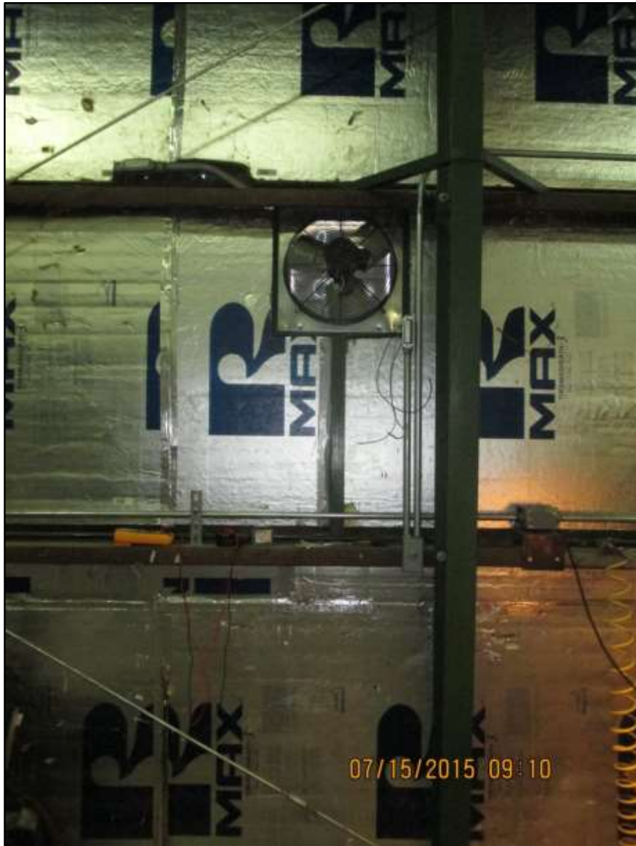
Tracy P&H Building Temporary Retrofit Exhaust fan that was installed on west wall of building was completed
