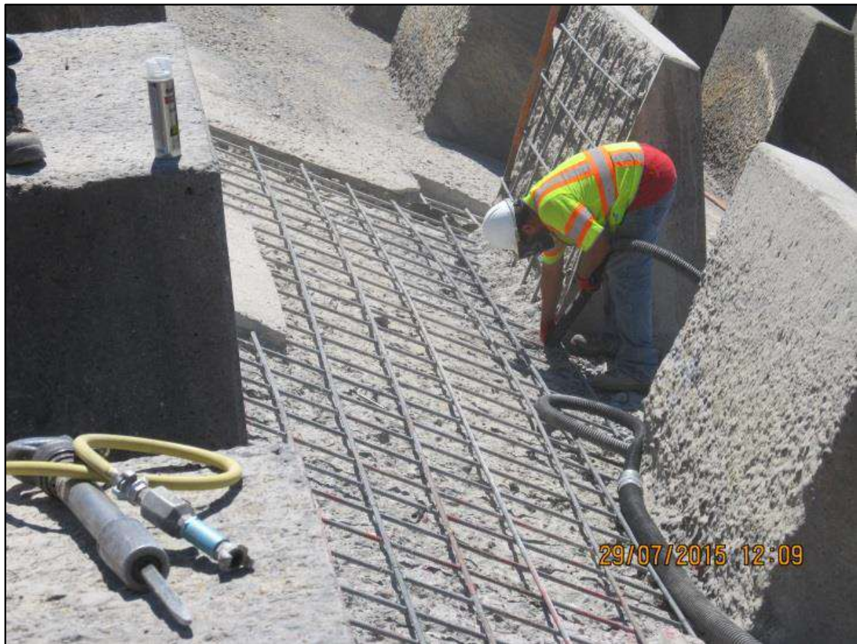
Marble Bluff Dam Spillway Repair Area of apron from which concrete has been removed
