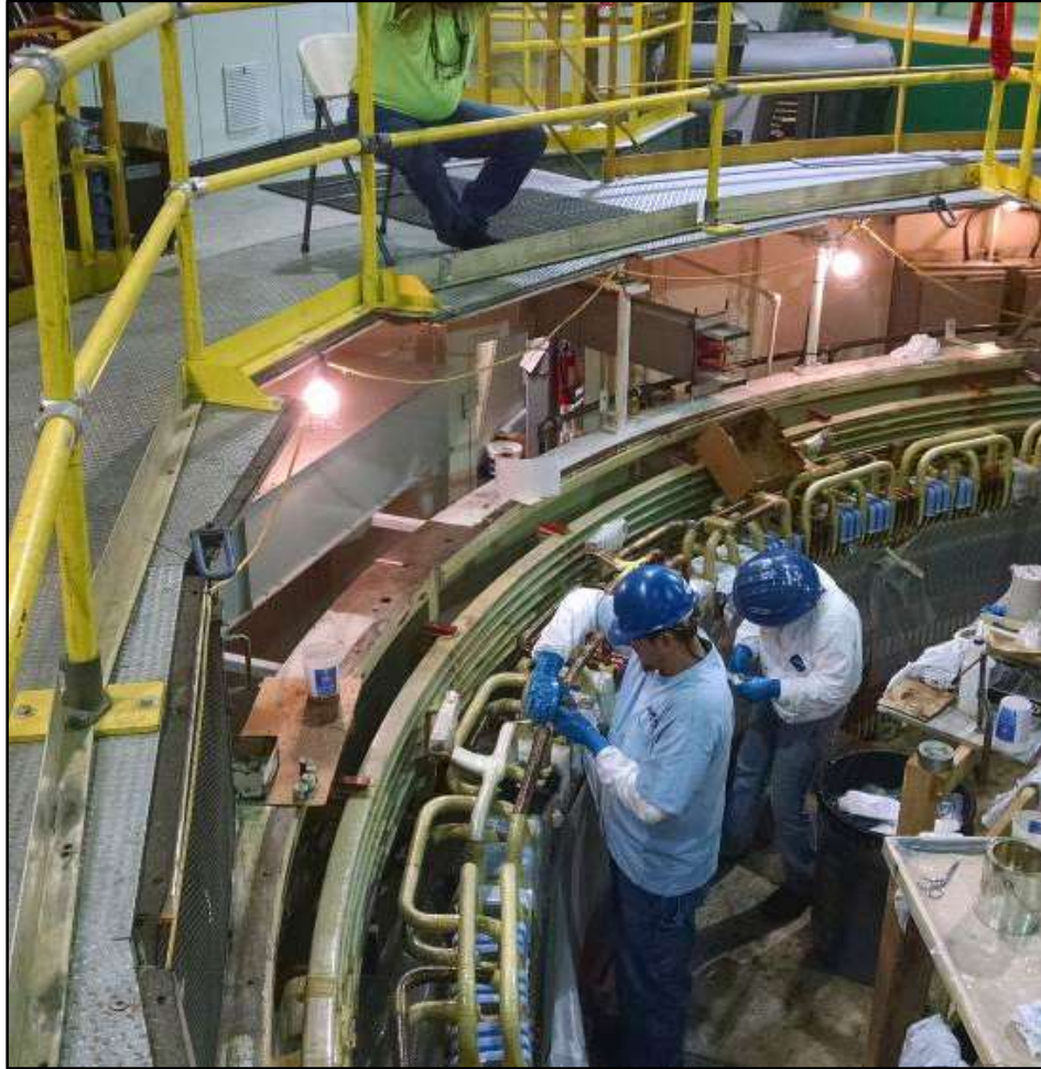
Folsom Power Plant Generators U1, U2, and U3 Rewind and Excitation System Replacement Andritz Hydro insulating group jumpers
