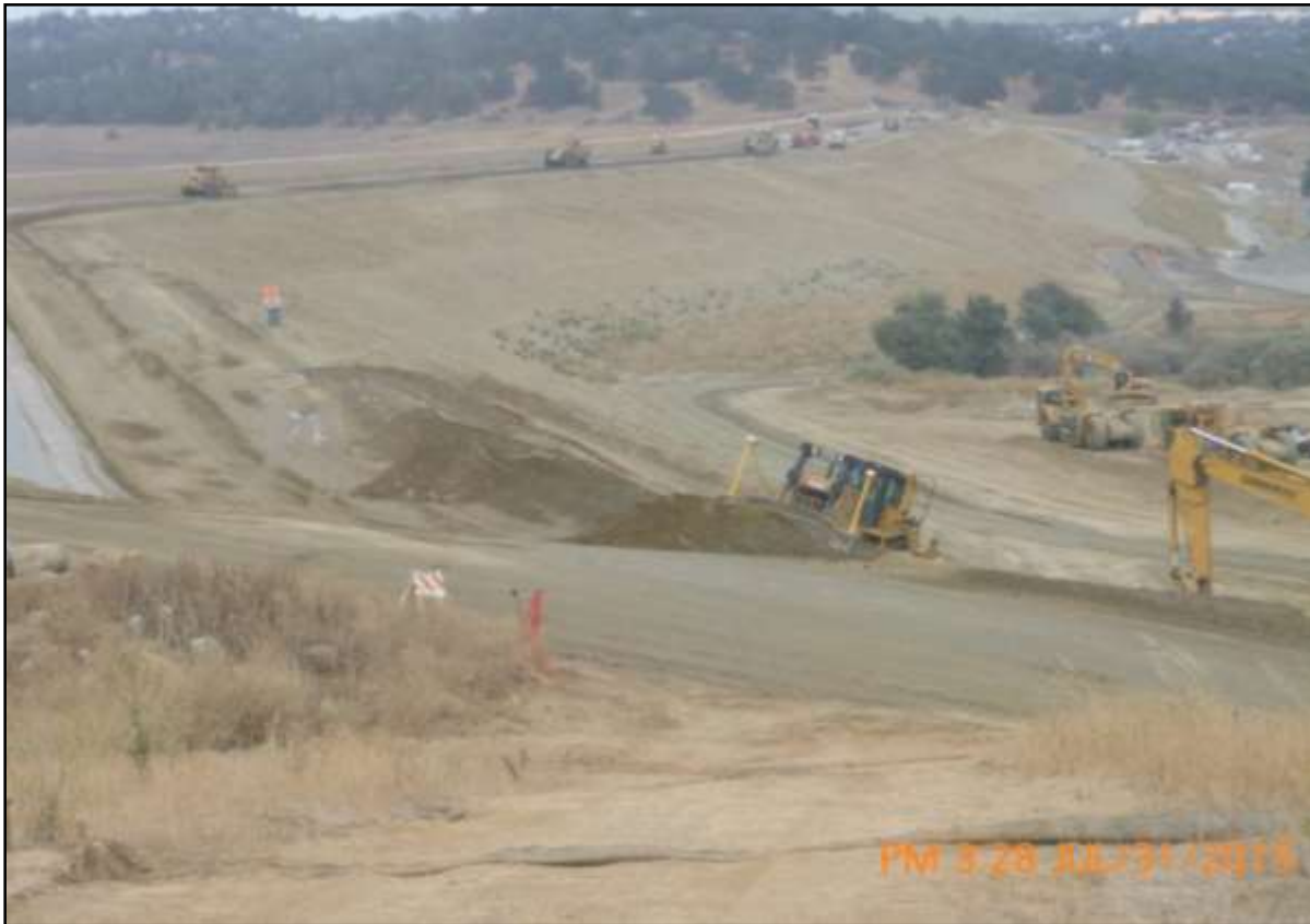
Mormon Island Auxiliary Dam Overlay View of the vertical chimney and embankment at elevation 476 feet
