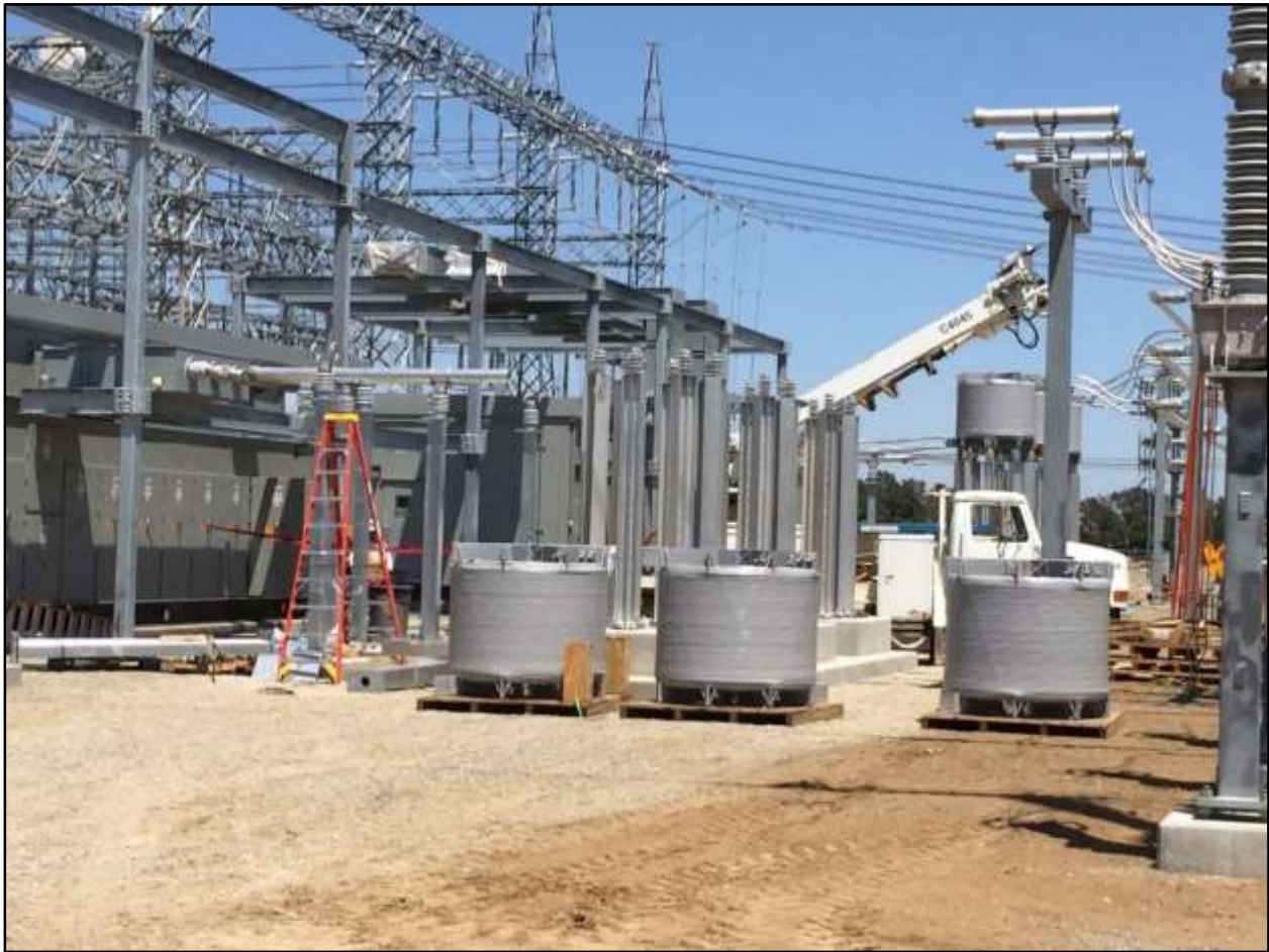
Tracy 13.8kV Switchgear/Breaker Replacement, Tracy Pumping Plant and Substation Building 8A being installed along with reactor columns, bushing box and 6-inch tubular bus
