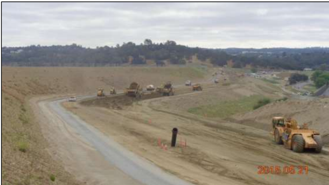
Mormon Island Auxiliary Dam Overlay View of the dam and chimney at elevation 445 feet.
