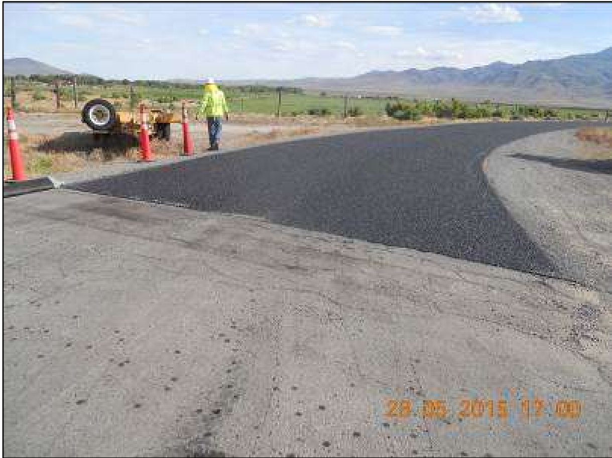
Marble Bluff Dam Asphalt Pavement Rehabilitation Chip Seal after application by subcontractors Statewide Construction Sweeping, Harco Trucking, Talley Oil, and Kustom Koatings
