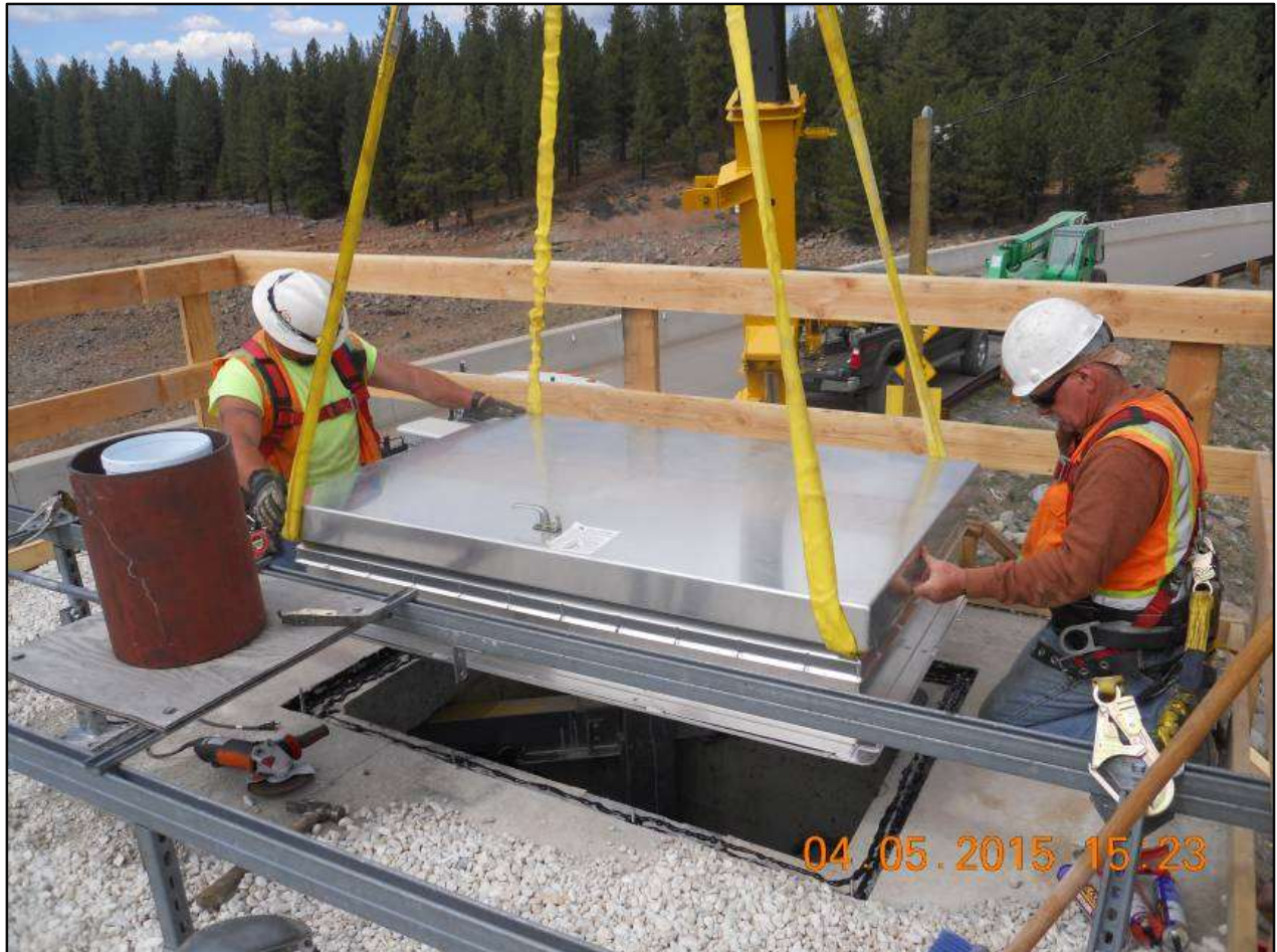
Prosser Creek Dam Refurbish High-Pressure Gate Seats and Regulating Gates Installation of the Bilco Hatch on the roof of the Gate Chamber building by Knight Construction workers
