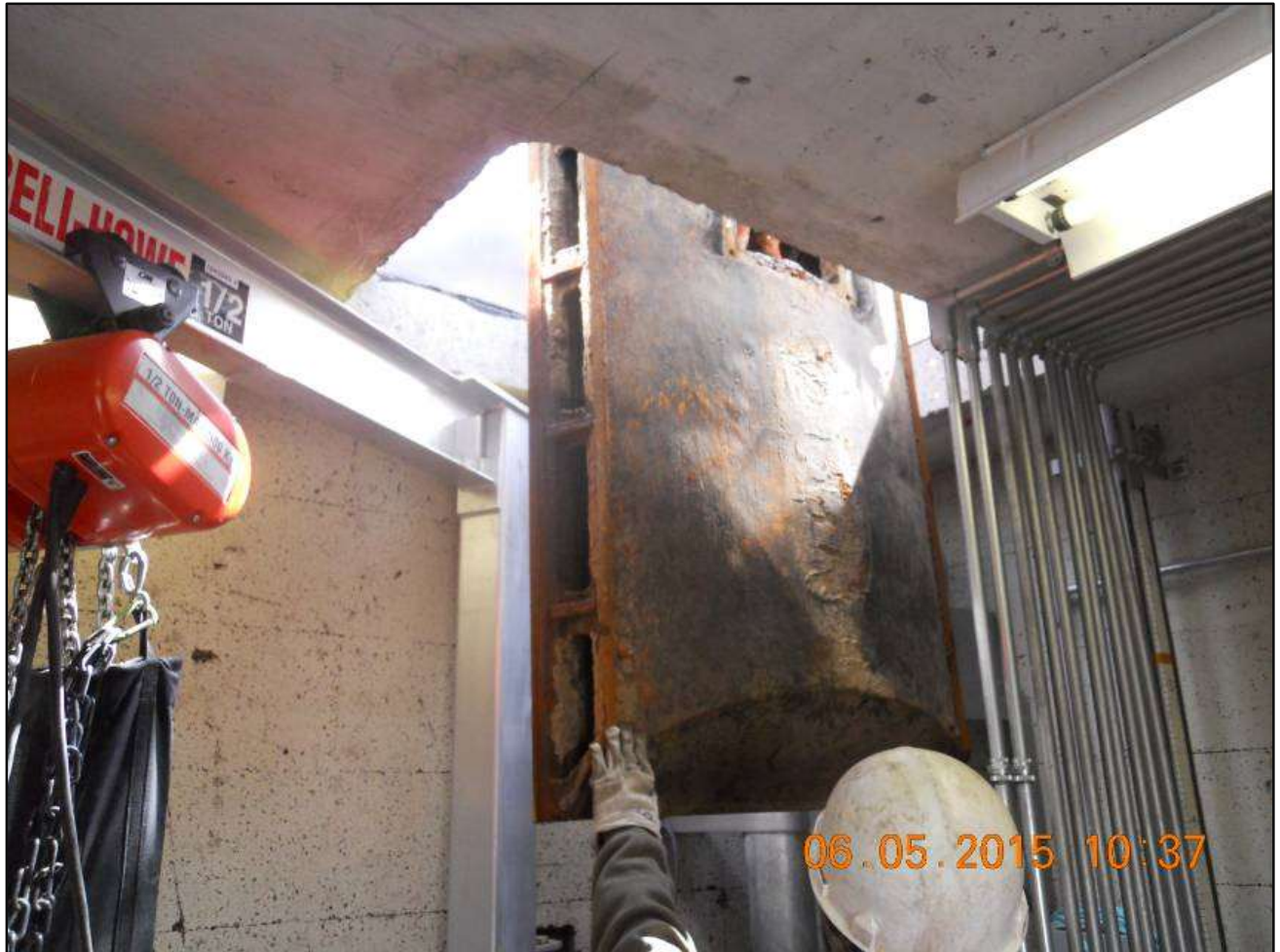
Prosser Creek Dam Refurbish High-Pressure Gate Seats and Regulating Gates Removal of the Gate 3 leaf through the Bilco Hatch by contractors
