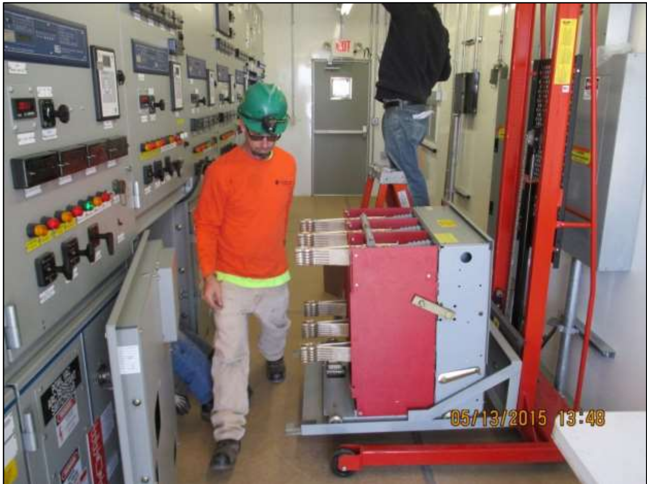
Tracy 13.8kV Switchgear/Breaker Replacement Tracy Pumping Plant and Substation Contractor Contra Costa Electric Begins Preparation for Release of Building 11A to Bureau of Reclamation for Operations
