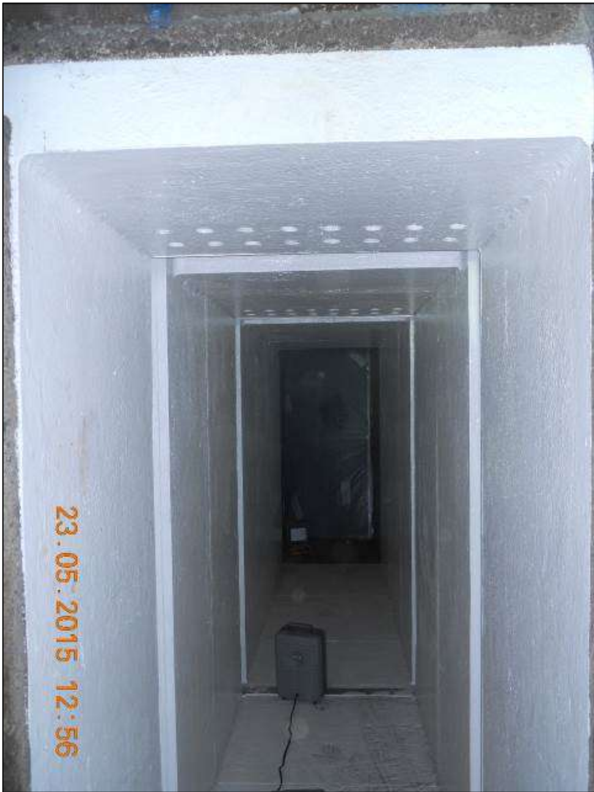
Prosser Creek Dam Refurbish High-Pressure Gate Seats and Regulating Gates The first coat of 6 to 8 mil. thick Macropoxy 646 applied to the frames for gates 3 and 4 by contractor
