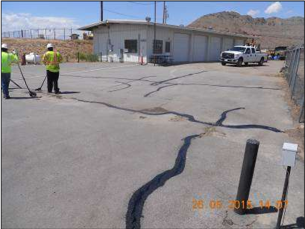
Marble Bluff Dam Asphalt Pavement Rehabilitation Rubberized Crack Seal being applied by contractor
