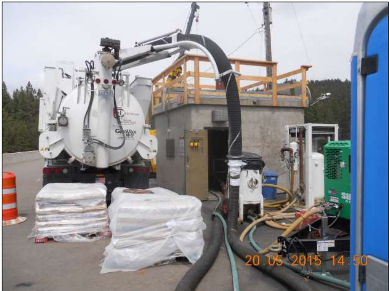
Prosser Creek Dam Refurbish High-Pressure Gate Seats and Regulating Gates A vacuum truck ready to remove blast media from the gate chamber
