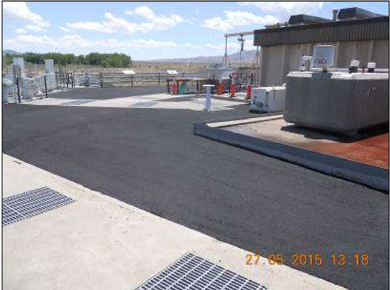
Marble Bluff Dam Asphalt Pavement Rehabilitation Slurry Seal after application by contractor
