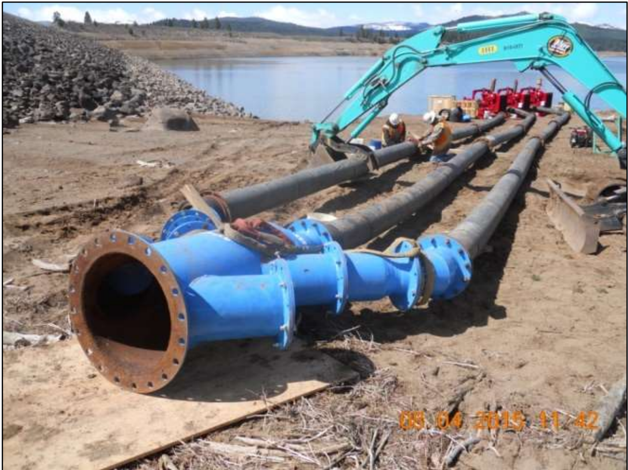
Prosser Creek Dam Refurbish High-Pressure Gate Seats and Regulating Gates Knight Construction completes the installation of the three 12-inch pump lines to the manifold from the pumps.
