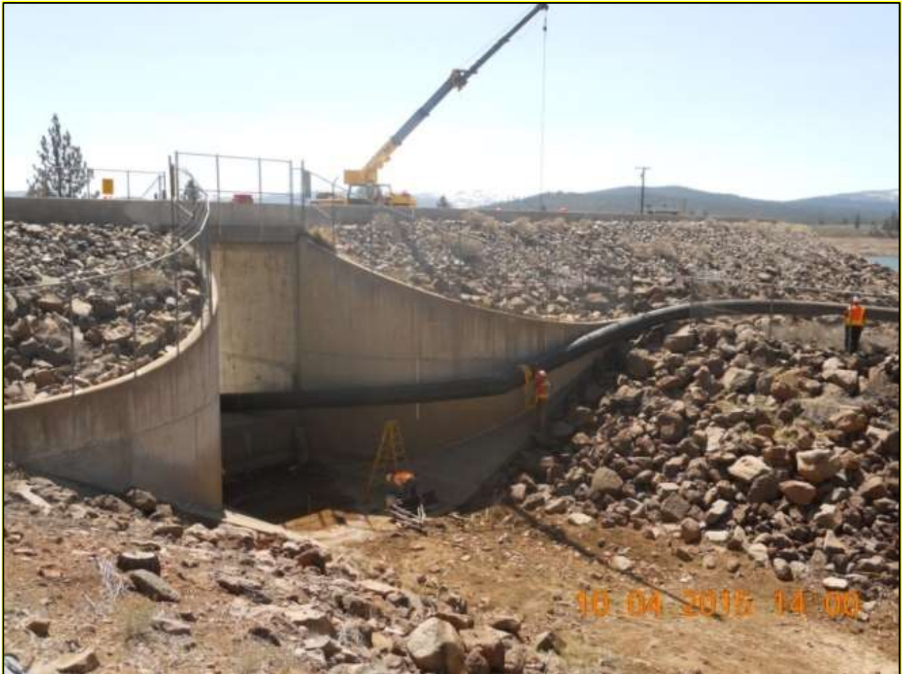
Prosser Creek Dam Refurbish High-Pressure Gate Seats and Regulating Gates Installation of the 24-inch HDPE pipe from the diesel pumps to Prosser Dams Spillway.
