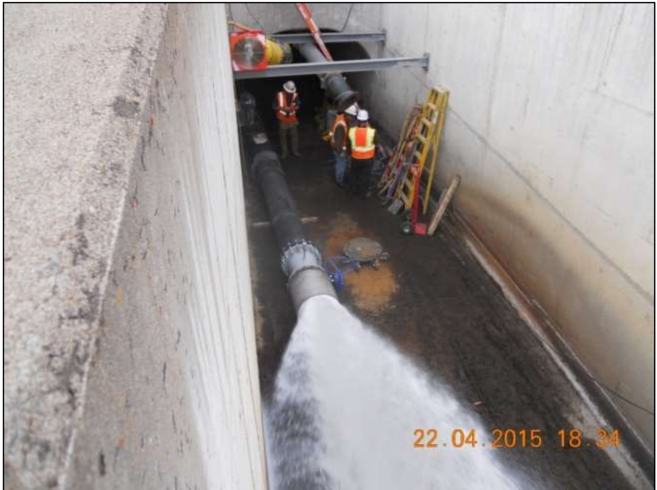
Prosser Creek Dam Refurbish High-Pressure Gate Seats and Regulating Gates The Downstream valve is opened on the bypass system to begin delivering water to the Truckee River.
