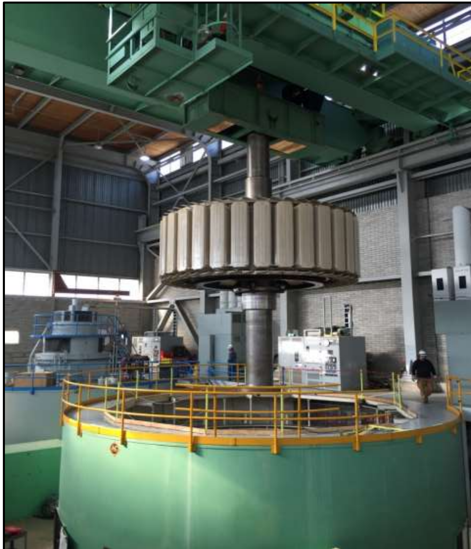
Spring Creek Powerplant Generators G1 and G2 Rewind, Spring Creek Powerplant - Bureau of Reclamation Staff reassembling Unit 2
