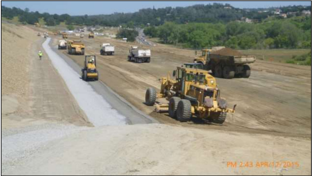
Mormon Dam Auxiliary Dam Overlay Scrapers placing Zone B material at the chimney from station 434+00 to station 458+00, while the motor grader and 20-ton roller spread and compact each lift.
