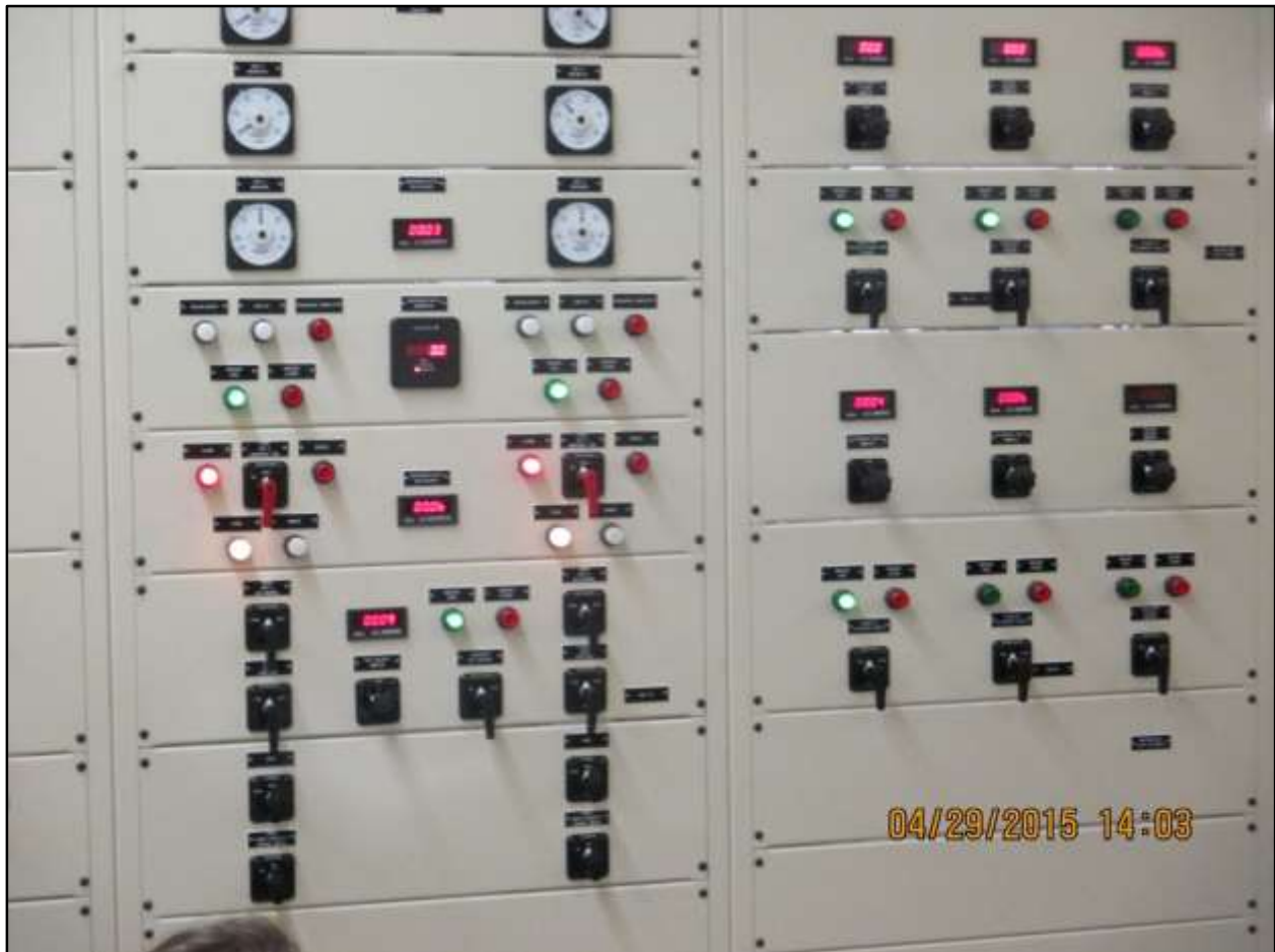
Tracy 13.8kV Switchgear/Breaker Replacement Control panel CCA2F and CCA3F during function testing of pumps #2 and #6 and the Tie breakers showing indicating lights operational
