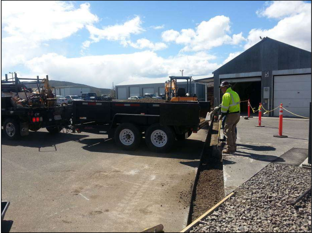
Klamath Basin Area Office Pivot Gate System Nomlaki crew placing the aggregate base material on the electrical trench in preparation for the paving operation.
