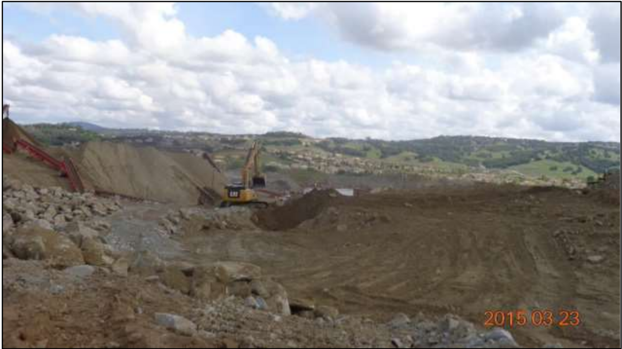
Mormon Island Auxiliary Dam Overlay Fisher Industries loading grizzly screen that is Producing Zone A and B materials for stockpile
