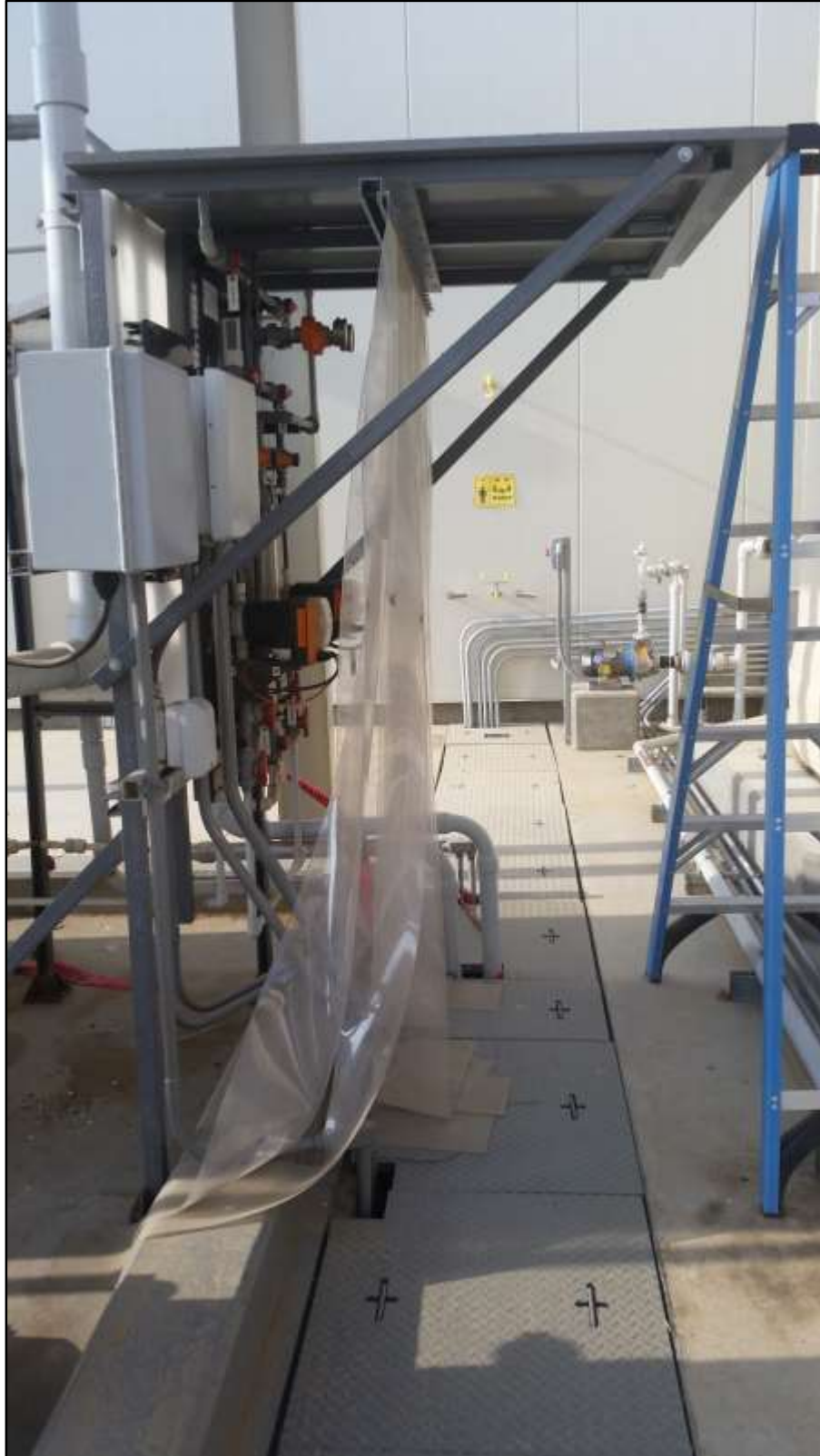
San Luis Demonstration Treatment Plant Coating operations and the installed HCl curtain at the HCl containment area
