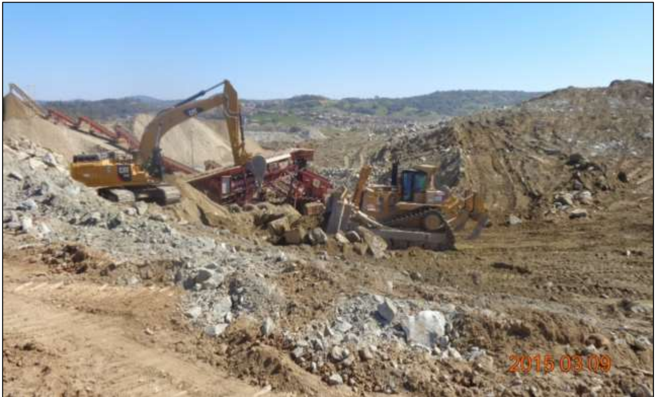
Mormon Island Auxiliary Dam Overlay - Sub-contractor operating grizzly screen with a Cat 349 excavator and Cat D10 dozer producing stockpile of Zone A and B material
