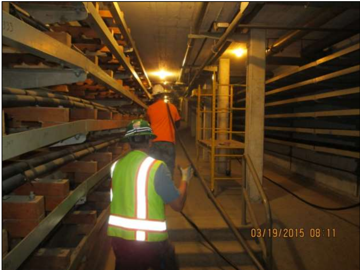
Tracy 13.8kV Switchgear/Breaker Replacement at Tracy Pumping Plant and Substation Electricians pulling control cables in 13.8kV tunnel section
