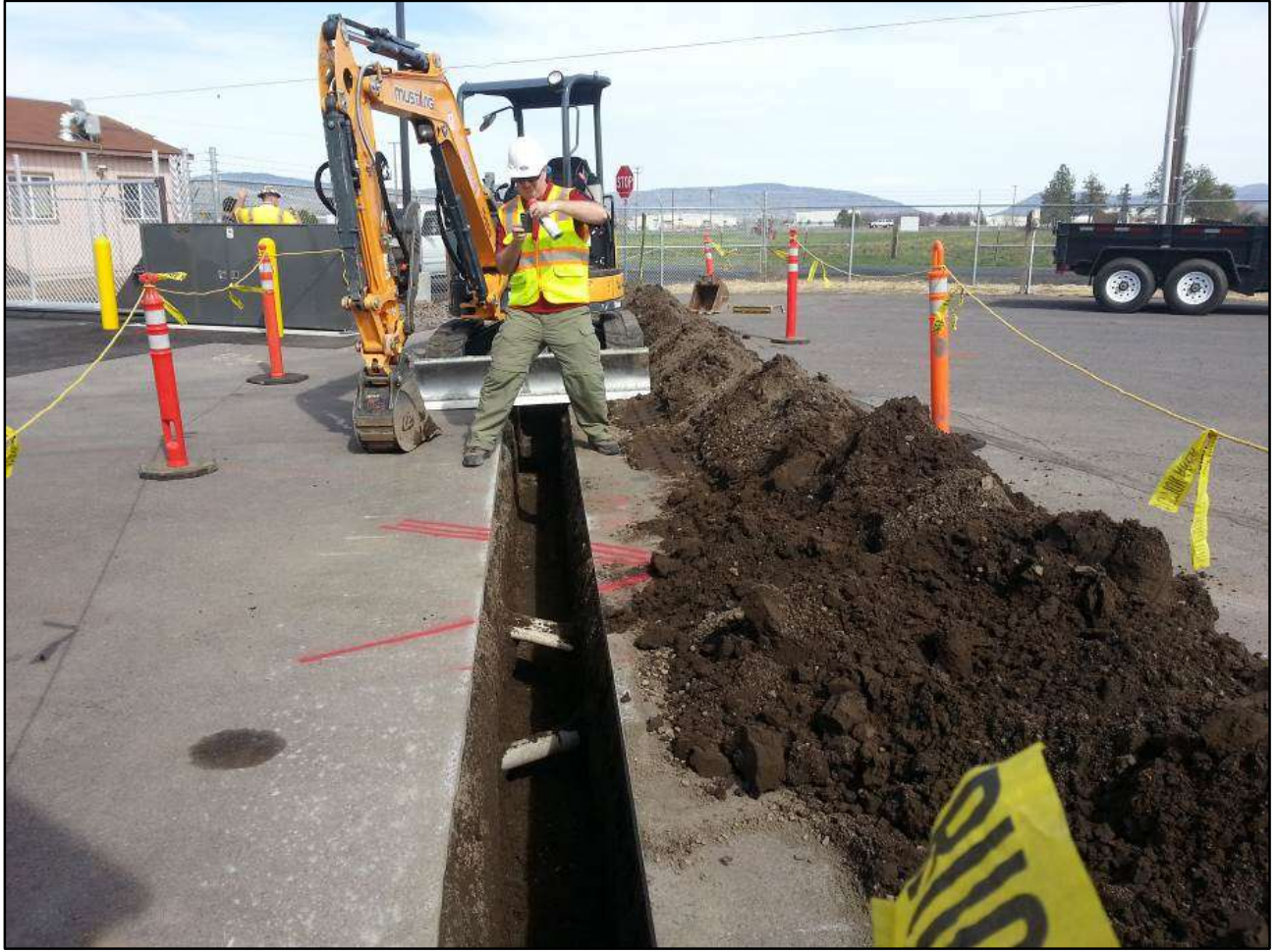
Klamath Basin Area Office Pivot Gate System View of the electrical trench and the communication and power conduits encountered during the excavation
