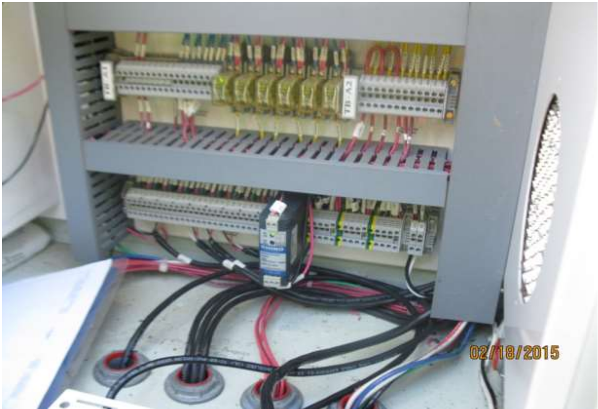
North Fork Screens and Ladders Gate Modulations. North Battle Creek Feeder Dam 24-volt DC power supply installed in Panel California.
