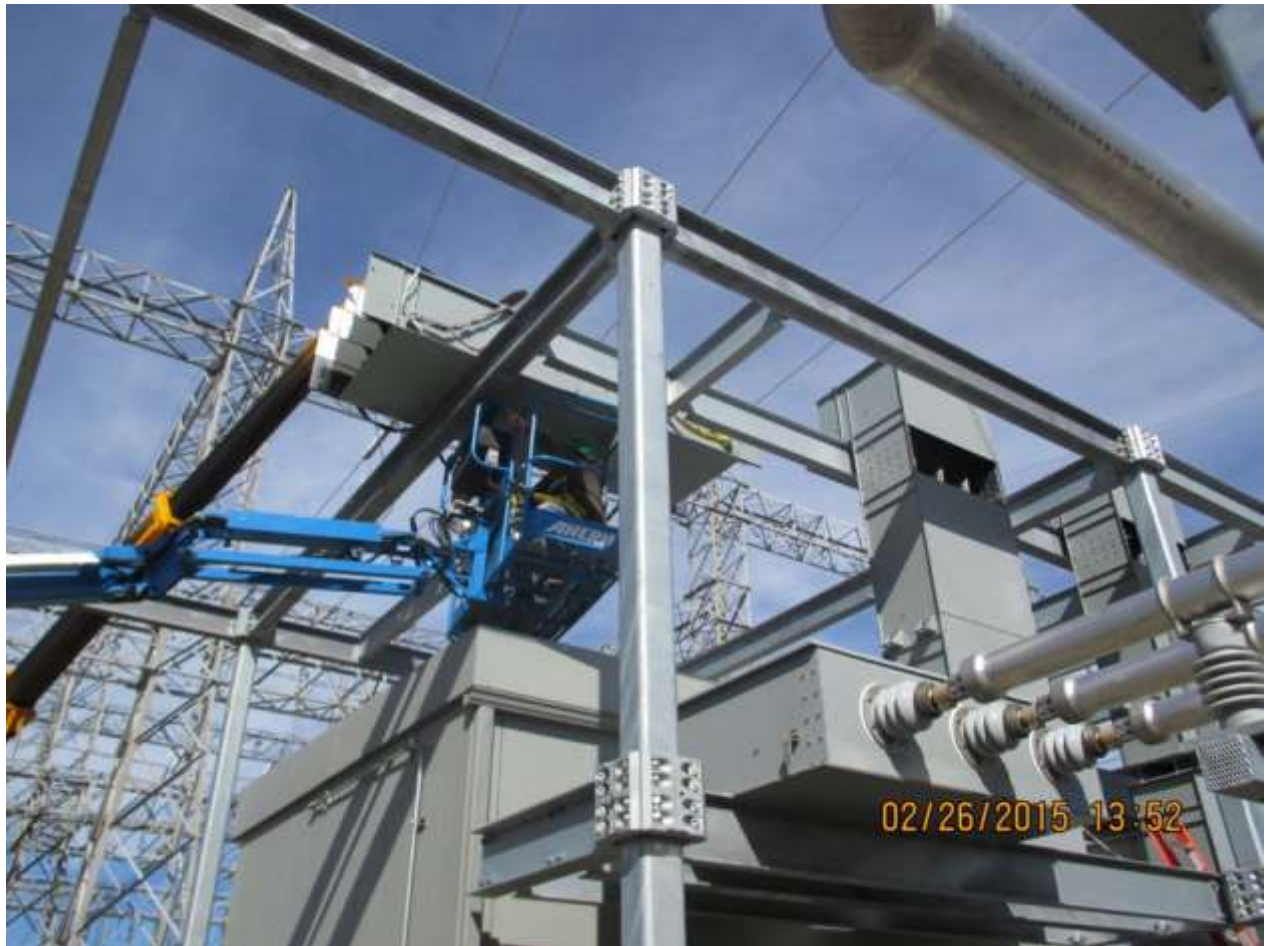
Tracy 13.8kV Switchgear/Breaker Replacement at Tracy Pumping Plant and Substation Installation of the nonsegregated bus duct over top of building 11A
