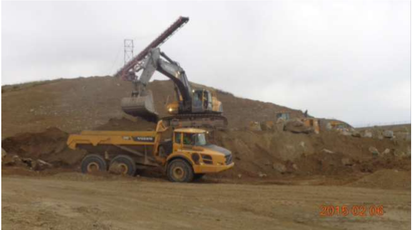
Mormon Dam Auxiliary Dam Overlay. Fisher Industries haul truck being loaded by. The Cat excavator with material for the crushing plant
