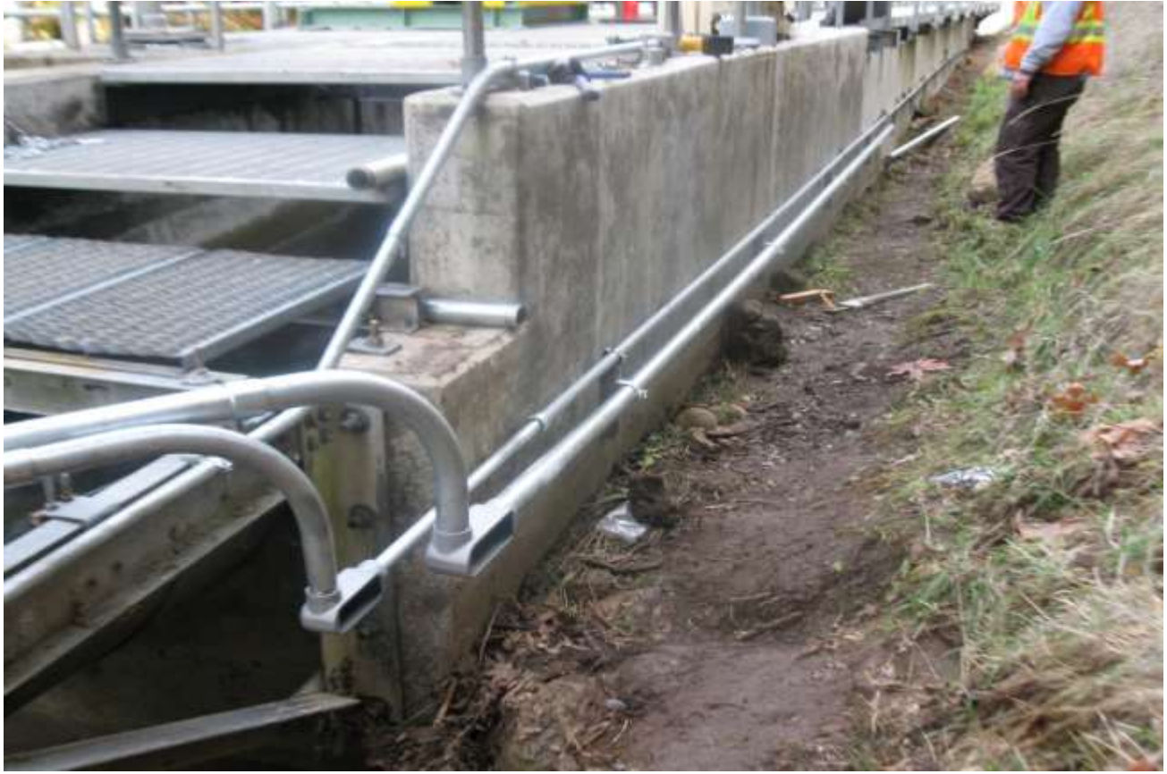
Battle Creek Salmon and Steelhead North Fork Screens and Ladders Gate Modulations Installing new 2" conduit, for power, below existing 1" conduit which will be used for analog.
