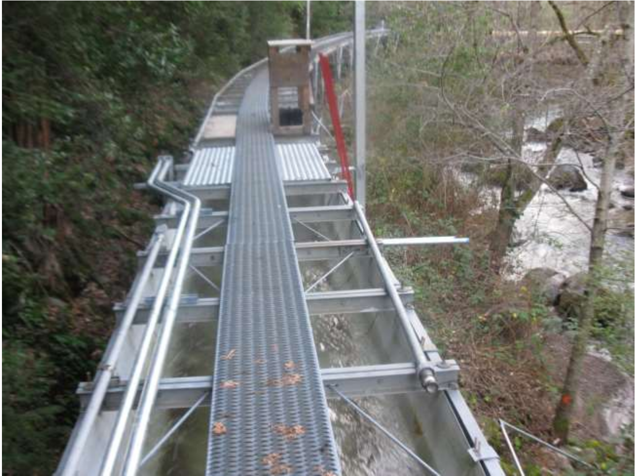
Battle Creek Salmon and Steelhead North Fork Screens and Ladders Gate Modulations Conduit installed at new sensor location (Looking downstream).
