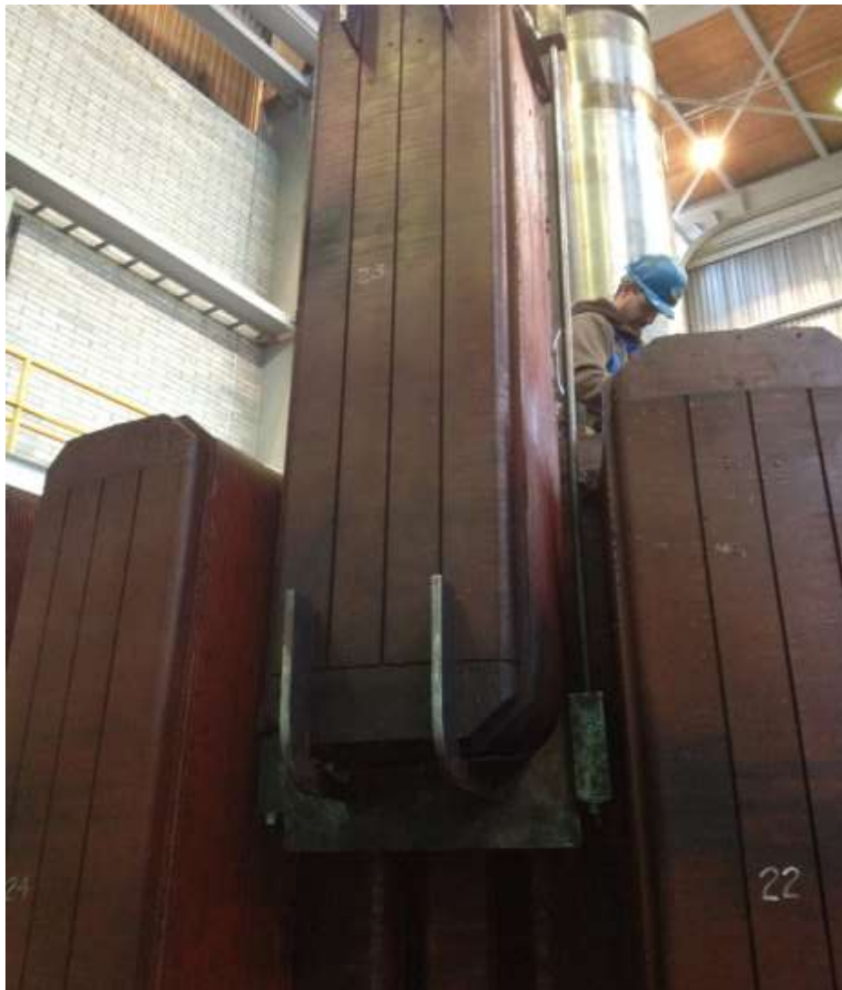
Spring Creek Powerplant Generators G1 and G2 Rewind Unit 2 rotor pole removal being performed by contractor
