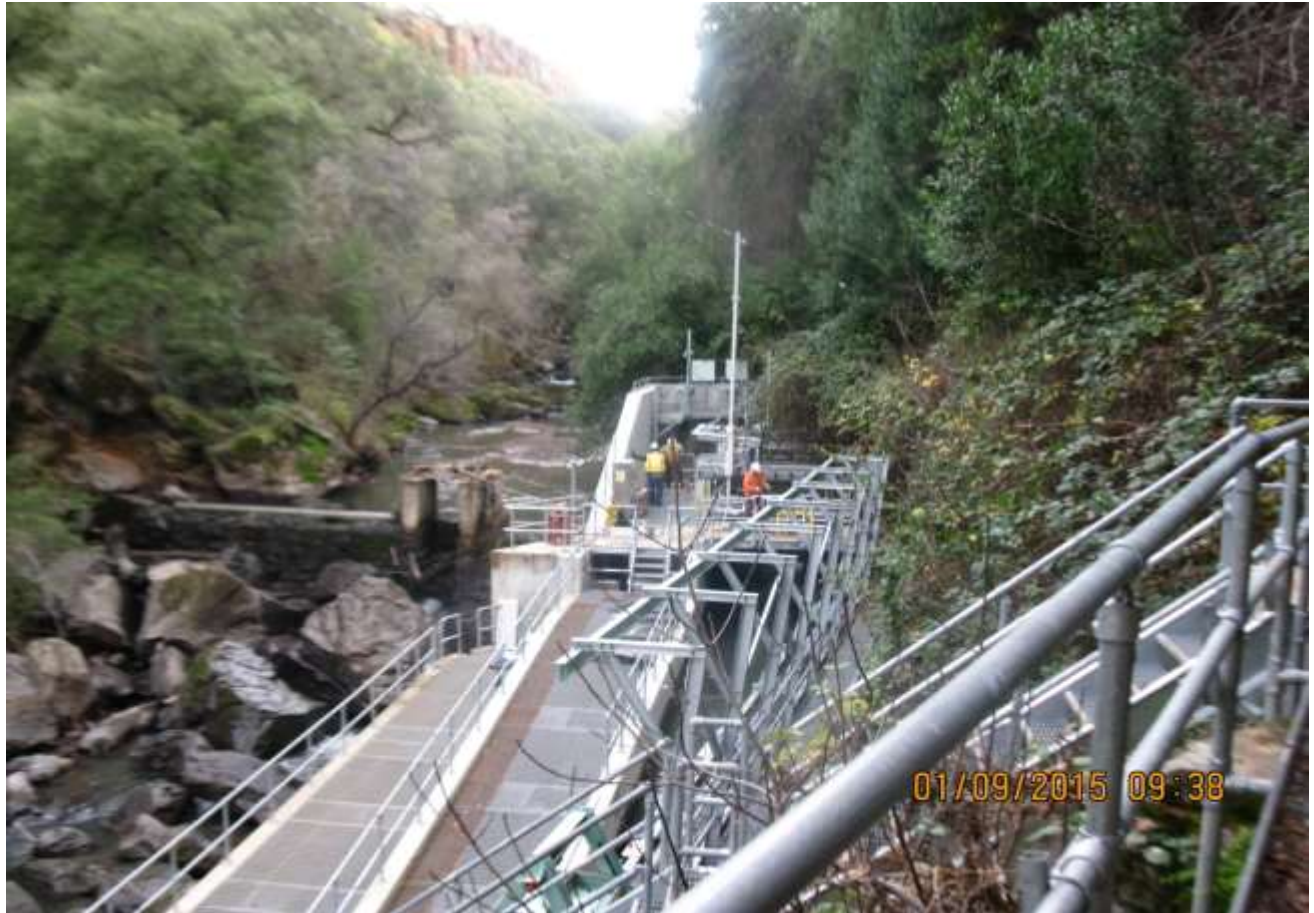
Battle Creek Salmon and Steelhead North Fork Screens and Ladders Gate Modulations Start of installing conduits at Eagle Canyon Dam during a scheduled outage of electrical power and during a scheduled clearance to be working inside the fish ladder.
