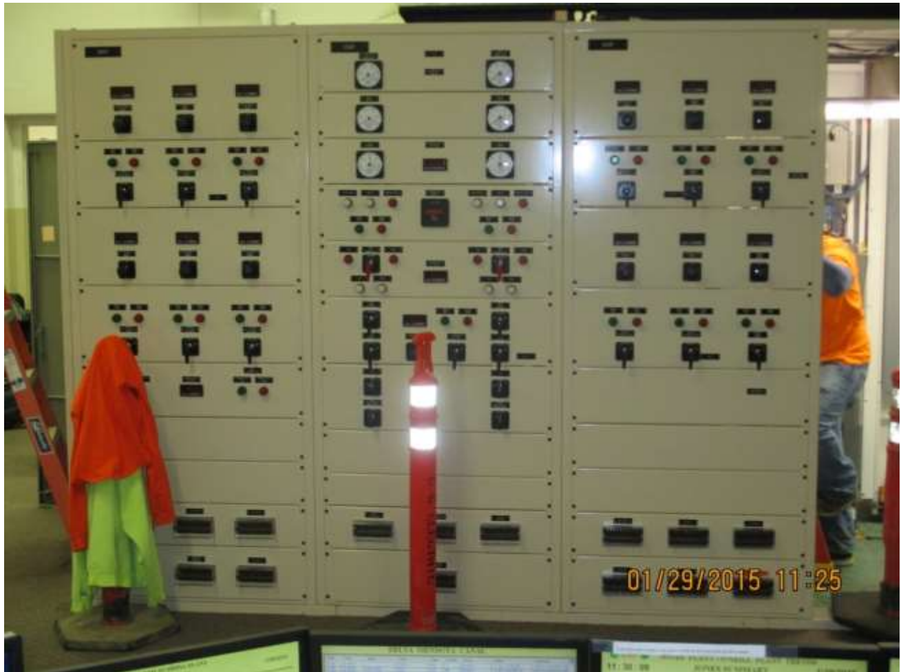
Tracy 13.8kV Switchgear/Breaker Replacement New panel skins CCA1F, CCA2F, and CCA3F, from left to right, installed
