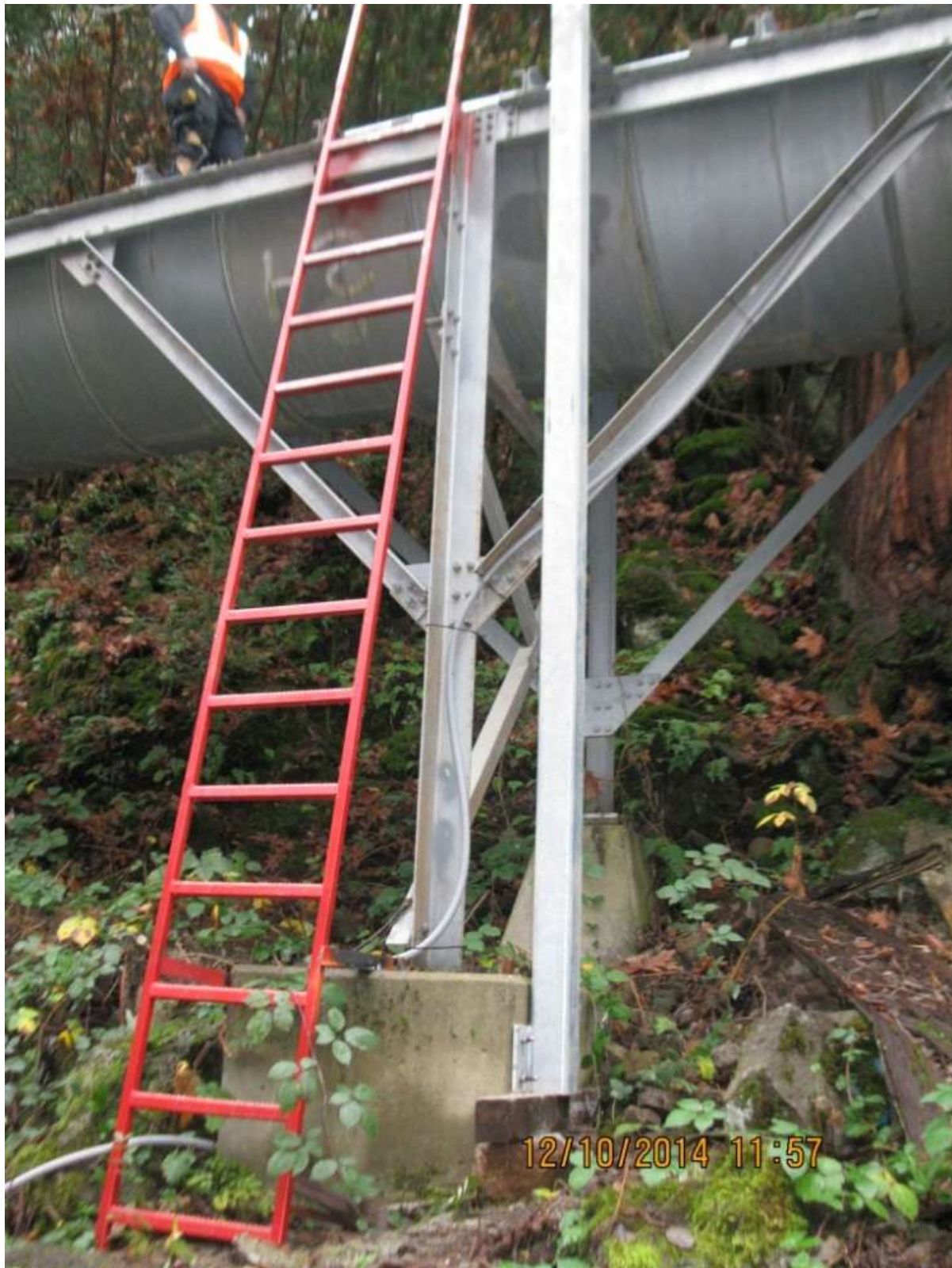
North Fork Screens and Ladders Gate Modulations Installation of steel support for the new flow sensor control panel.
