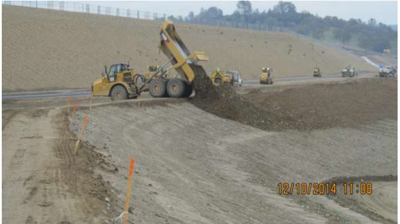
Mormon Dam Auxiliary Dam Overlay CAT 740B articulating end dump placing cobble slope protection material which was spread with the CAT D8T dozer between approximate stations 420+00 and 430+00.
