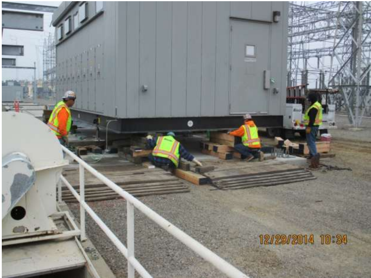
Tracy 13.8kV Switchgear/Breaker Replacement. Contractor lowering Building 11A onto the concrete slab using hydraulic jacks.
