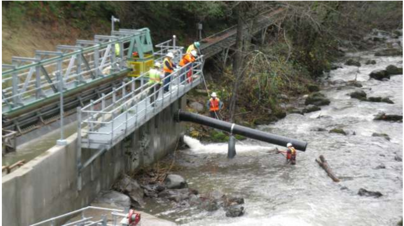
North Fork Screens and Ladders Gate Modulations Locating existing flow sensor and conduit for removal
