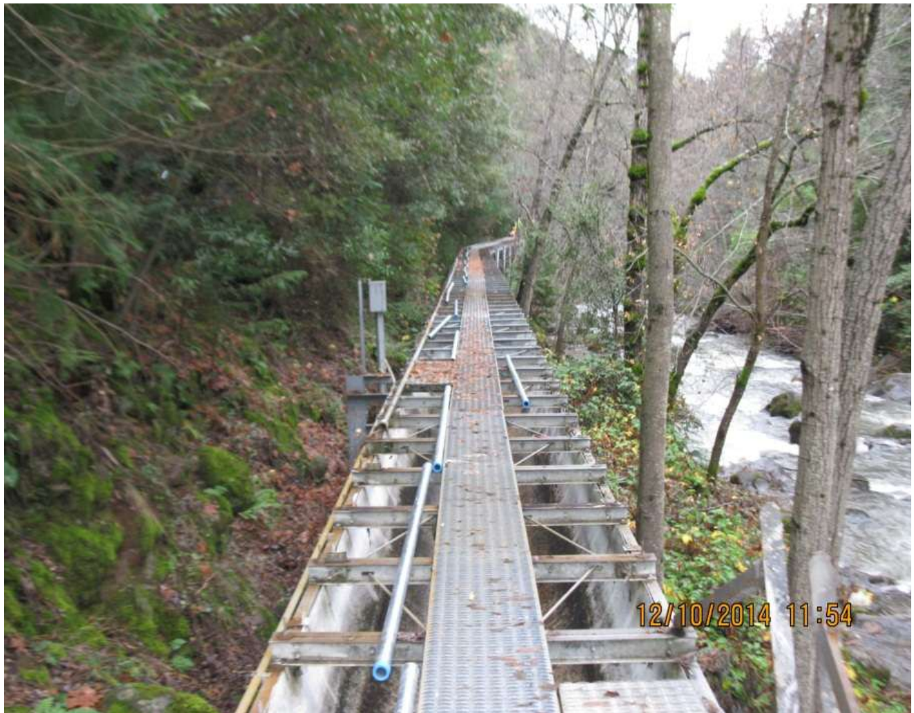
Battle Creek Salmon and Steelhead Restoration Project North Fork Screens and Ladders Gate Modulations Installation of new conduit to the new flow sensor control panel.
