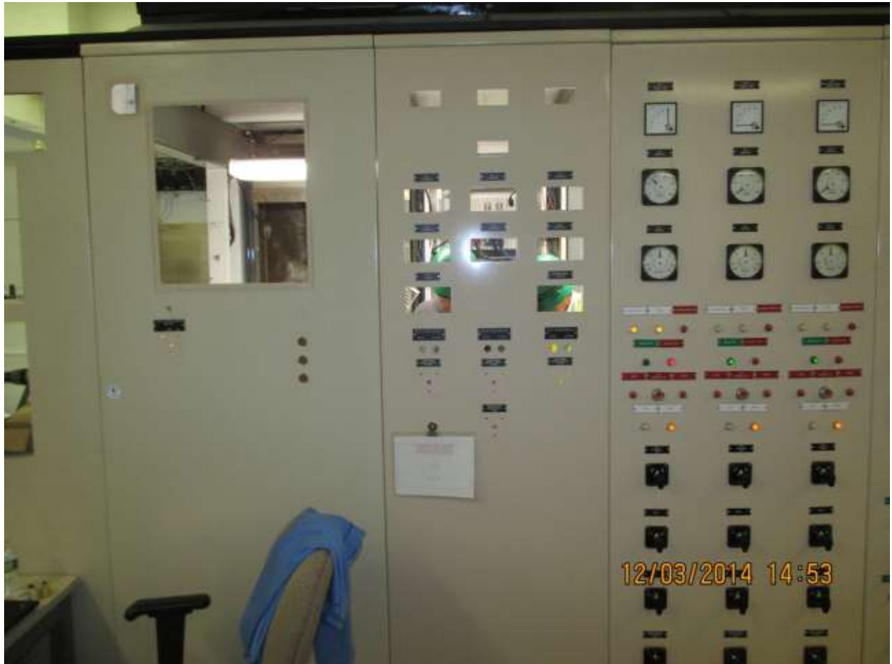
Tracy 13.8kV Switchgear/Breaker Replacement Contractors removing unused panel controls and wiring after installing proper labeling
