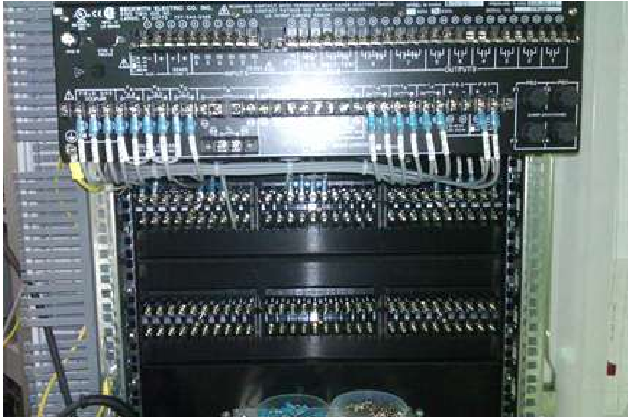
Folsom Power Plant Generators U1, U2, and U3 Rewind and Excitation System Replacement Depiction of wired connections between test switch X95 and the Beckwith relay
