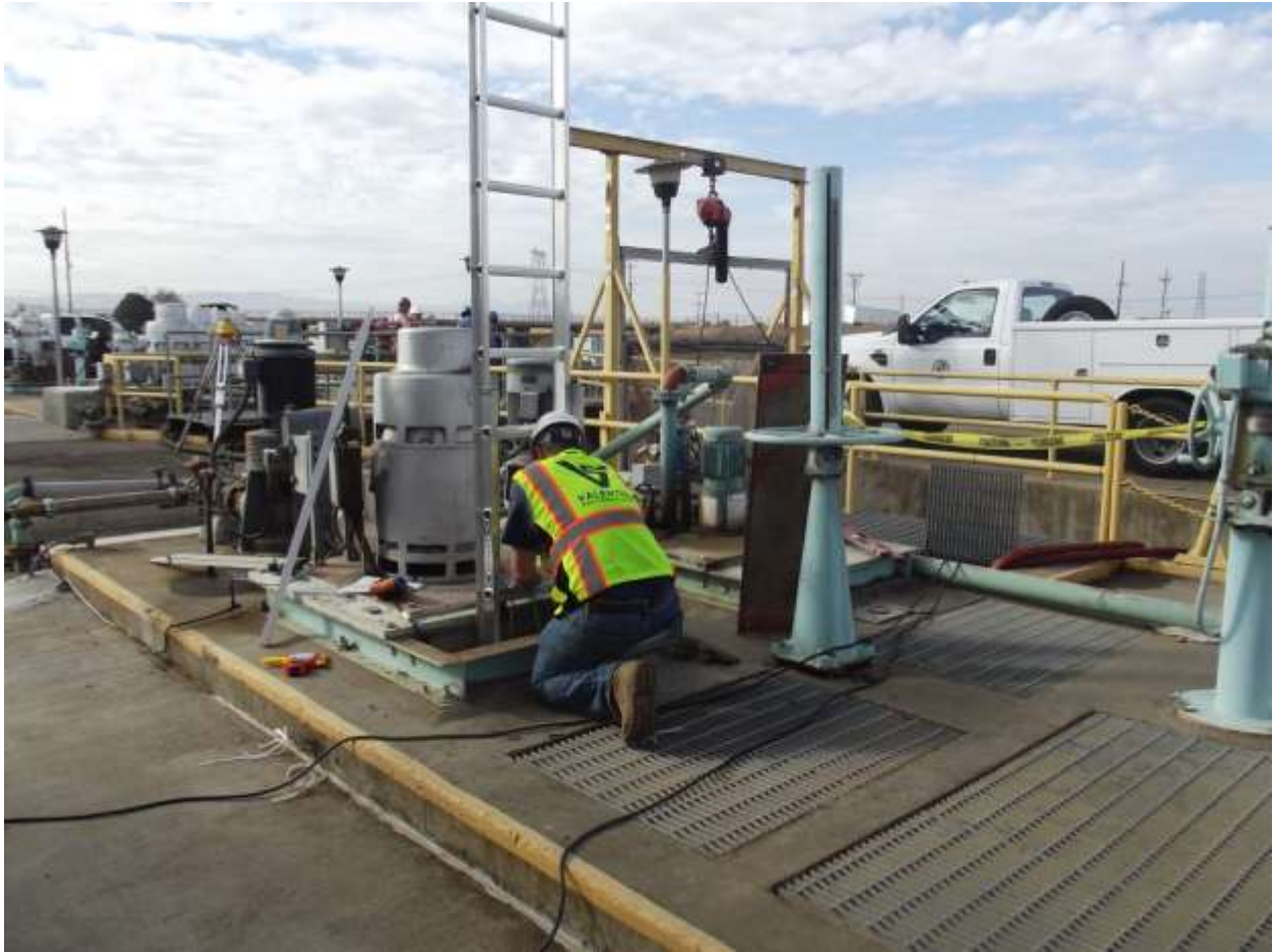
Tracy Fish Collecting Facilities, Secondary Louver Replacement The contractor's worker assisting the crew making measurements inside the pump pit to facilitate installation of the new pumps and fish screen
