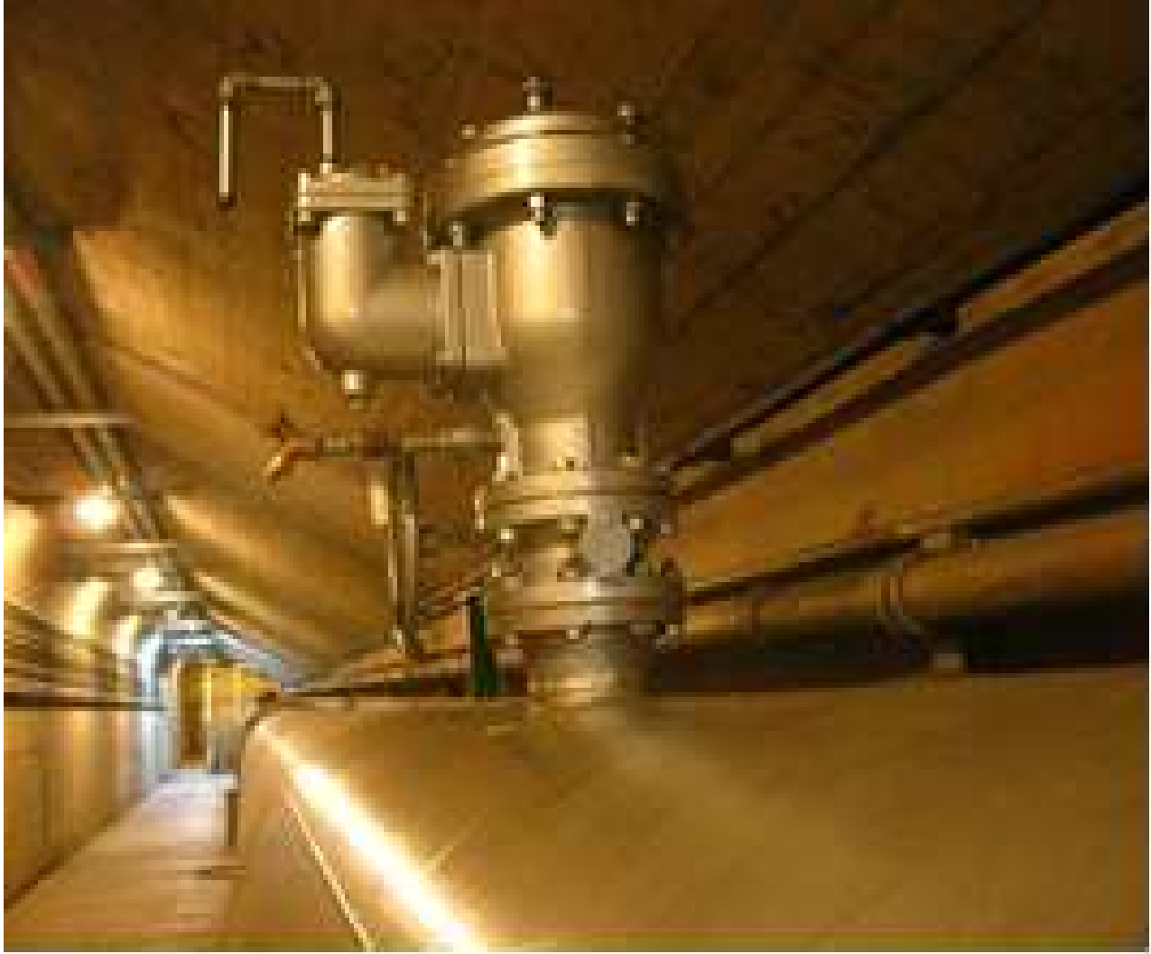
Northfork Pipeline Repair Folsom Pumping Plant New valve installed on pipeline (lighting causes golden appearance)
