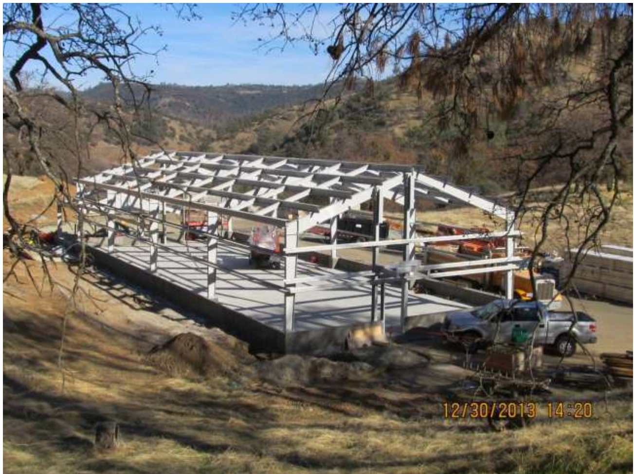
New Melones Artifact Storage Building Major steel components of the building
