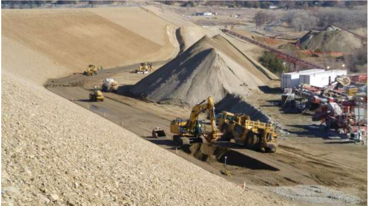
Mormon Dam Auxiliary Dam Overlay Caterpillar 336E Excavator excavating the coarse filter zone
