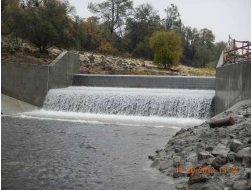
Baldwin Creek Fish Barrier Completed fish barrier structure
