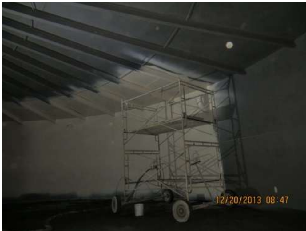
San Louis Demonstration Treatment Plant Coating of interior of sump water storage tank
