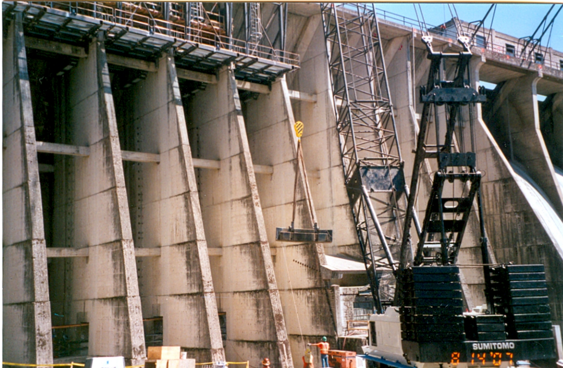
CN22-200-0743 Stony Gorge Dam Modification. Orland Project, CA. Shimmick Construction Company Inc. Spec/Contract No. CO642/06CC202026. BOR. Contractor is performing a load test on the 165-ton Sumitomo crane using the 60,000lb counter weight from the 165-ton American crane. Photo by D. Milani. 8-14-07.
