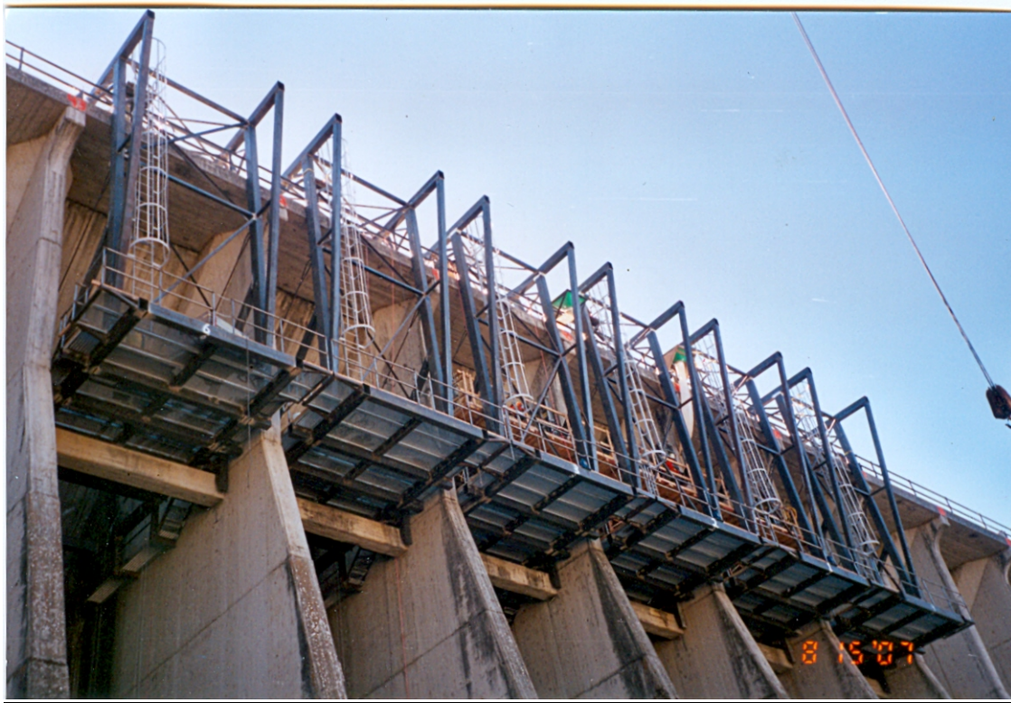
CN22-200-0745 – Stony Gorge Dam Modification, Orland Project, CA. Shimmick Construction Company Inc. Spec/Contract No. CO642/06CC202026. BOR. Six of seven C-hangers installed between bays 37-43. Contractor did rebar scan survey, Core drilled end threaded anchor bar, set capital/strut forms and placed concrete from C-hangers. Photo by D. Milani. 8-15-07
