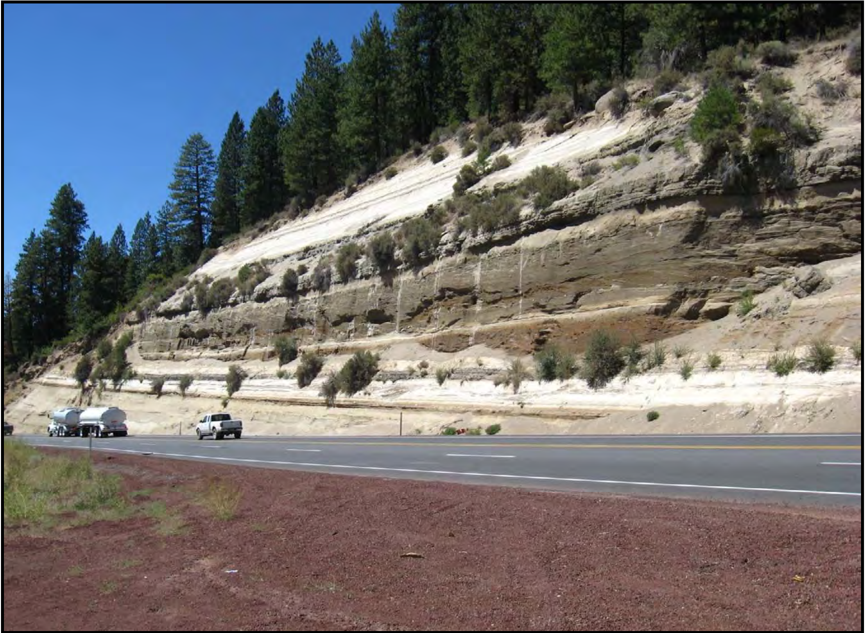
Photo 16. View of cutslope along Hwy 97 about 6 miles north of Chiloquin, Oregon. Exposed are deposits of airfall tuff and alluvial volcaniclastic tuffaceous sediment that form an escarpment about 400 feet above the Williamson River flood-plain. The current mapping did not determine if deposits such as shown here can be traced into the project area. Photo by M. McCulla, 8/22/07.
