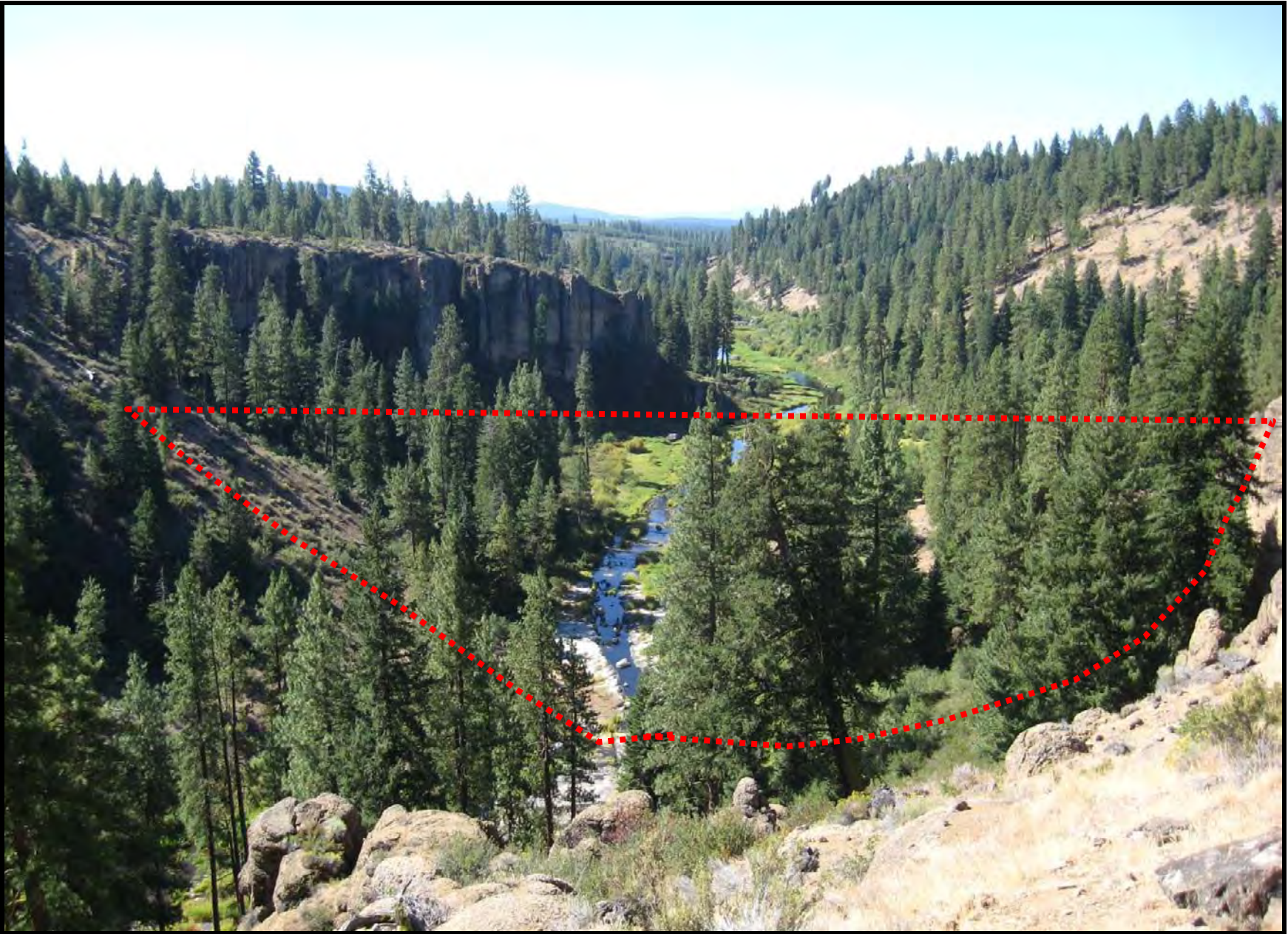
Photo 9. Downstream view of the Williamson River Canyon. The dotted line represents the proposed location of an embankment (approximately 150 feet high) for a water storage project in the SE \frac{1}{4} , NW \frac{1}{4} , Sec 25, T33S, R7E. Both abutments of the site are composed of moderately to well indurated tuff breccia (Qtb) and other volcanoclastic rock. Photo by M. McCulla, 8/22/07.
