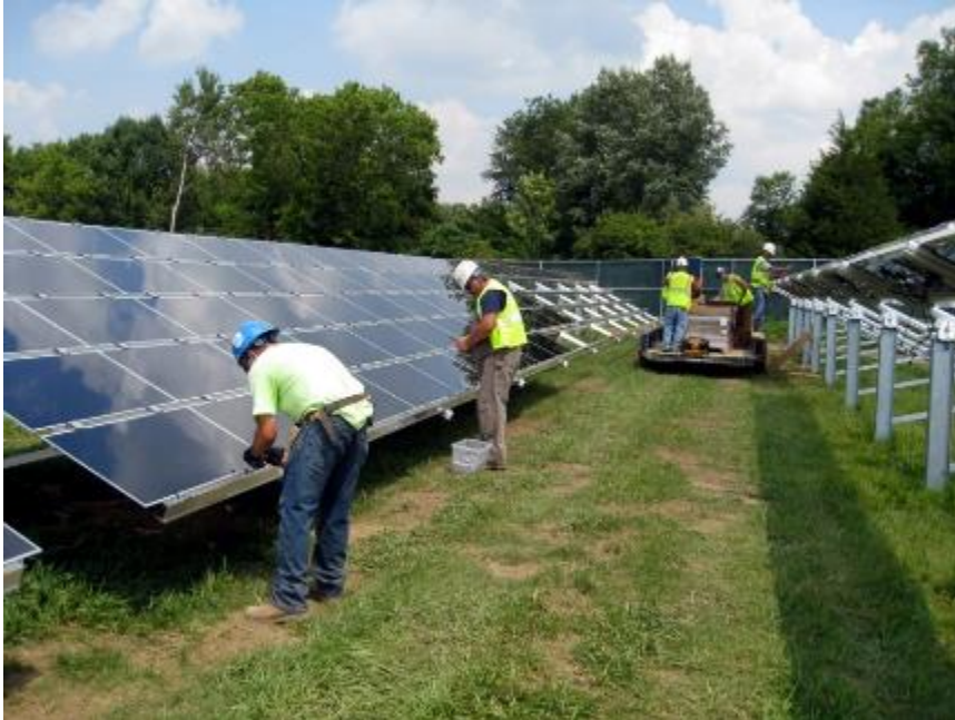
Figure 6-11. Installation of Utility-Scale Solar Arrays at Shared Solar Facility
