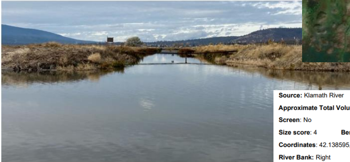
Figure 32. Diversion at KENO-18. October 2021.
