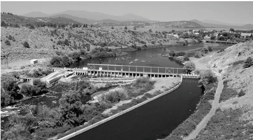
FIGURE 2-2d The Link River Dam, shown in this 2006 view from the same location as the views in Figures 2-2 a, b, and c, now includes a fish ladder, recently installed near the right abutment (left side of the dam in this image).
