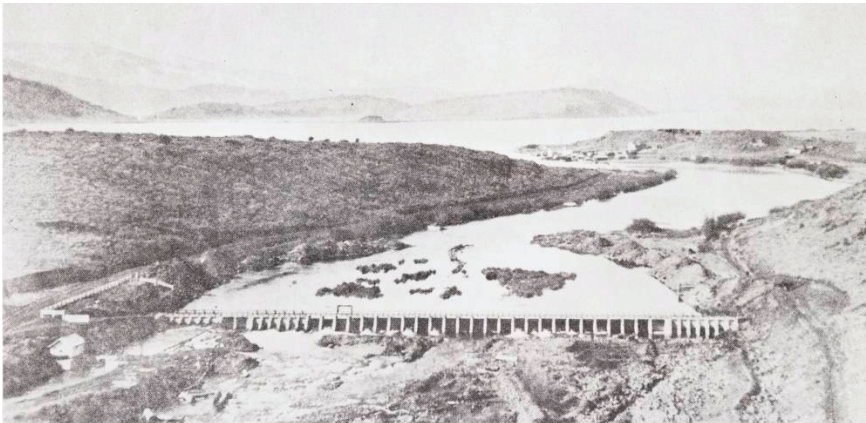
FIGURE 2-2b The newly completed Link River Dam spans the channel and diverts much of the river's discharge into the Keno Canal on the right bank in this 1922 image made from the same location as in Figure 2-2a. SOURCE: Boyle 1976. Reprinted with permission; copyright 1976, Klamath County Museum.
