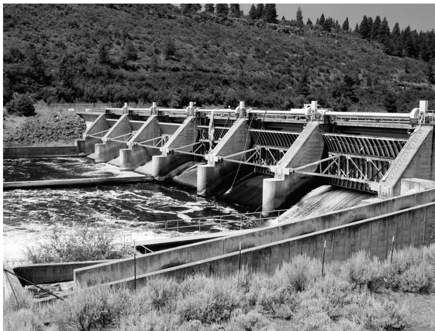
FIGURE 4-1 Keno Dam rests atop a bedrock sill across the Klamath River near Keno, Oregon. The fish ladder for the dam is on the left abutment of the dam in the foreground of this view.
