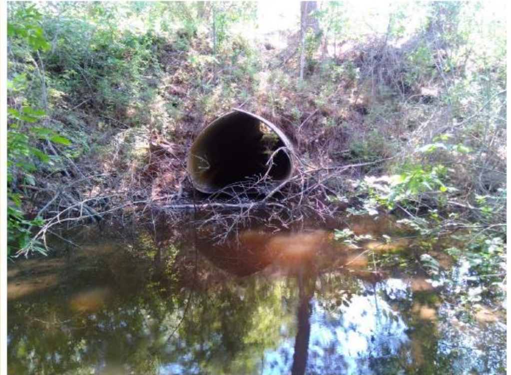
Figure 48. Looking upstream from the stream channel at the Ager Beswick culvert on Deer Creek on 06/25/2021.
