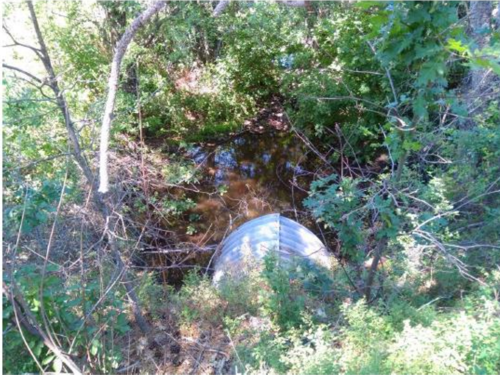
Figure 47. Looking downstream from the road at the Ager Beswick culvert on Deer Creek on 06/25/2021.
