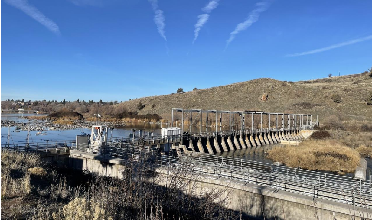
Link River Dam December 2021
