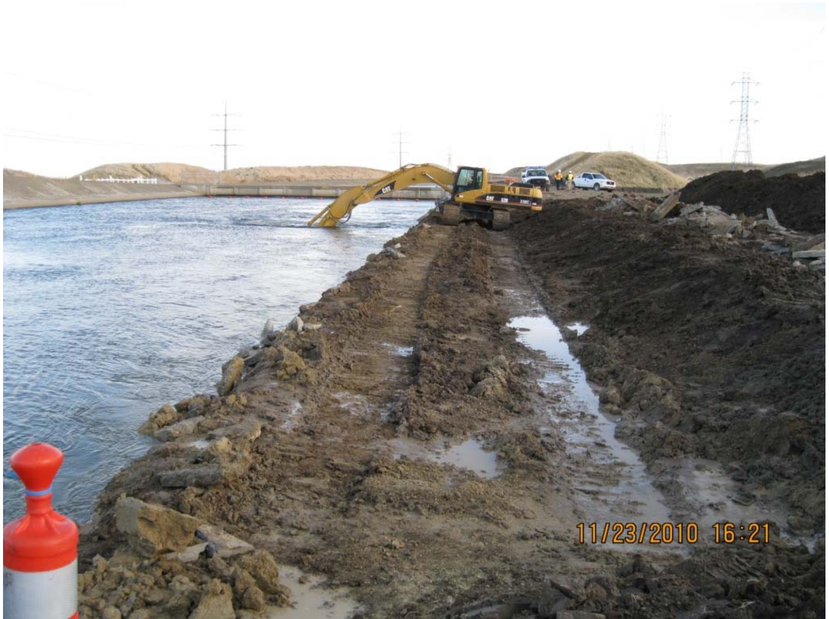
Removal of canal's concrete liner using excavator
