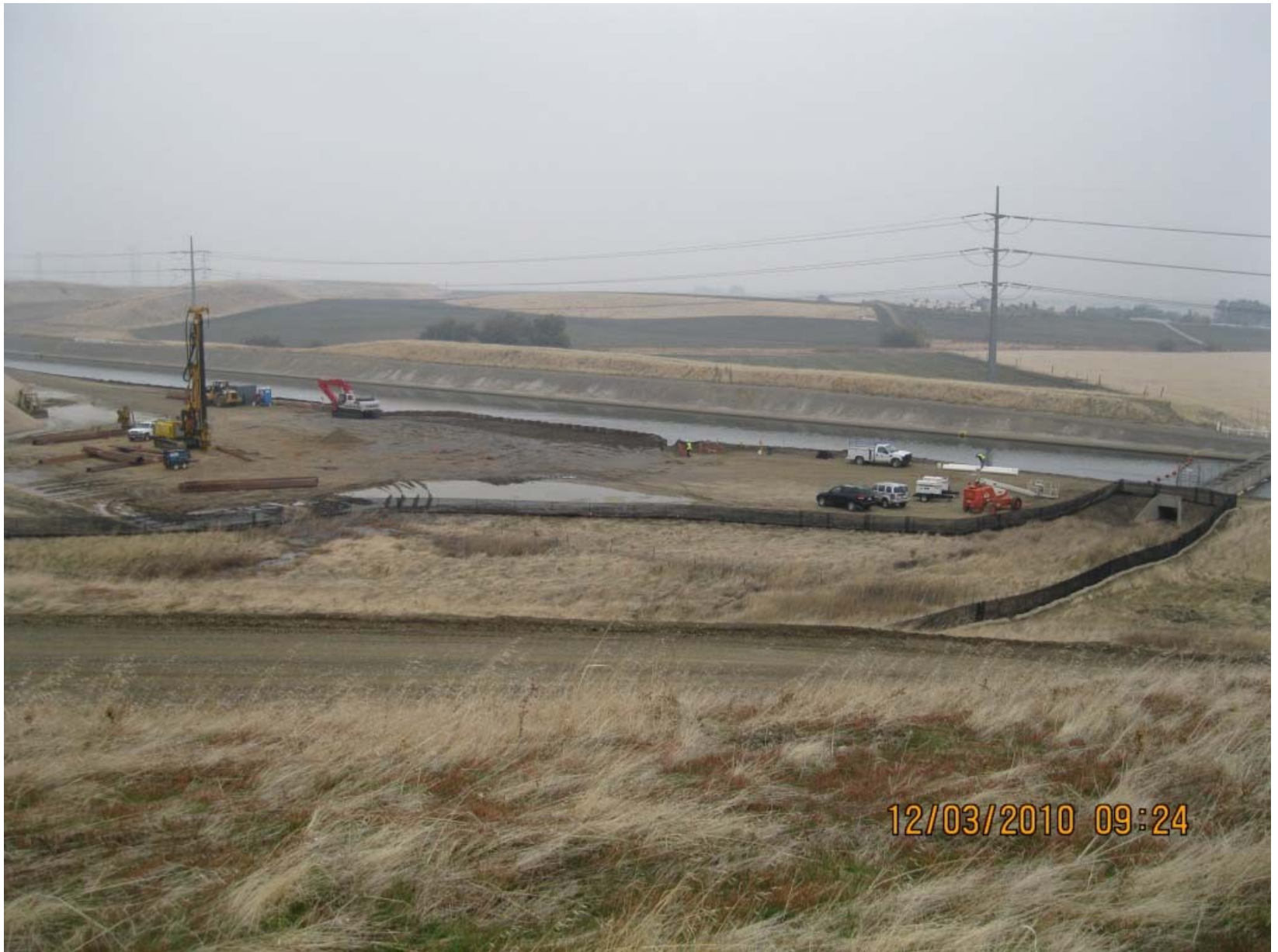
Work area exclusion fence
