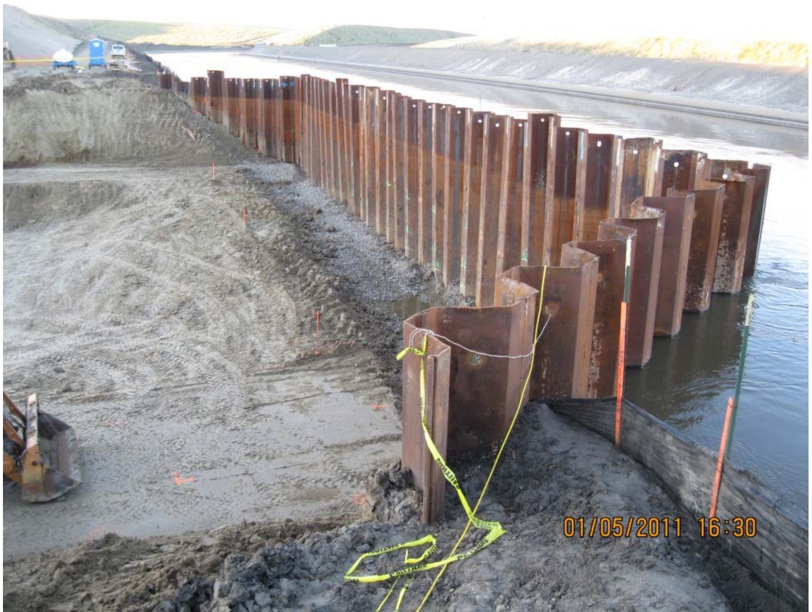
Excavation at intake to Pump Plant on Delta-Mendota Canal
