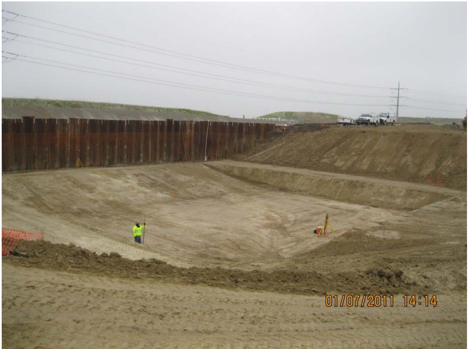
Excavation to finish grade
