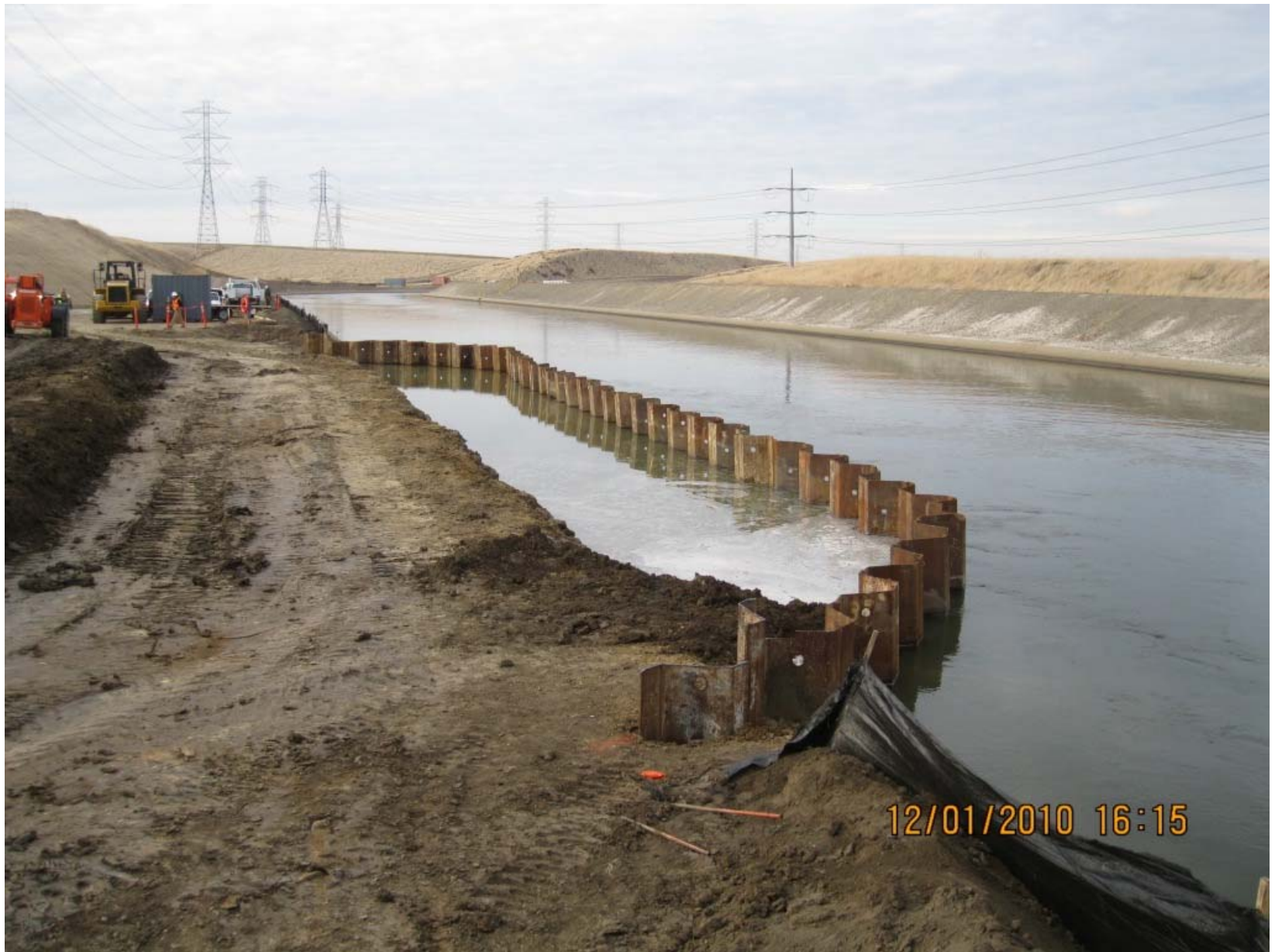
Intermediate sheet piles set into DMC
