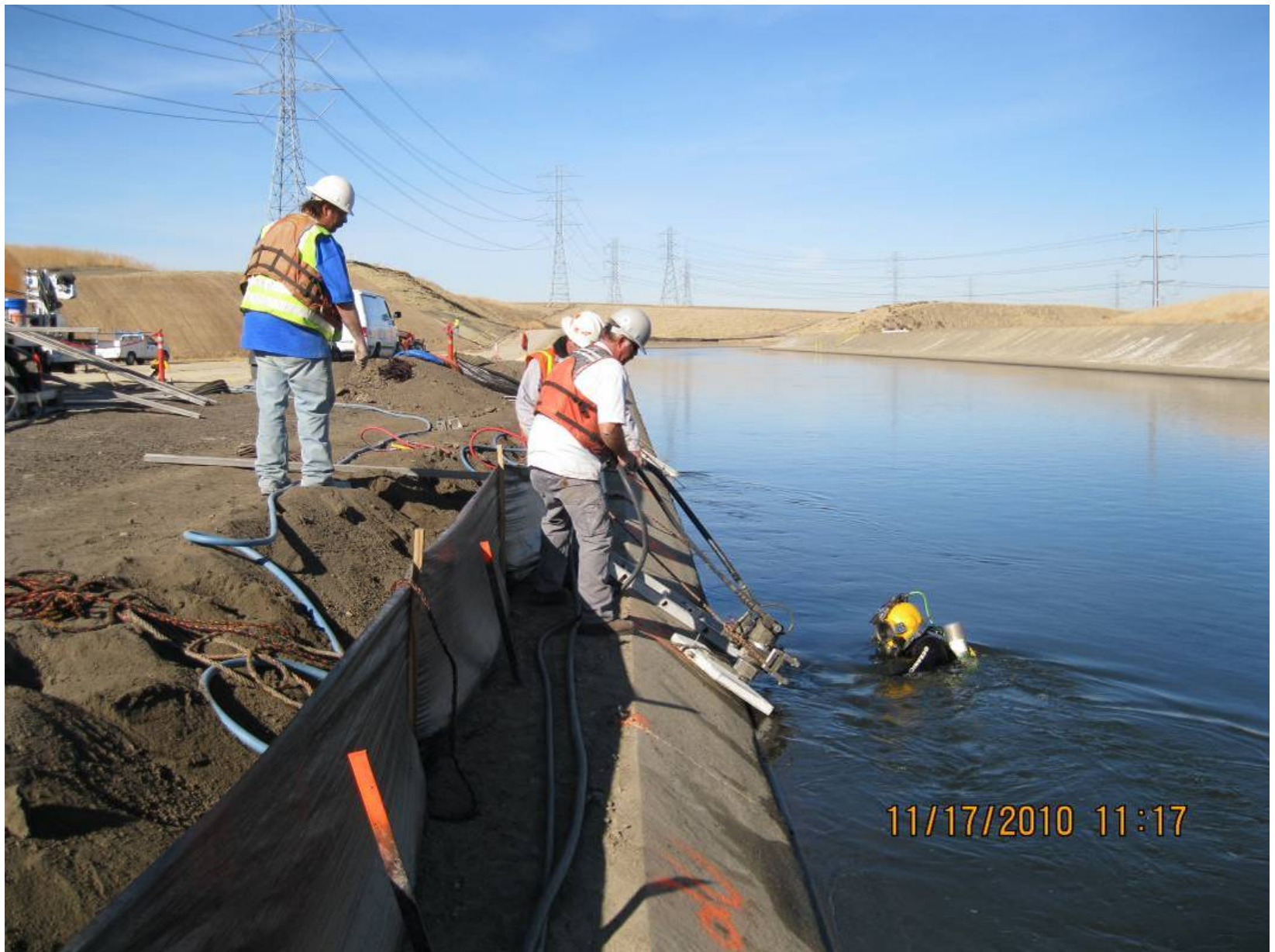
Diver beginning canal liner concrete cutting using 12" radius saw.
