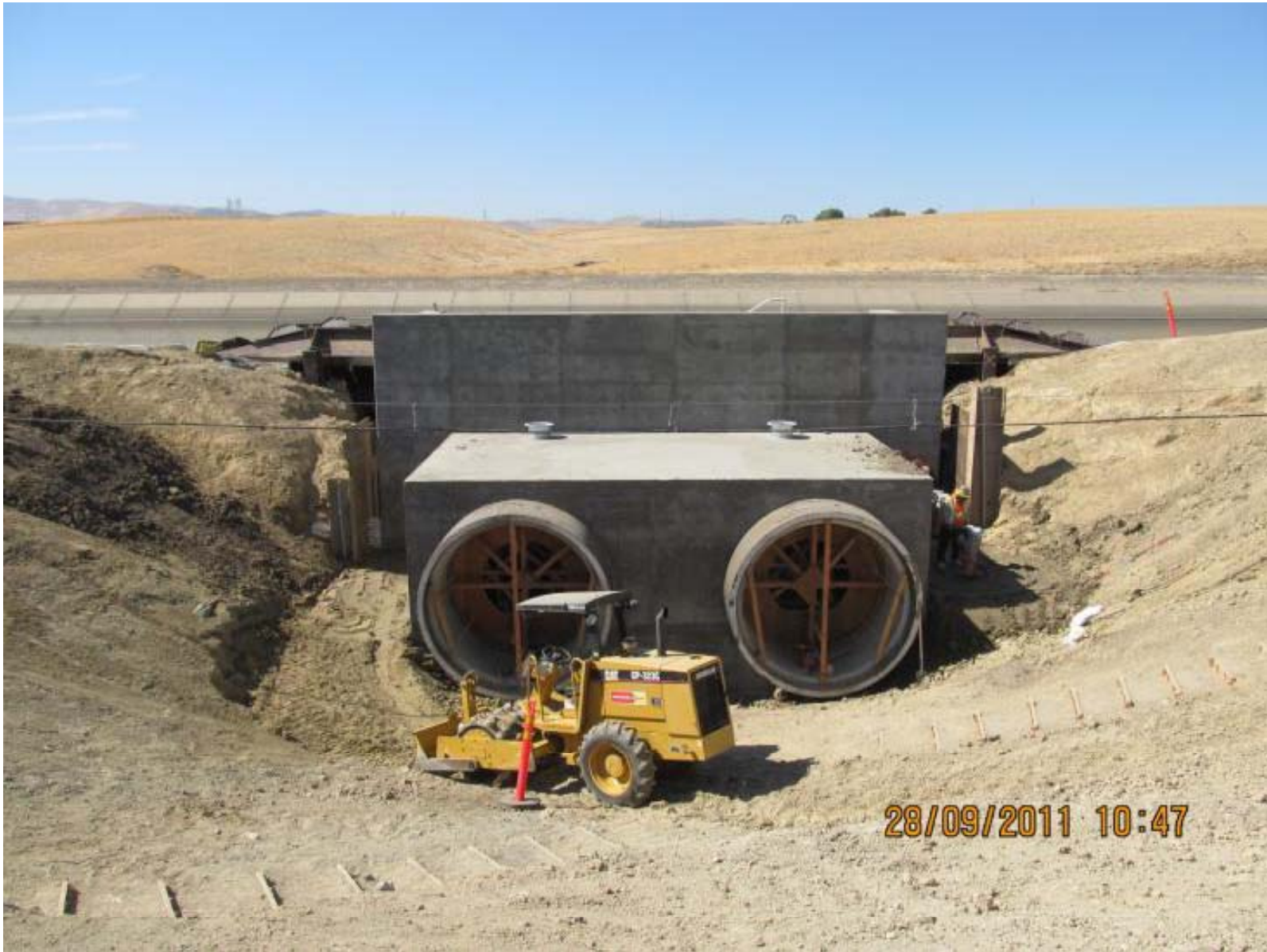
California Aqueduct Turnout concrete complete
