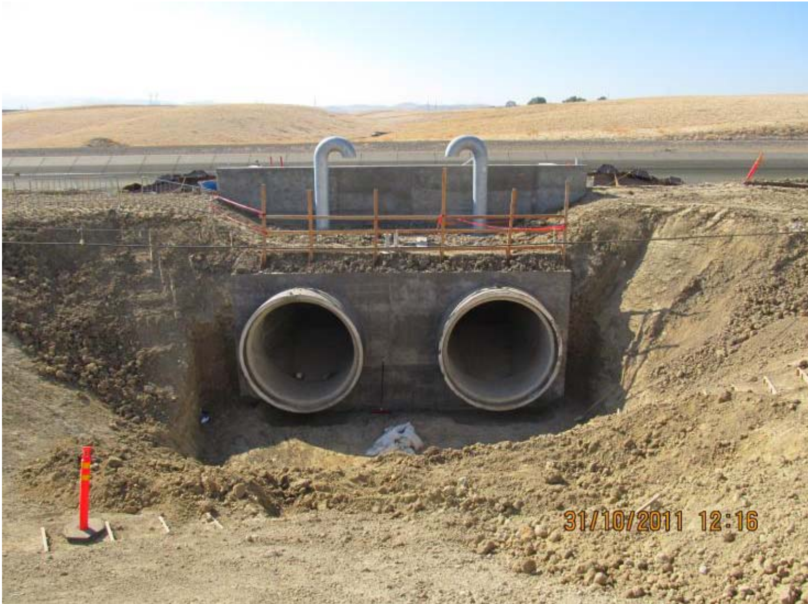
California Aqueduct backfilled and gooseneck vents installed
