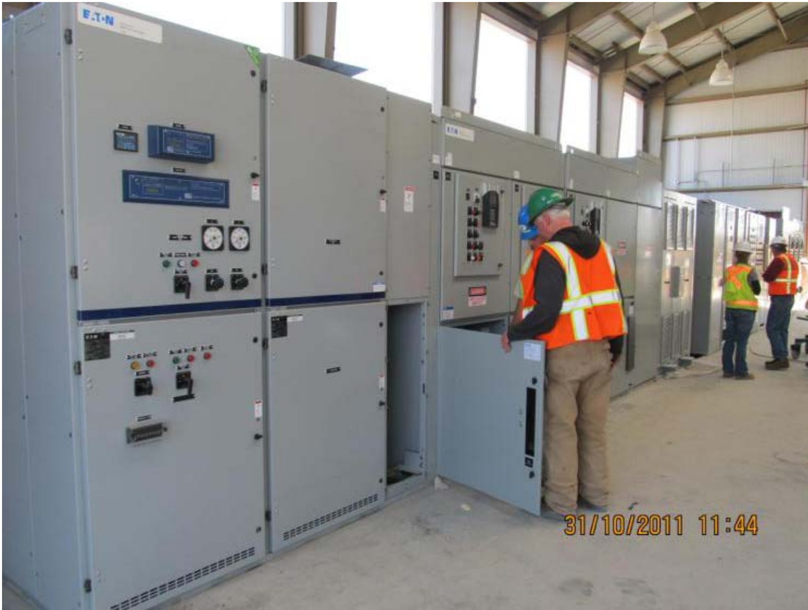
Installing Pumping Plant Motor Control Center
