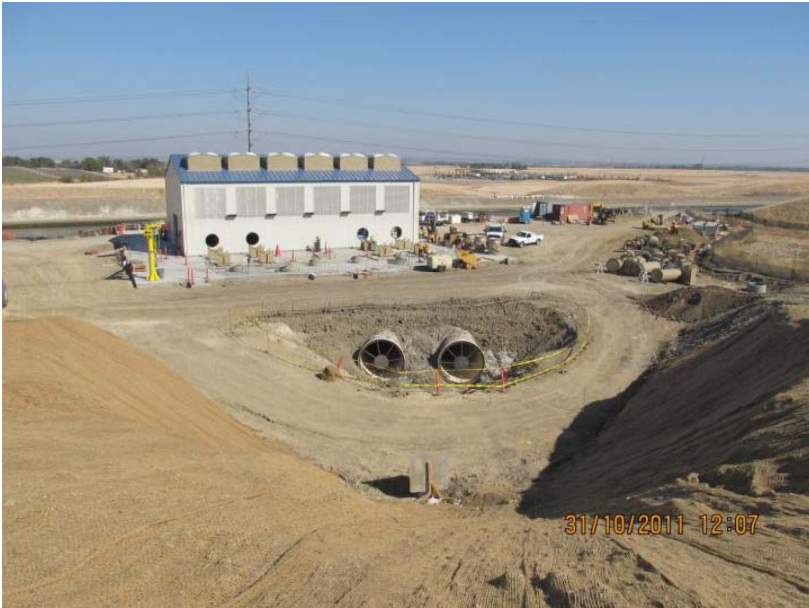
108-inch steel pipe backfilled; concrete deck complete
