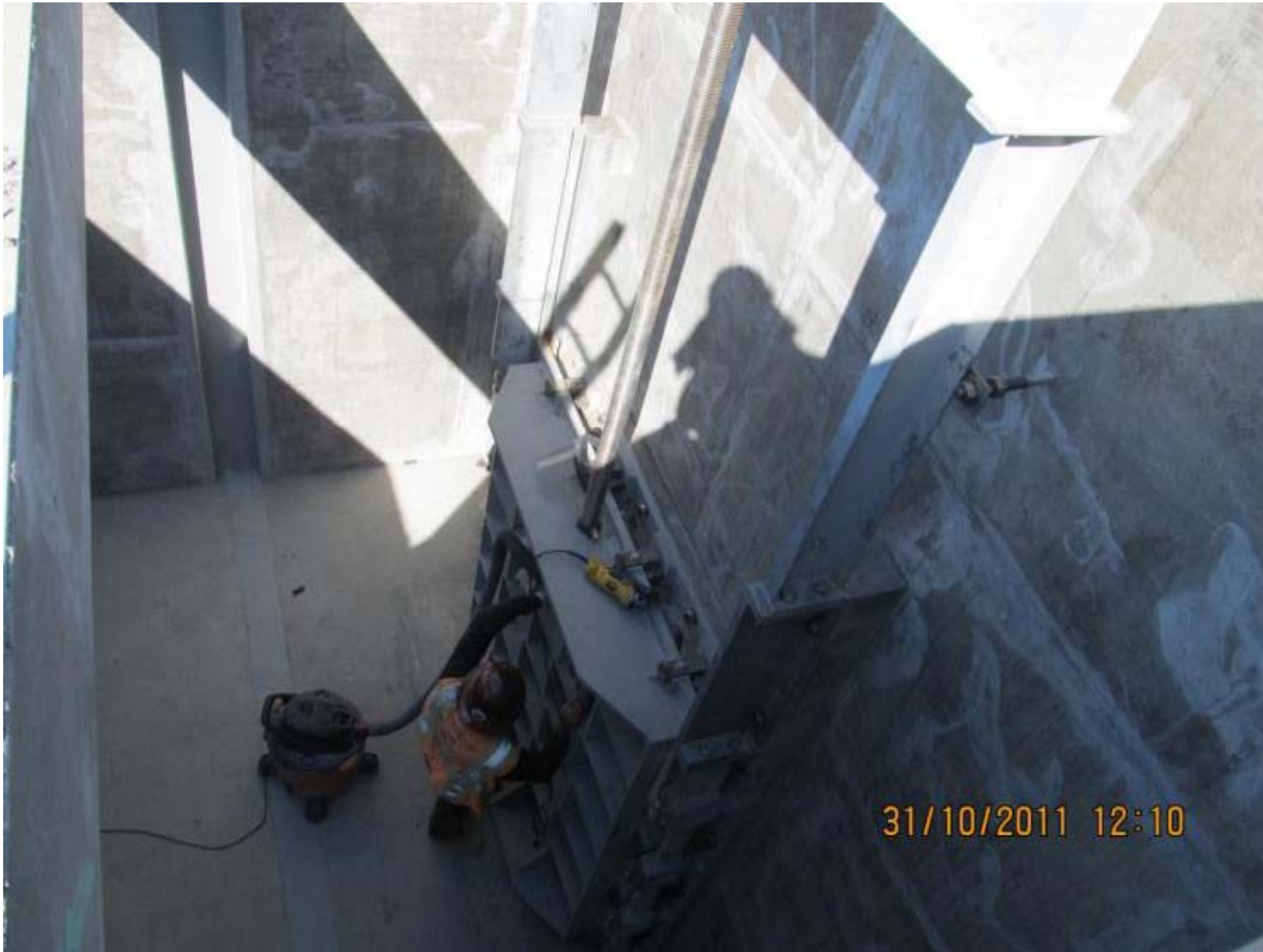
California Aqueduct turnout slide gate
