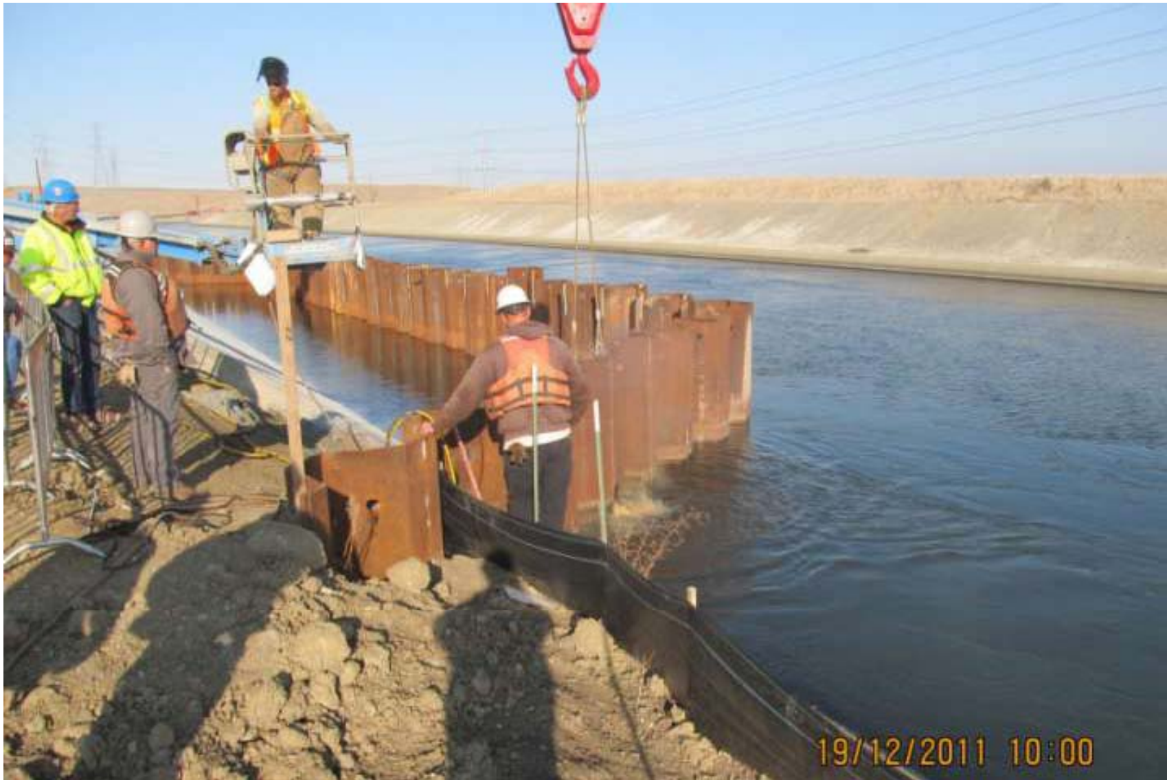
Divers use an air-arc to cut DMC coffer dam sheet piles
