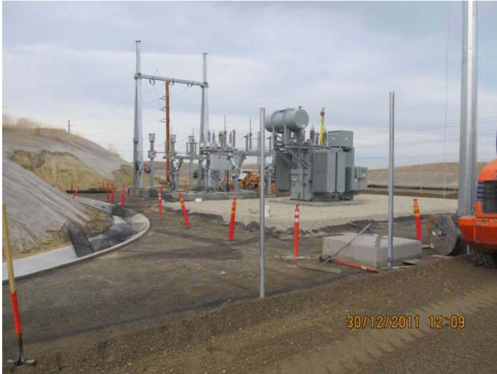
Geogrid laid at the switchyard awaits compacted gravel on December 30th
