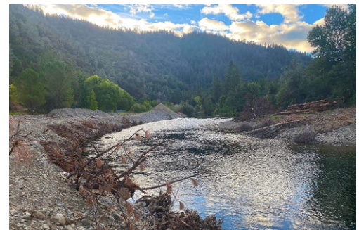
Looking upstream in a new meander constructed on the mainstem Trinity River at the Chapman Ranch Phase B Channel Rehabilitation Project restoration site. Trees with rootwads are buried in the bank to provide stability while riparian vegetation grows in.
