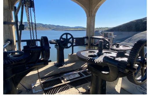
Orland Unit Water Users Association completed the dam's replacement regulating gate installation and the lower and mid-level gates' rehabilitation last fall (its machinery is shown in this photo).
