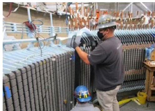
Contractor employee installing one of the 228 new multi-turn coils into the slots in the new stator as part of the Jones Pumping Plant Unit Rewind Project. The C.W. “Bill” Jones Pumping Plant operates in conjunction with the nearby Tracy Fish Collection Facility to protect and salvage fish from pump operations.
