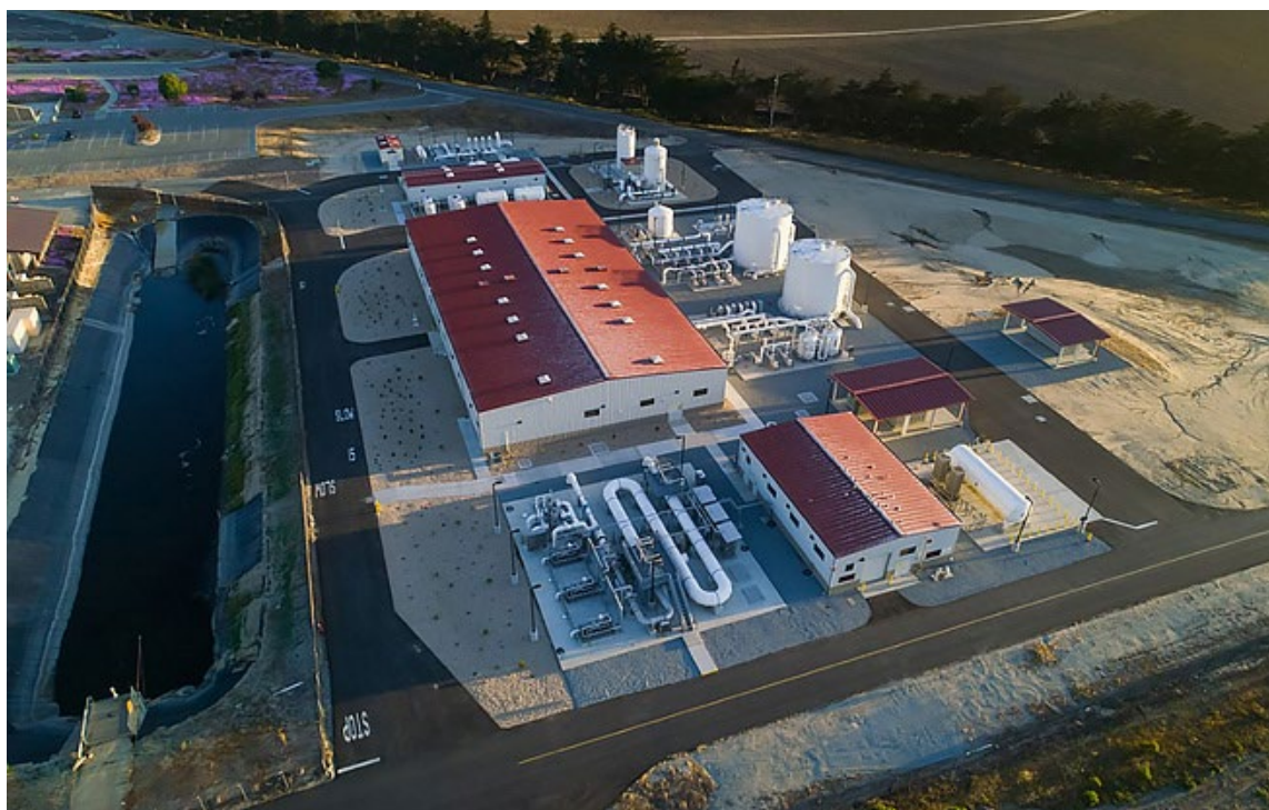
This advanced water purification facility serves 12 Monterey County communities, providing wastewater treatment services and recycling 4 billion gallons of crop water.
