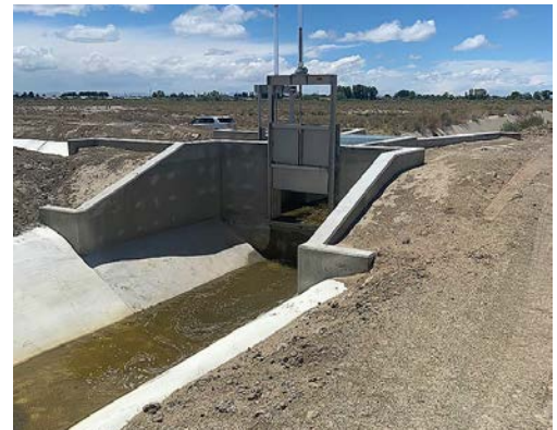
A Fallon Paiute-Shoshone Tribal grant in west-Central Nevada improved and expanded a Reclamation canal within the Reservation. Photo shows a 4-foot stainless steel slide gate at Segment 1 in May 2021.
