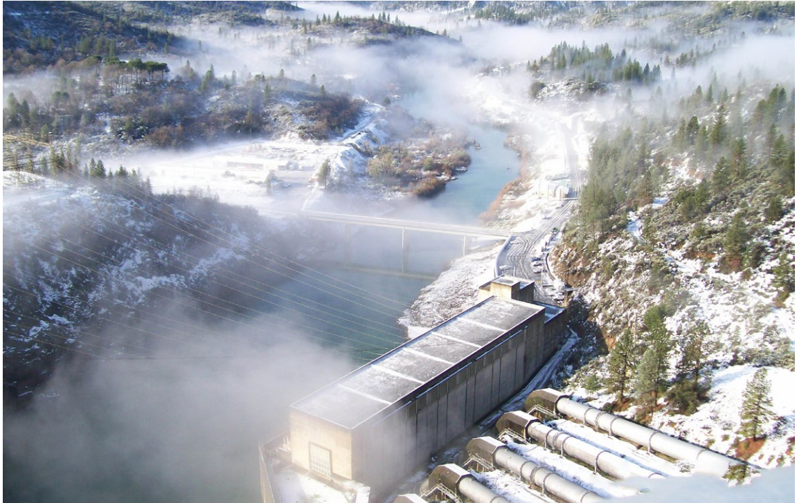
Shasta Powerplant is located just below Shasta Dam and includes five main generating units which have a capacity of approximately 710 megawatts.
