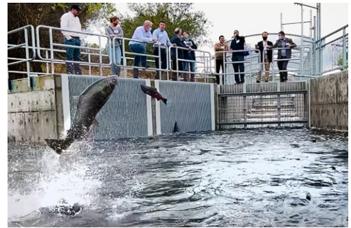
Visitors view returning fish at the entrance of the new Nimbus Fish Hatchery ladder — a more reliable, safer system for collecting adult fall-run Chinook salmon and Central Valley steelhead trout.
