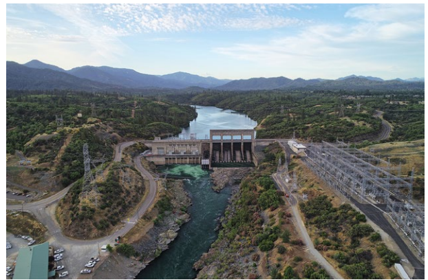
Aerial view of Keswick Dam and Powerplant. CVP power generation is 'shaped' so that maximum production is predominantly available during peak demand hours from afternoon through early evening.
