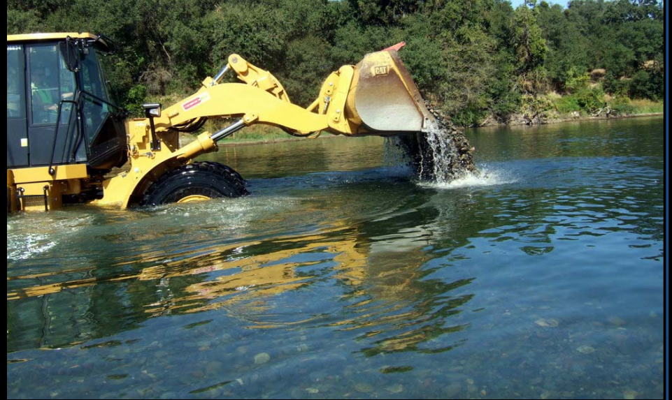
Gravel Placement at Upper Sunrise
