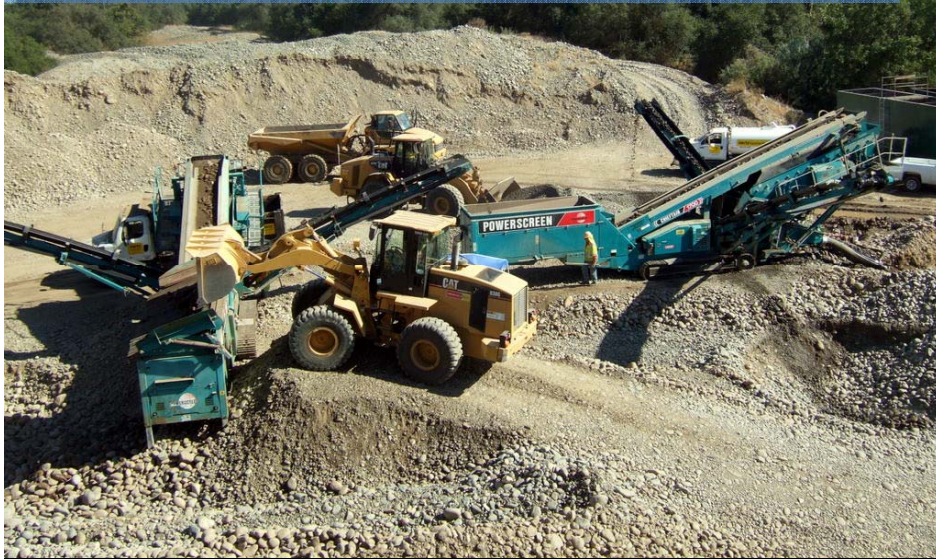
Sorting Dredger Tailings for Placement into American River
