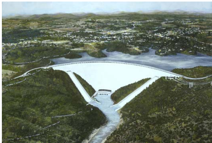
Figure II-1. Artist Rendition of Double Curvature Concrete Arch Auburn Dam and Powerplant at River Mile 20.1 on North Fork American River
