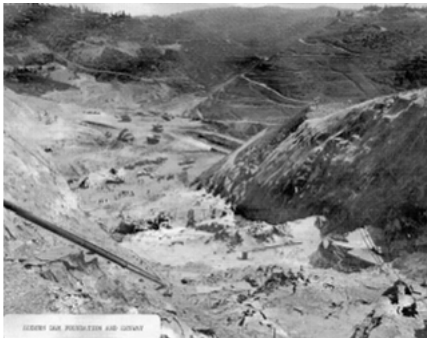
FIGURE II-3. WORK AT AUBURN DAM SITE
