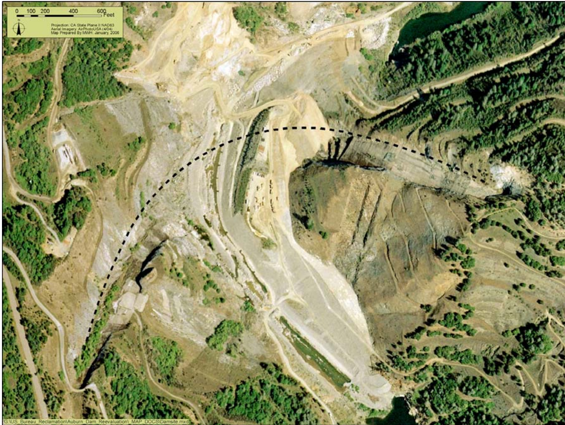
FIGURE II-4. AERIAL VIEW OF AUBURN DAM SITE AND FOUNDATION
