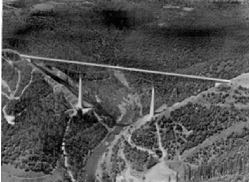
FIGURE II-2. AUBURN-FORESTHILL BRIDGE LOOKING NORTH
