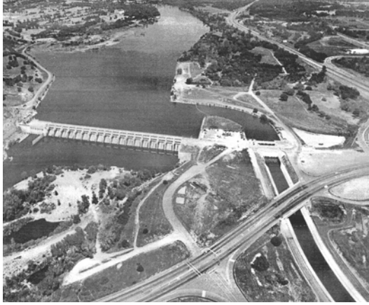
FIGURE II-8. UPSTREAM DIVERSION OF THE FOLSOM SOUTH CANAL FROM LAKE NATOMA LOOKING EAST
