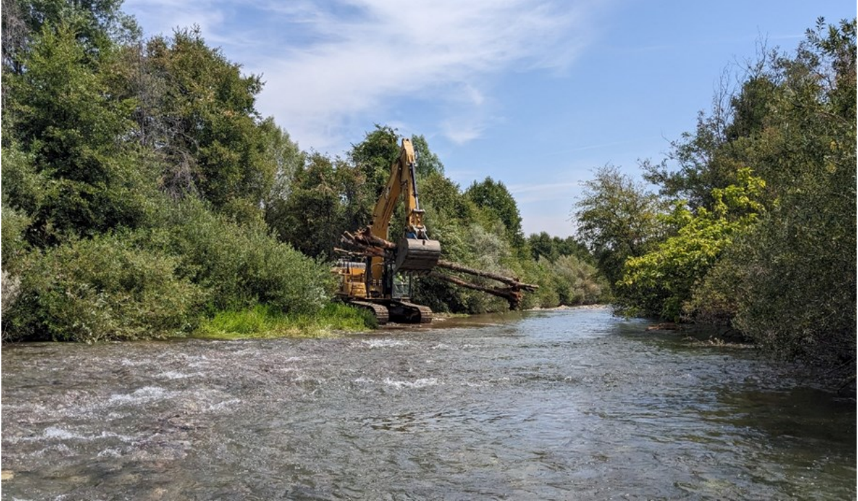
Figure 12. Large wood placements at the Gold Dredge augmentation site in 2024.
