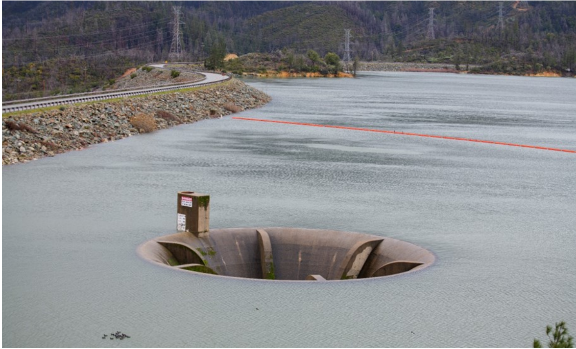
Figure 4. Water cresting the Whiskeytown Dam spillway during the WY 2024 gloryhole spill event. (Reclamation/M. Burke)
