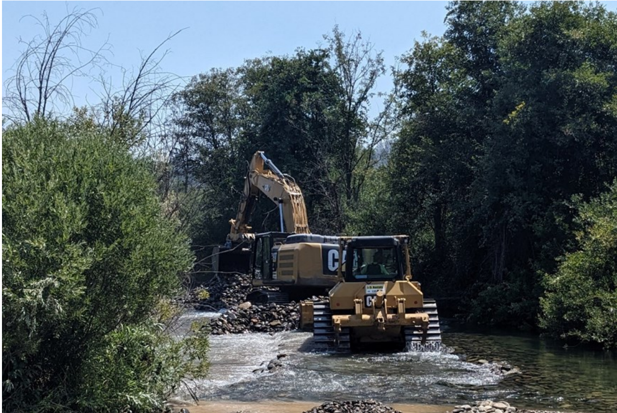
Figure 10. Riffle supplementation implementation at the Phase 2A/Gold Dredge gravel augmentation site in WY 2024.
