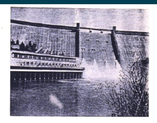
Shasta Dam bypass through low level outlet valves to meet temperature objectives.
