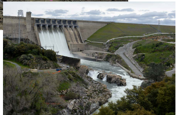
Folsom Lake storage was at an extremely low stage after three years of drought with the temperature control shutter system exposed (above; taken on November 14, 2015). Four months later, Folsom Lake storage recovered and flood control spills occurred after several intensive winter storms (right; taken on March 8, 2016). Photo credit: Yung-Hsin Sun; used with permission.
