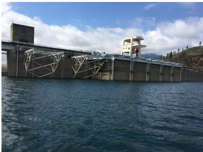
Upstream face of Shasta Dam in 2017, showing the top of the TCD. Photo credit: Watercourse Engineering, Inc; used with permission.
