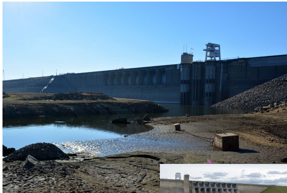
Folsom Lake storage was at an extremely low stage after three years of drought with the temperature control shutter system exposed (above; taken on November 14, 2015). Four months later, Folsom Lake storage recovered and flood control spills occurred after several intensive winter storms (right; taken on March 8, 2016). Photo credit: Yung-Hsin Sun; used with permission.
