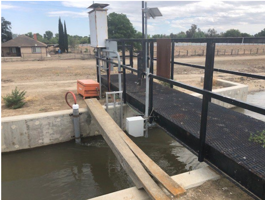
Real-time diversion monitoring of flow and salinity at the Patterson Irrigation District inlet
