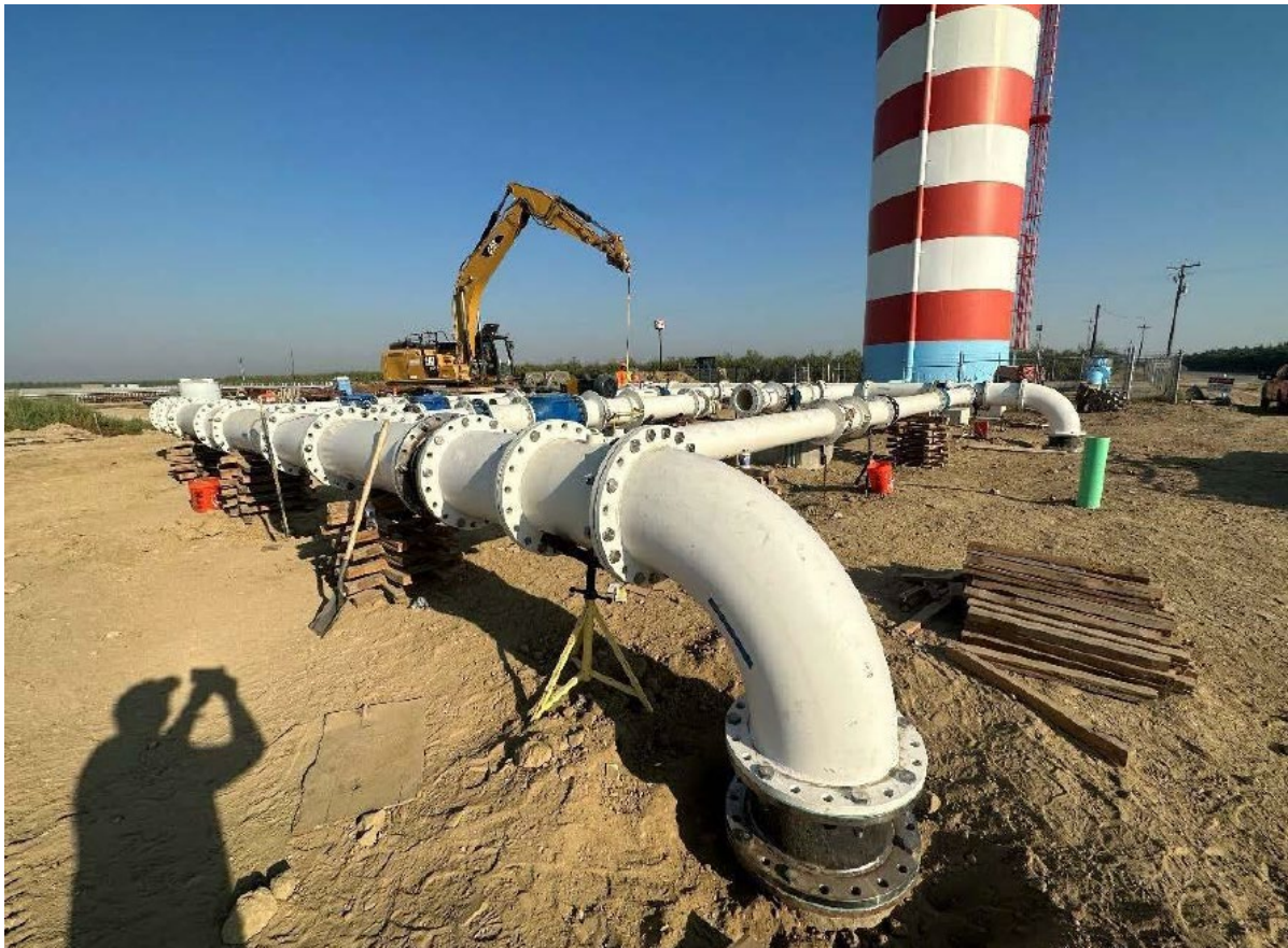
Semitropic Water Storage District's Cal Fed B230 System Extension Project showing the installation of the Pumping Station. (Reclamation photo)
