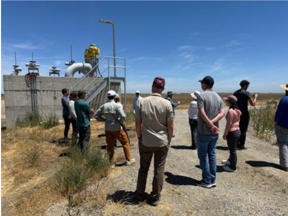
Field trip hosted by SJVDA and Reclamation to the SJRIP facility, showcasing the control center and pump station for the new temporary subsurface drainage storage system (Reclamation photo)
