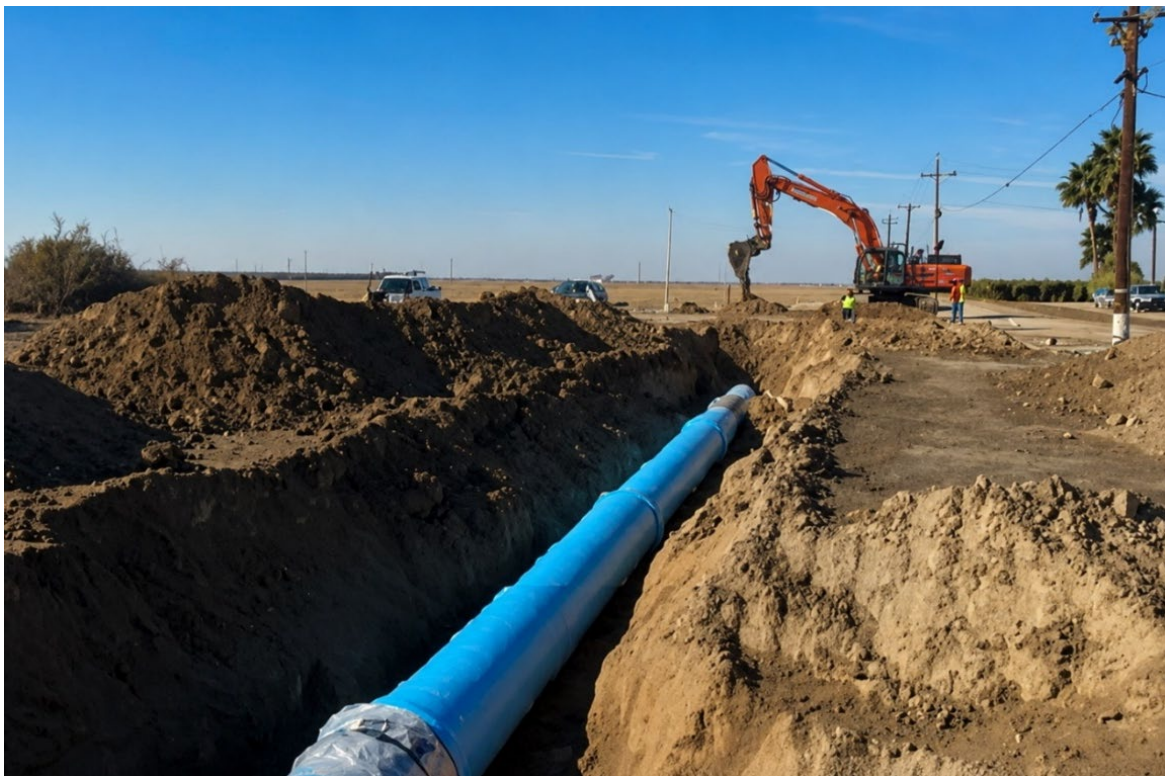
Semitropic Water Storage District installs pipeline at Lateral DE-1-A to improve water conveyance efficiency and support Bay-Delta water conservation efforts. (Reclamation courtesy photo)
