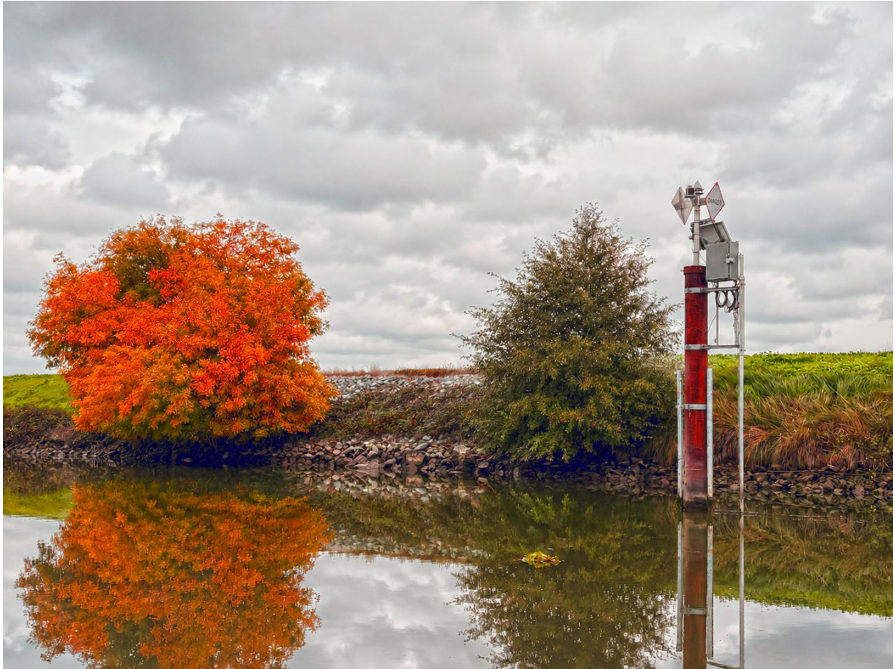
Late-fall view of the South Mokelumne River monitoring station. (Lillian McCormick, Reclamation)
