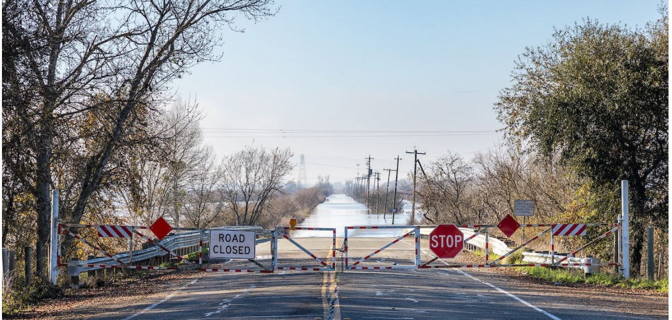
Closed county road in Yolo County due to high water and flood overtopping from Fremont Weir near the Big Notch. (DWR photo)
