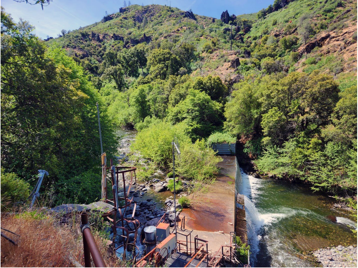
South Diversion Dam to be removed (Reclamation photo)
