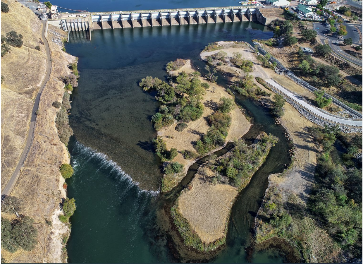
Figure 5. Completed project at Nimbus Basin, October 22, 2022. Salmon can be seen holding along the upstream part of the riffle (small black areas).
