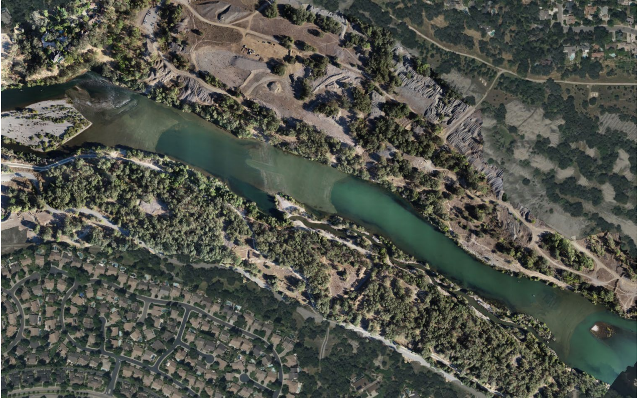
Figure 4. Aerial view of completed project at Lower Sailor Bar, September 30, 2022. The two side channels can be seen on the south side of the river and the three lighter colored areas are the gravel placements.
