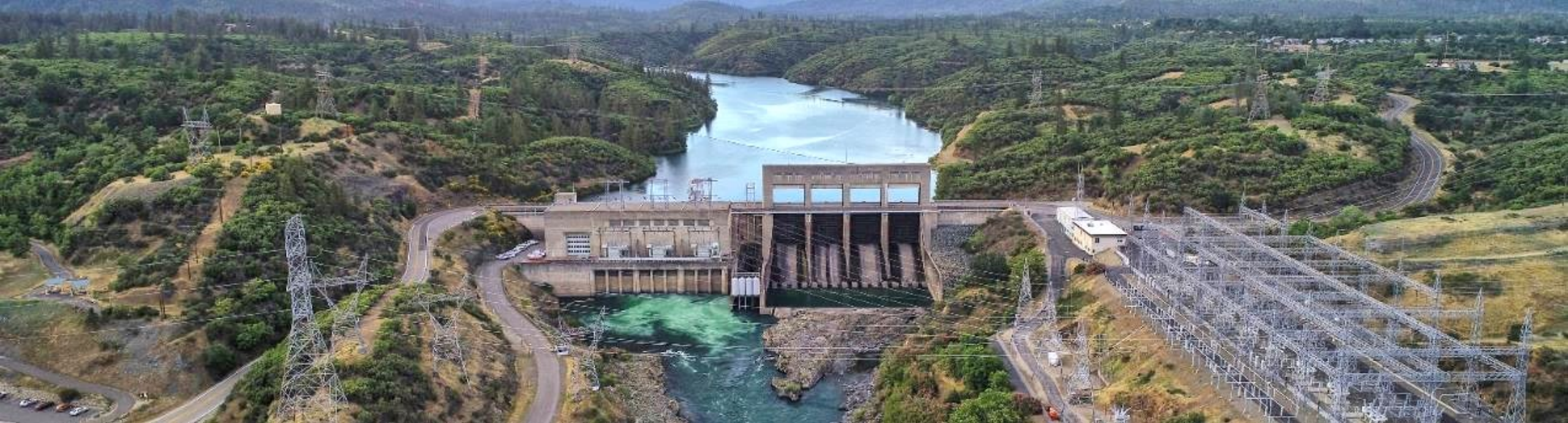
Keswick Dam, Sacramento River, Photo credit: John Hannon, Reclamation
