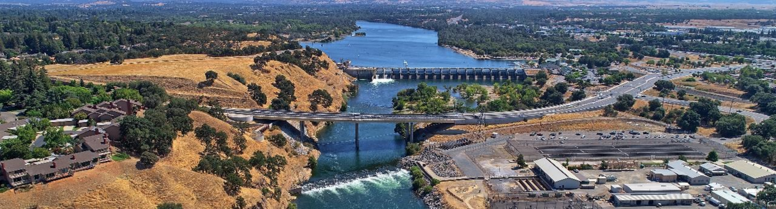
Nimbus Dam, American River, Photo credit: John Hannon, Reclamation
